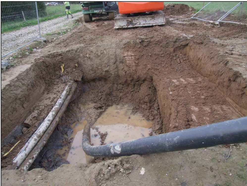
Plate 100: Typical Joint Bay excavation through previously examined horizons: example Joint Bay 2/3 within FRS151, view to N.
