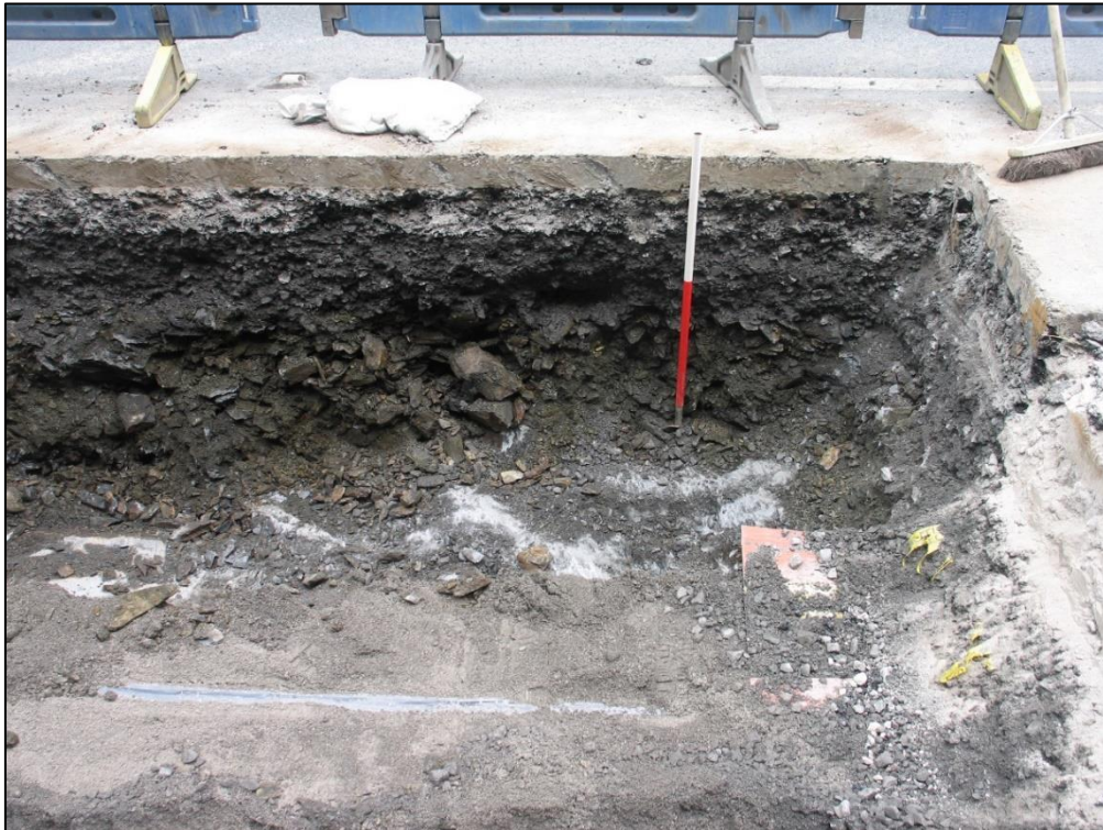
Plate 72: Excavated Joint Bay on line of A485 Road (location of ND186) showing modern road make-up (1m scale; 0.5m divisions), view to SE.
