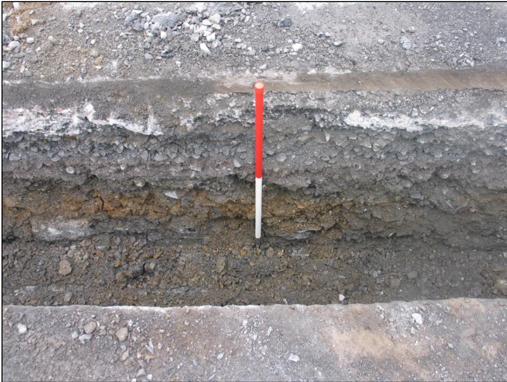
Plate 67: Trench cutting A485 Road (location of ND186) showing modern road make-up and redeposited shale contexts (074) – (077) (1m scale; 0.5m divisions), view to W.
