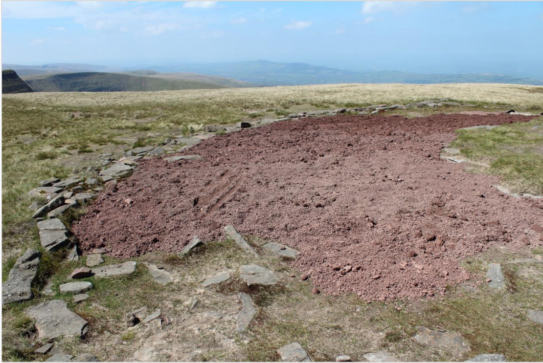
Photo 11: Fan Foel - showing the site after all the soil had been replaced within the eroded area. Looking roughly northeast.
