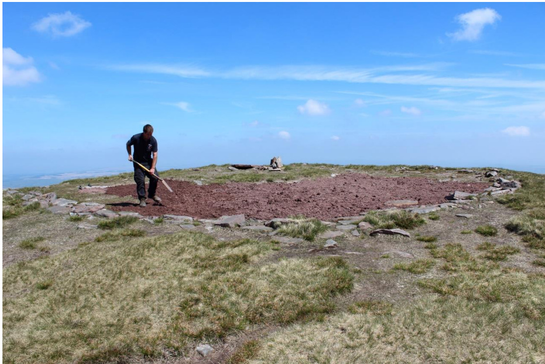
Photo 10: Fan Foel - showing a BBNP warden replacing the soil within the eroded area defined by the stone kerb. Looking roughly east.
