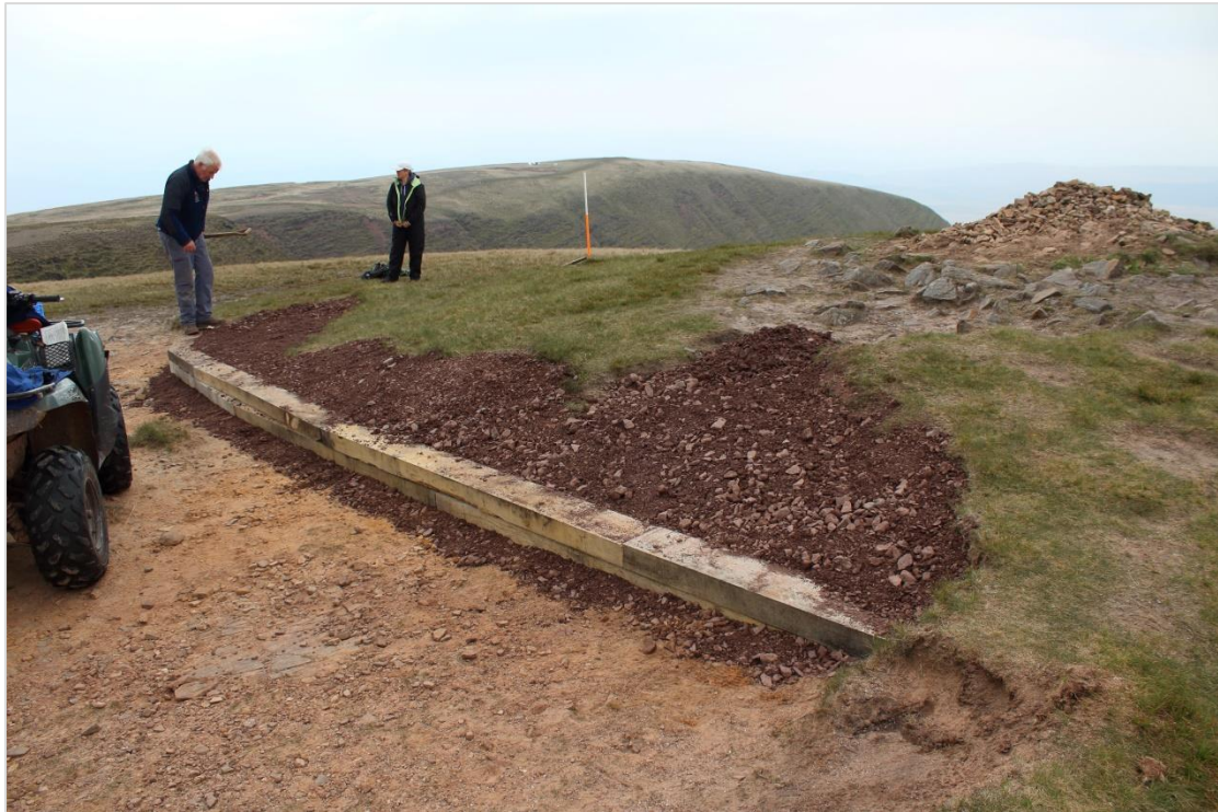
Photo 18: Twr y Fan Foel – the completed soil packed into the gap against the wooden revetment. Looking roughly north.
