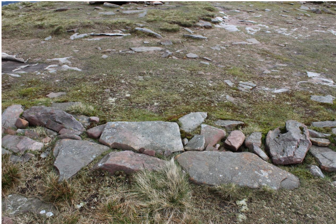
Photo 6: Fan Foel - showing detail of the exposed stone kerb and evidence of exposed geotextile. Looking roughly east.
