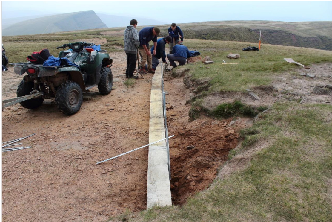
Photo 16: Twr y Fan Foel – building a wooden revetment to the southern side of the burial cairn. Looking roughly west.
