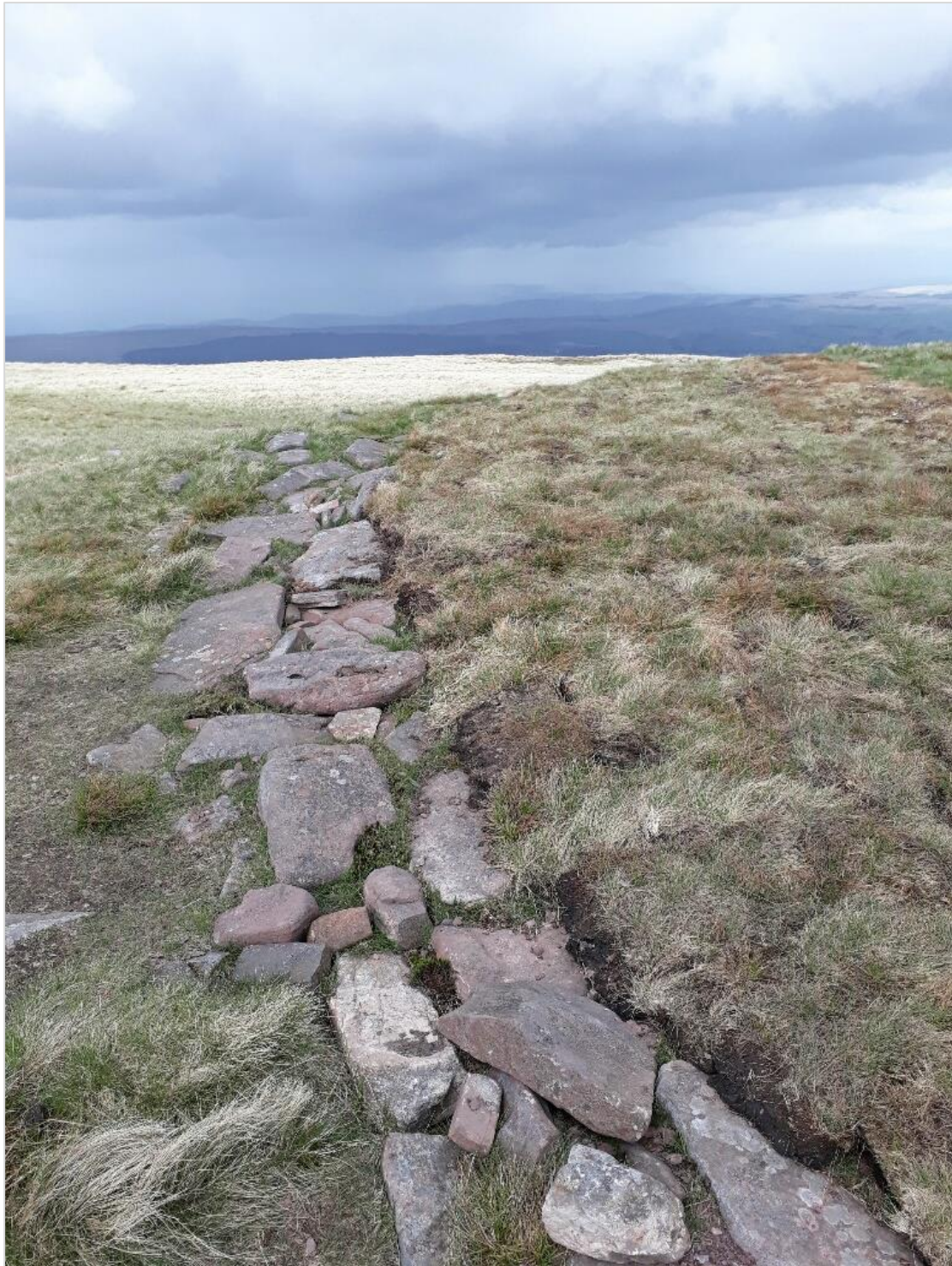
Photo 15: Fan Foel - showing detail of the exposed stone kerb after the eroded area had been re-turfed. Looking roughly north.
