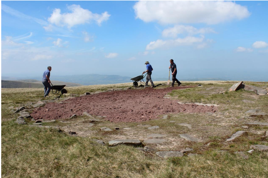
Photo 9: Fan Foel - showing the BBNP wardens replacing the soil within the eroded area defined by the stone kerb.. Looking roughly northeast.
