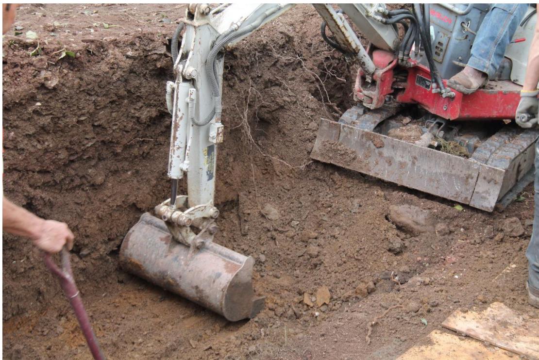
Photo 4: Looking northeast at the excavated foundation trench for the wall rebuild under excavation, at its deepest, showing brownish orange natural
