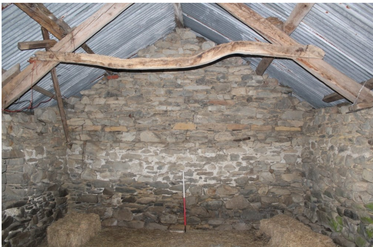
Figure 6. The interior of the farm building (north gable) showing selective areas of lime pointing.
