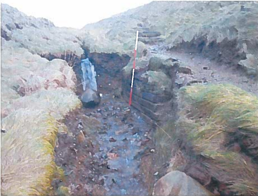
Porth y Rhaw: retaining wall as rebuilt but being undercut. Footpath above left to be cut further back into natural bank. Scale 2m. View E. 16/01/2014
