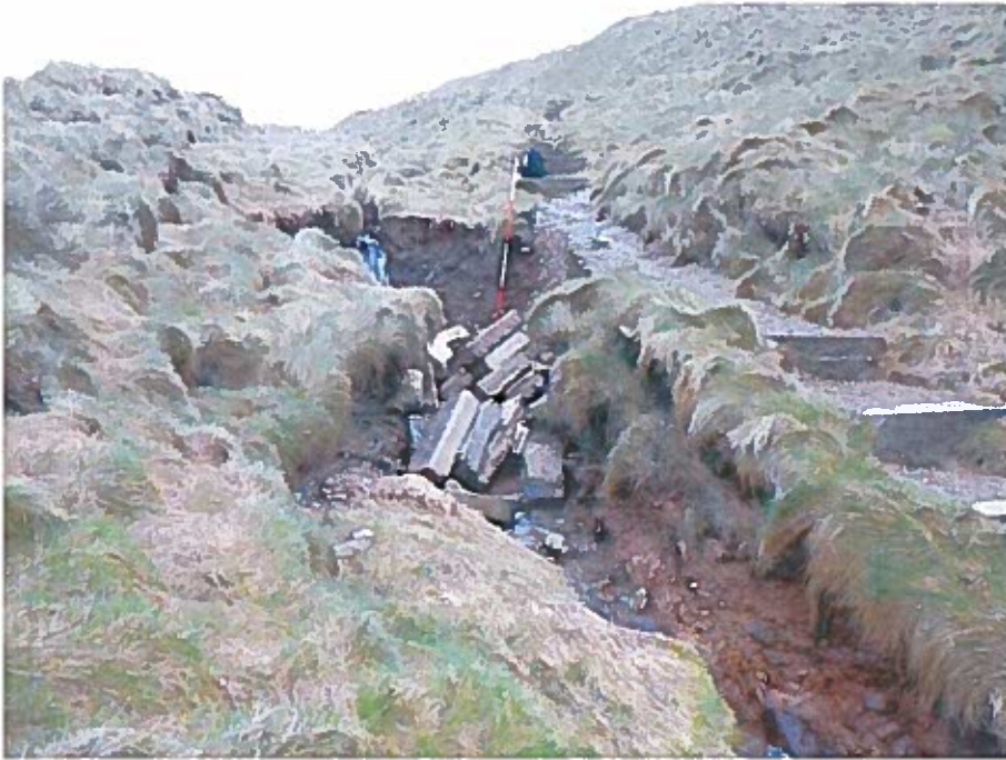
Porth y Rhaw: water damage to retaining wall. Scale 2m. View E. 12/02/2012
