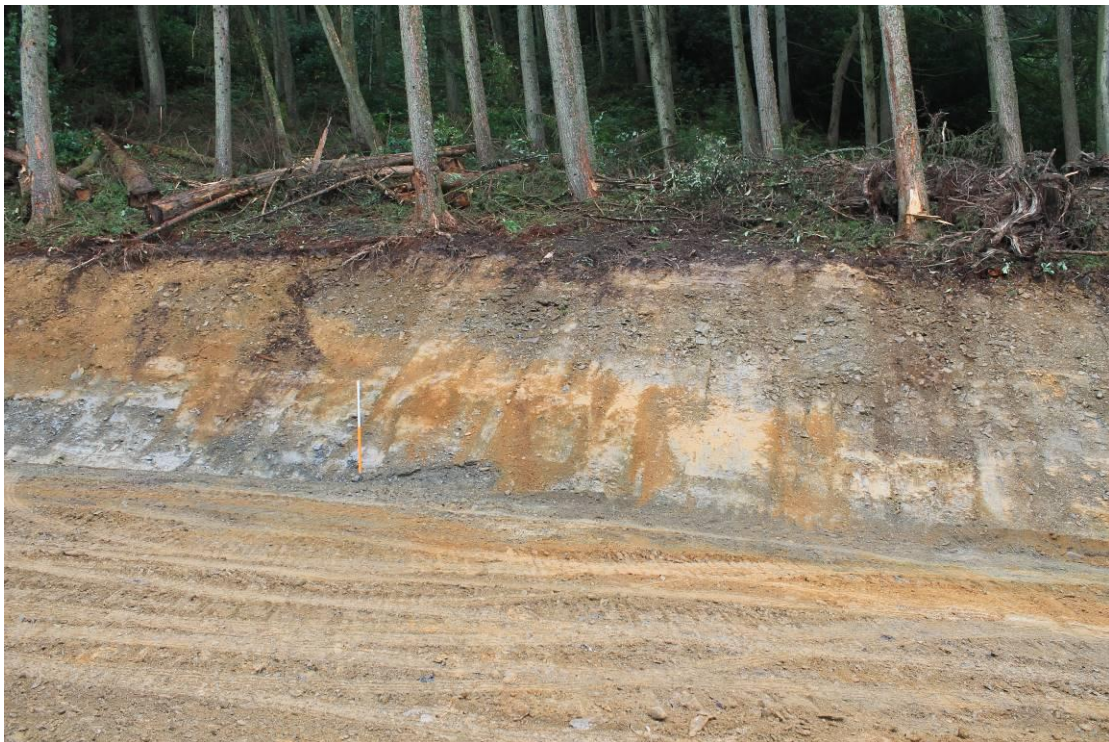
Photo 3: Representative section of access road showing topsoil and underlying sands and silts.
