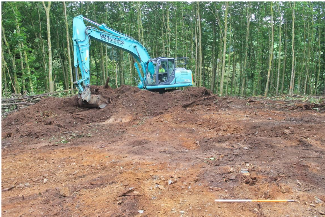
Photo 1: Mechanical excavator removing the topsoil and exposing the underlying silts and sand.
