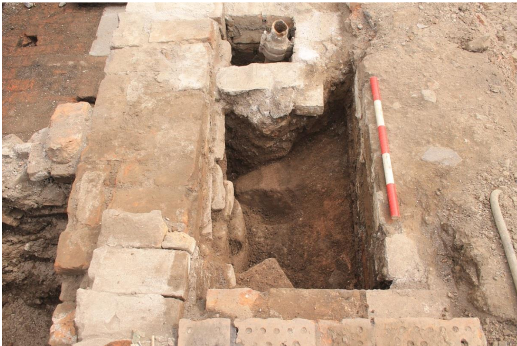
Photo 28: Gap between the furnace room section of wall [1] and wall [2], with hot water pipe and brick surround. View east; 0.5m scale
