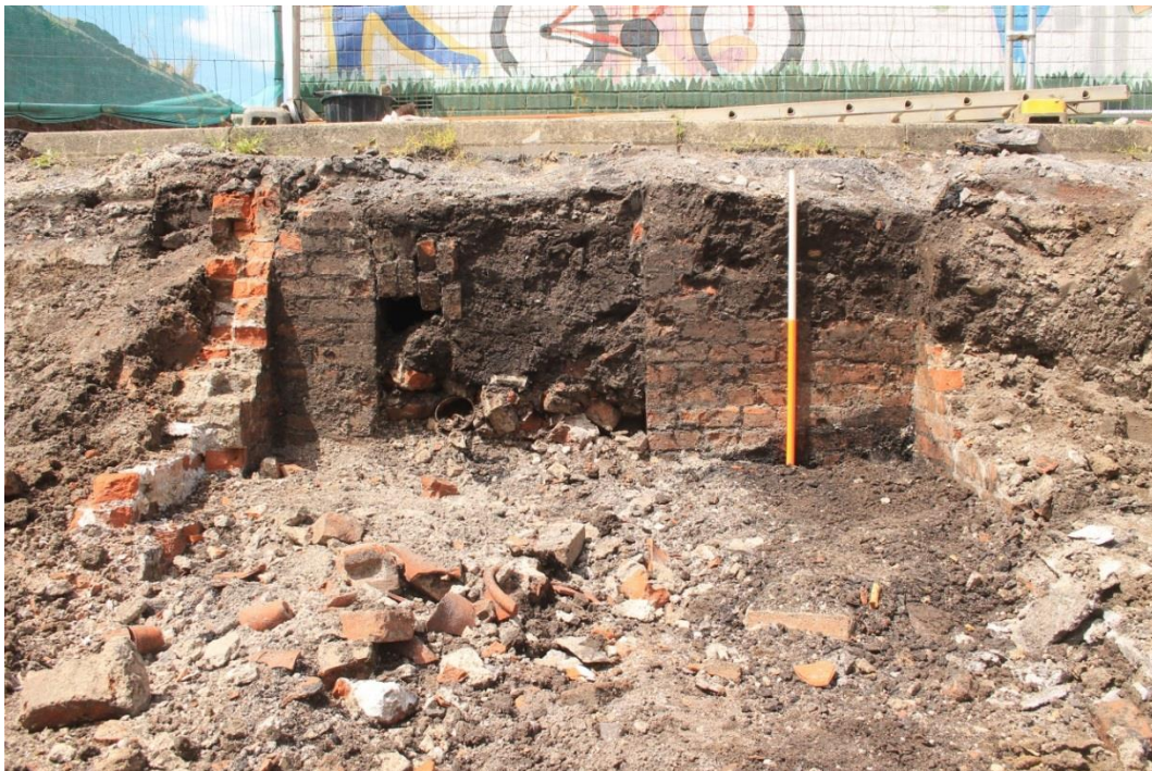
Photo 30: North wall of furnace room with possible collapsed arch. View north; 1m scale.
