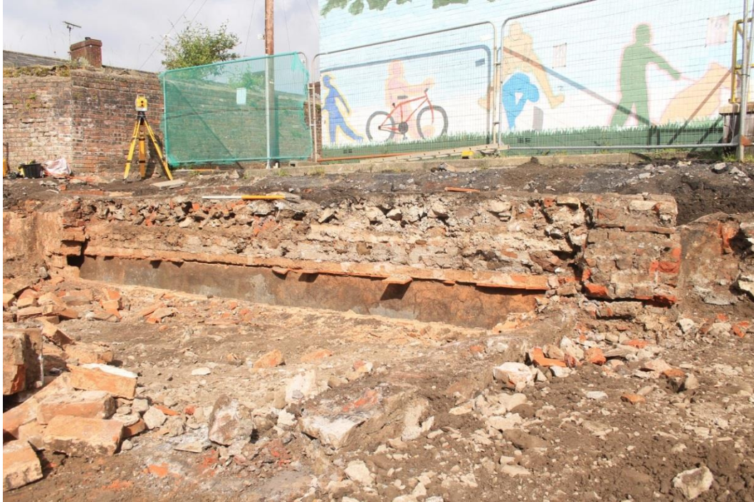
Photo 7: Flue [6] exposed within wall [2]. View NW; 1m scale
