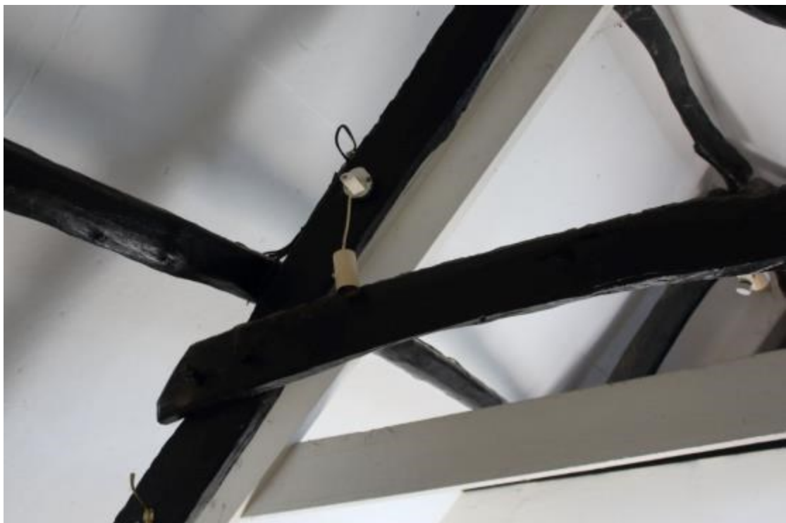
Photo 9: Both original and modern timber A-frames can be seen in the loft of the 18 th century building.
