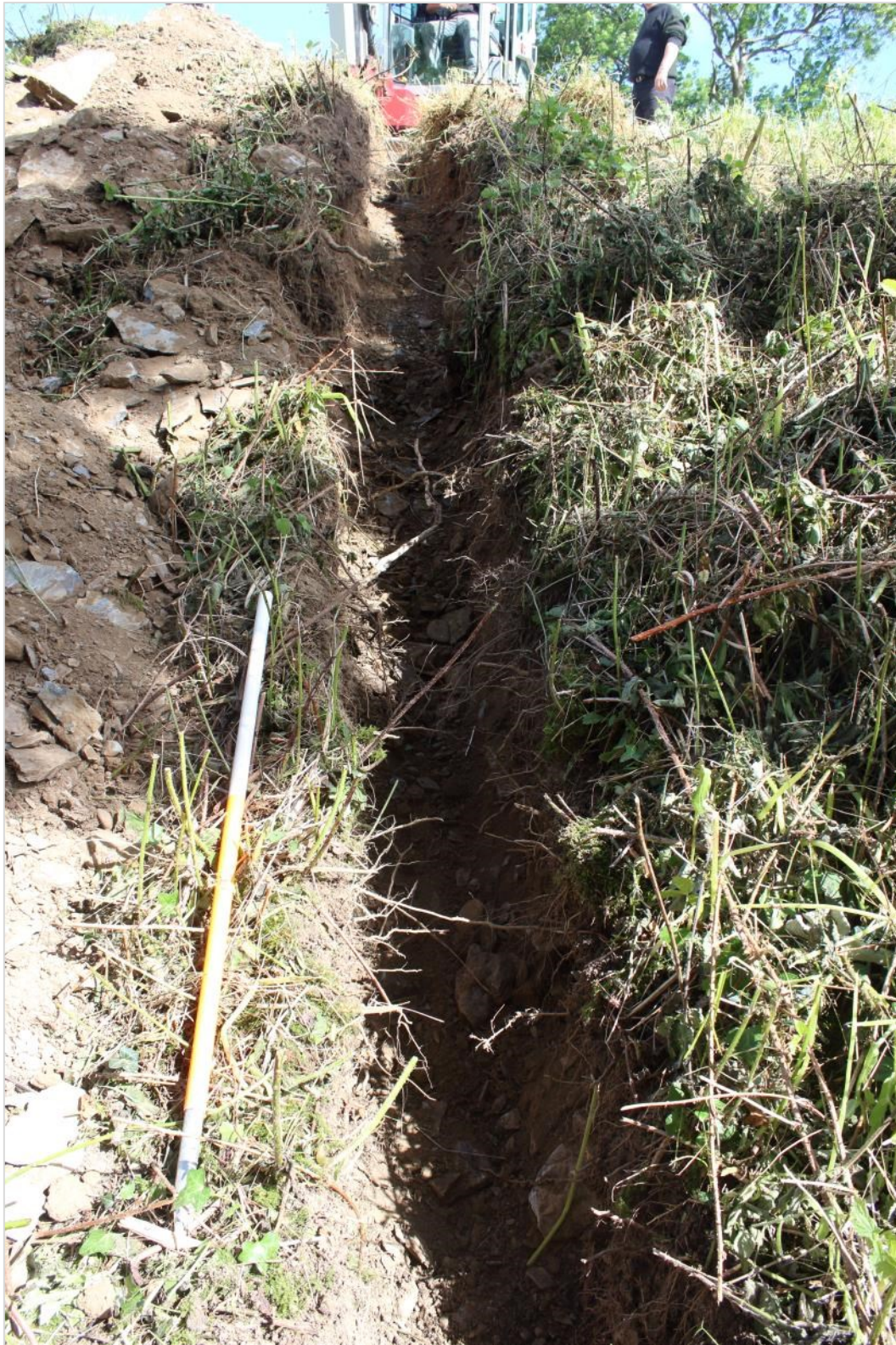
Photo 8: The fully excavated cable trench [B]. Note the number of large flat stones disturbed by the trench towards the top of the earthen bank. Facing north; 1m scale
