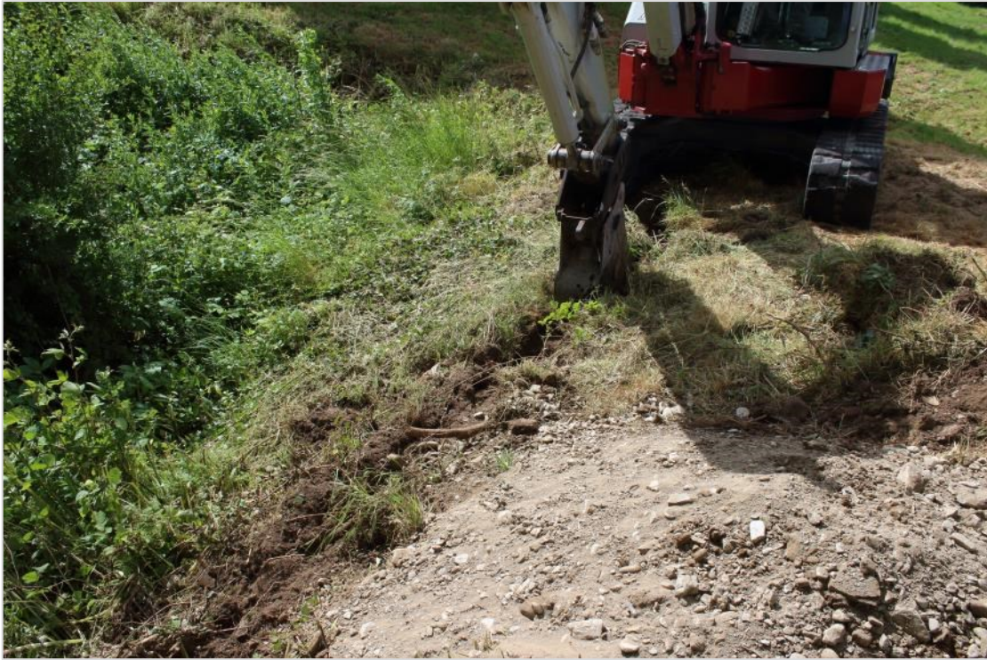
Photo 6: Excavating cable trench [A]. Facing south
