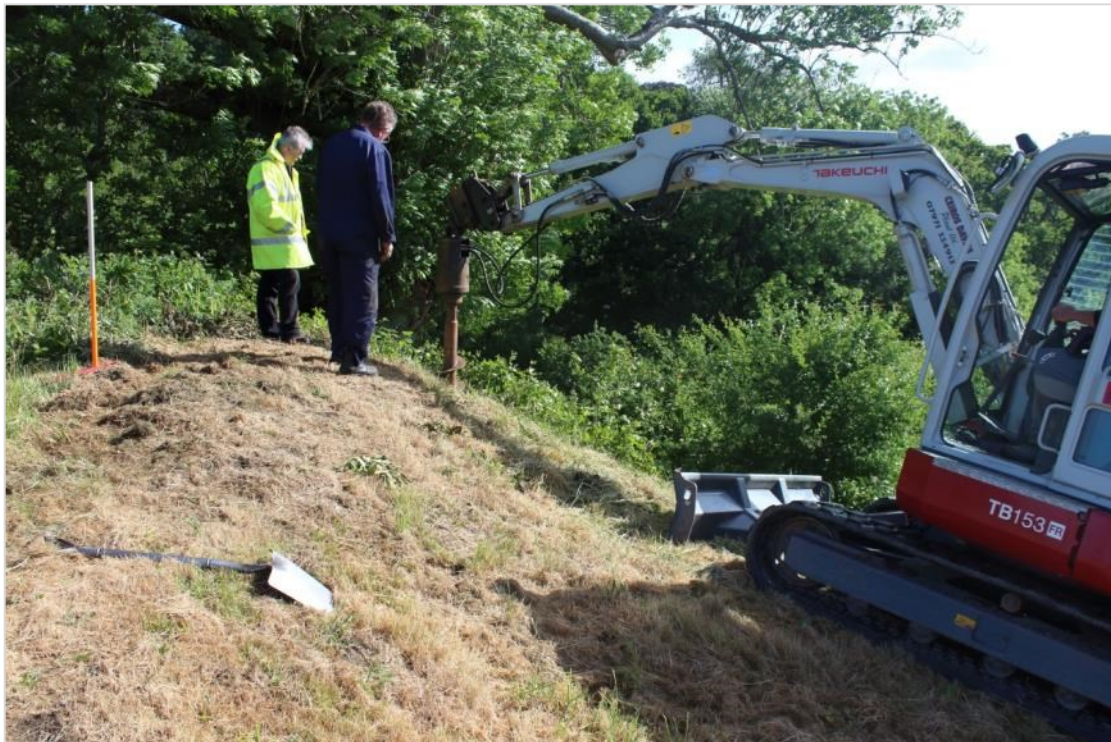
Photo 2: Machine excavation of hole [A]. 1m scale
