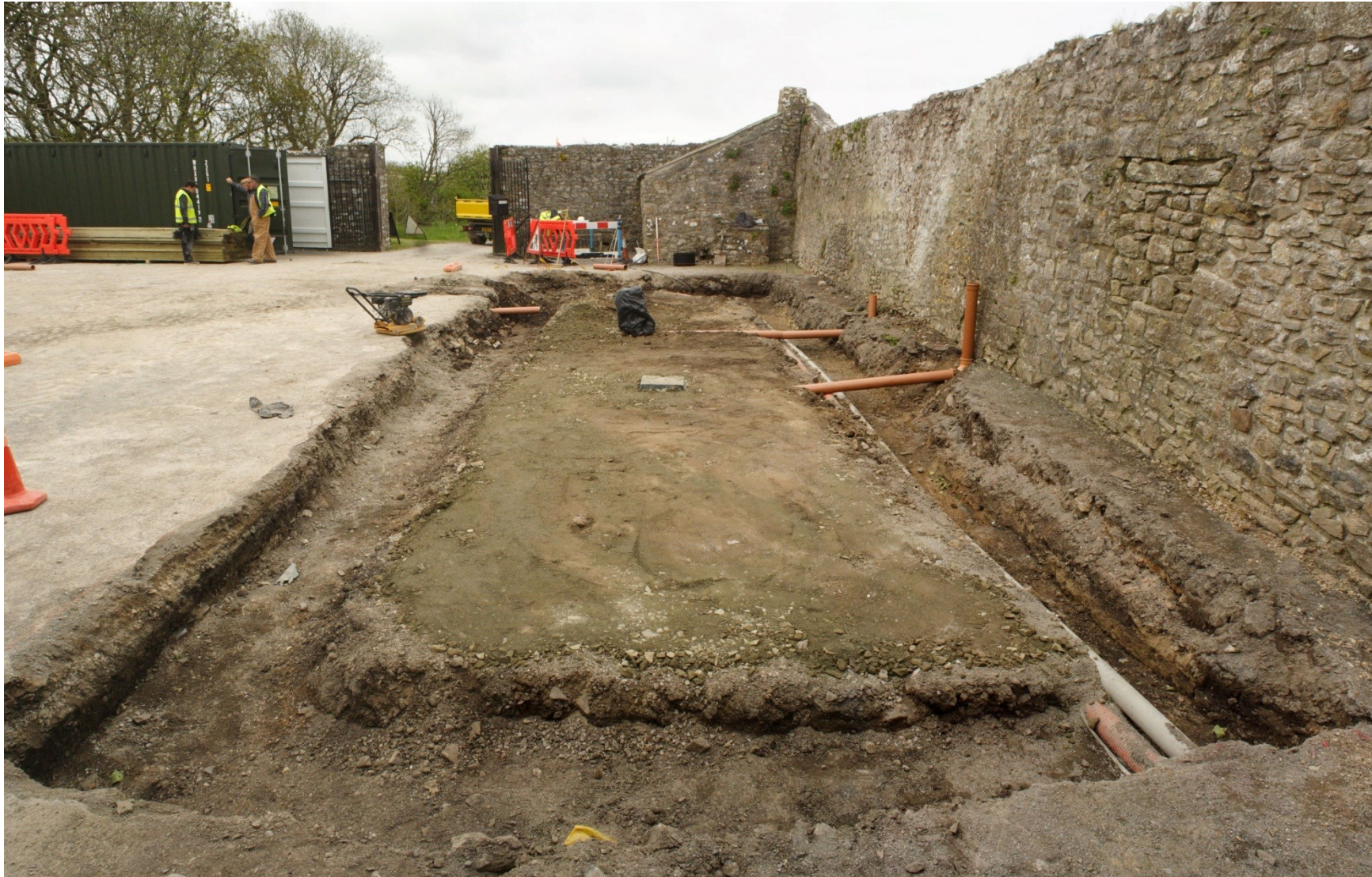
Photo 18: View east across the completed footprint for the new café building raft foundation, including radon mitigation system, service ducting and levelled material over central part of footprint
