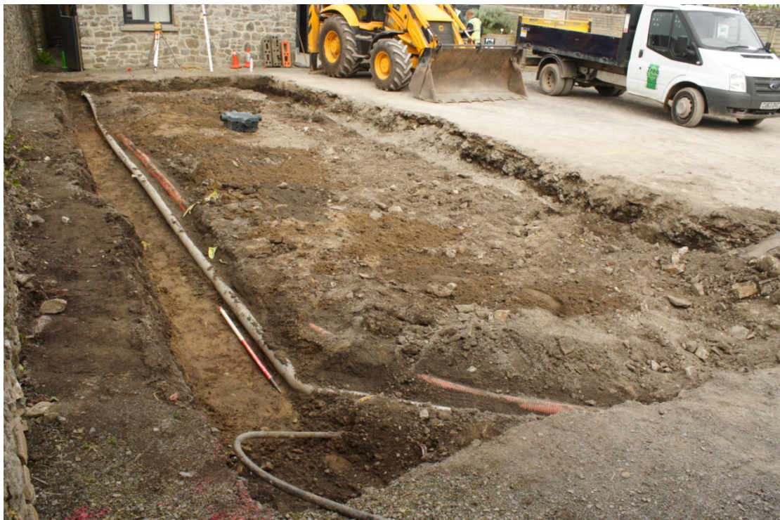
Photo 17: View northwest across café footprint following site strip and excavation of perimeter 'toe' trenches, prior to radon gas mitigation and service duct installation.
