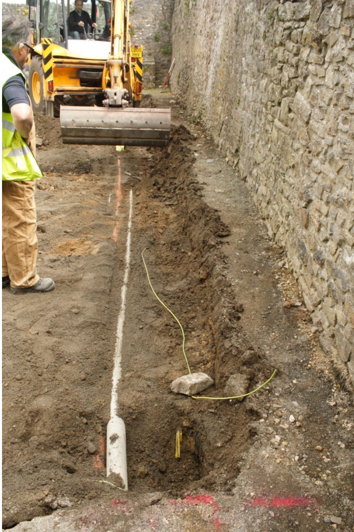
Photo 11: Southern edge of café footprint showing exposure of orange and grey service ducting and redundant earthing cable, viewing east
