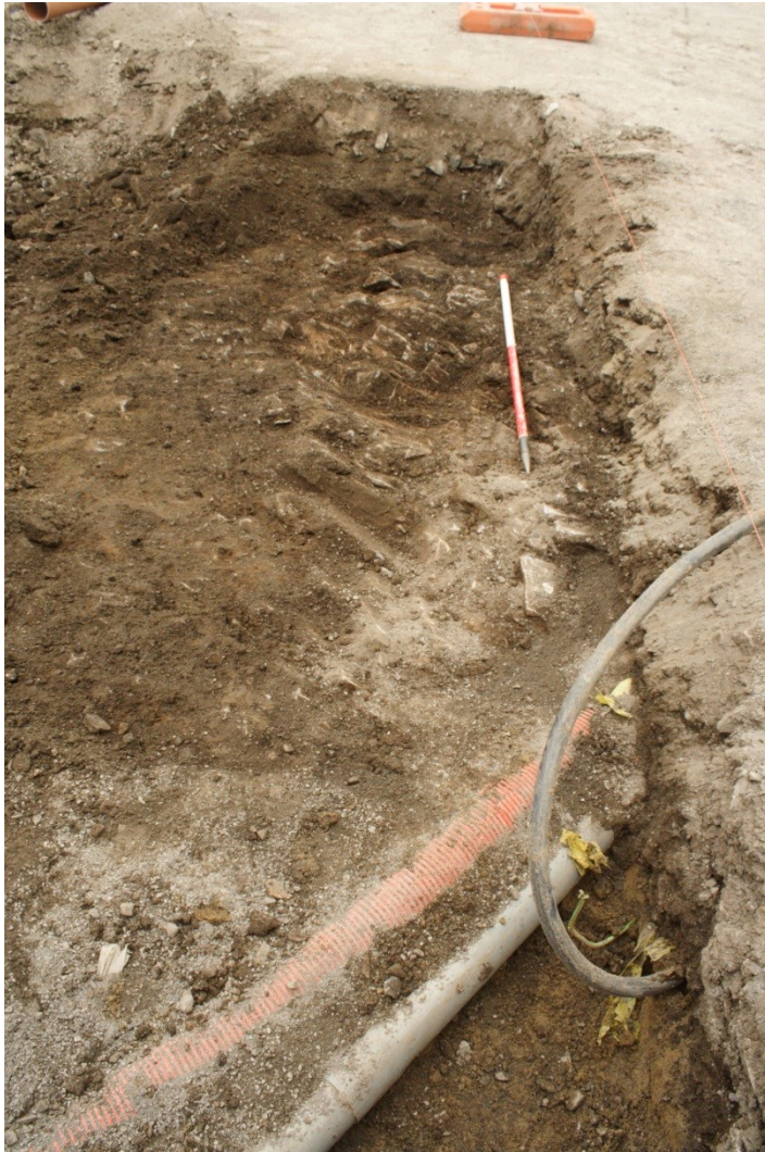
Photo 15: View north along eastern end of café footprint showing bedrock exposed along 'toe' trench and edge of rock-cut ditch with service ducts in foreground
