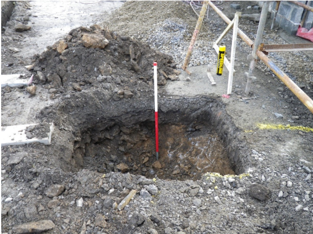
Photo 7: View east across western rectangular trench showing bedrock and mixed dark soil and rubble layer above
