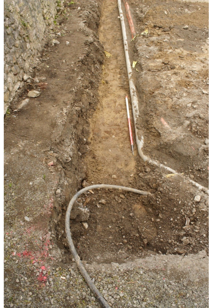
Photo 12: View west along orange and grey service ducting following removal of 'toe' with sand exposed beneath, and with redundant electricity cable visible
