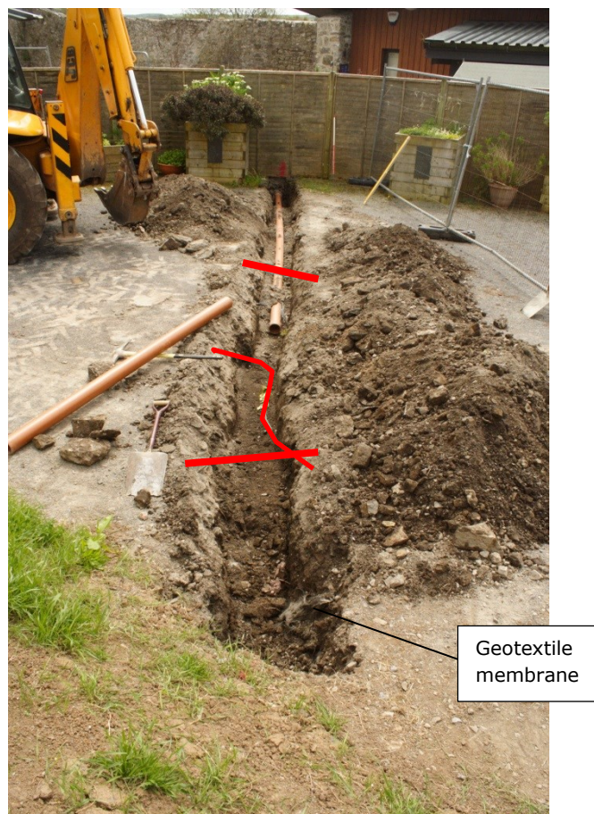
Photo 20: Electricity cabling recorded crossing the line of service Trench B (highlighted in red) viewing southeast. (Note the geotextile material in foreground associated with existing soakaway)
