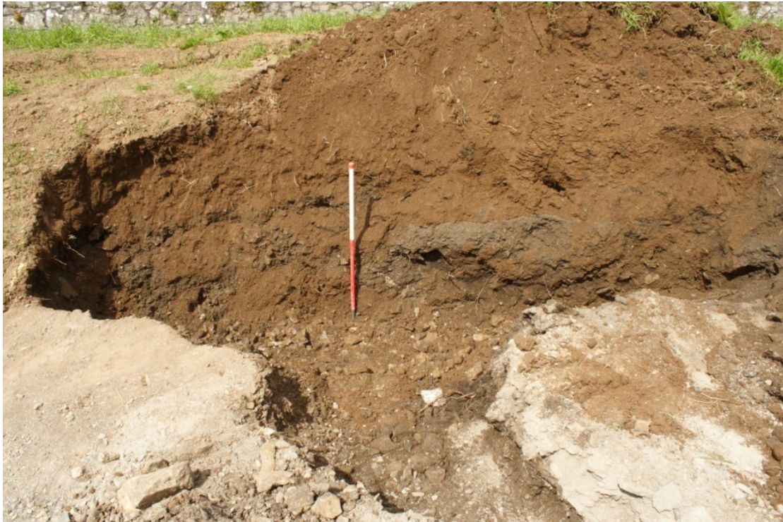
Photo 22: View northwest showing soakaway dug at the northwest end of service Trench B, with clean bedrock exposed at base.
