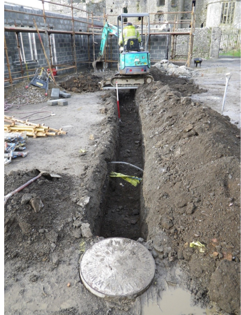
Photo 6: View west along drainage trench from existing manhole towards toilet block, with existing electricity cables visible crossing the trench (2013)
