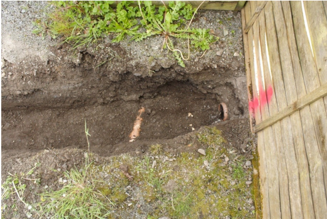
Photo 19: Plastic drain pipe exposed at the base of the service Trench B at the fence line, installed and observed in 2013, viewing east.
