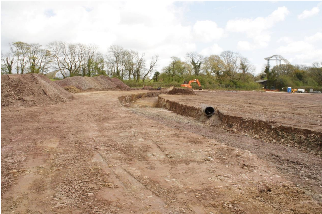
Photo 11: View east across the northern part of the Sky Dome footprint, showing the remains of the former diverted drainage pipe
