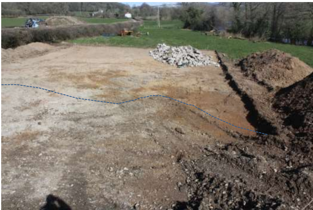
Photo 6: View northeast across site area showing change from former silage clamp area and stone in foreground to natural sands and gravels beyond (blue line)
