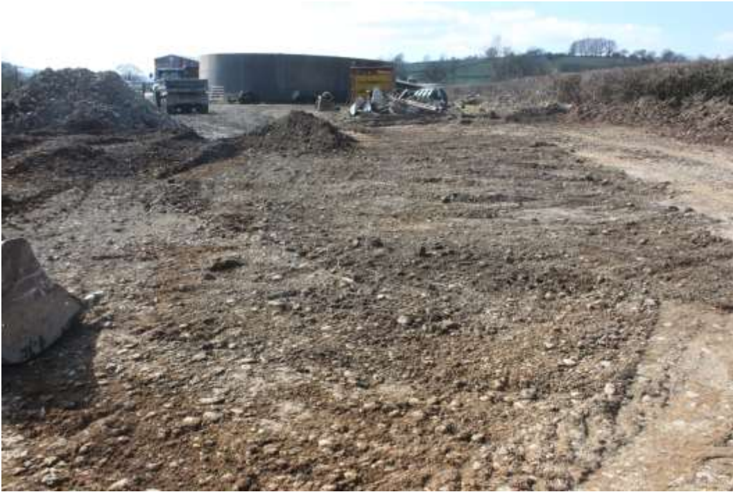
Photo 3: View southwest across western side of site area showing thin topsoil and remnants of stone levelling layer for former silage clamp
