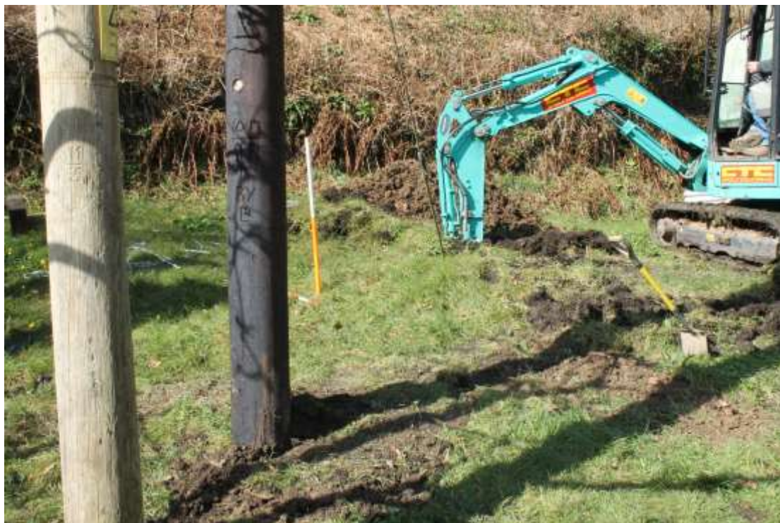
Photo 6: Looking west-northwest at excavation of the trench for the anchor stay at Pole 6
