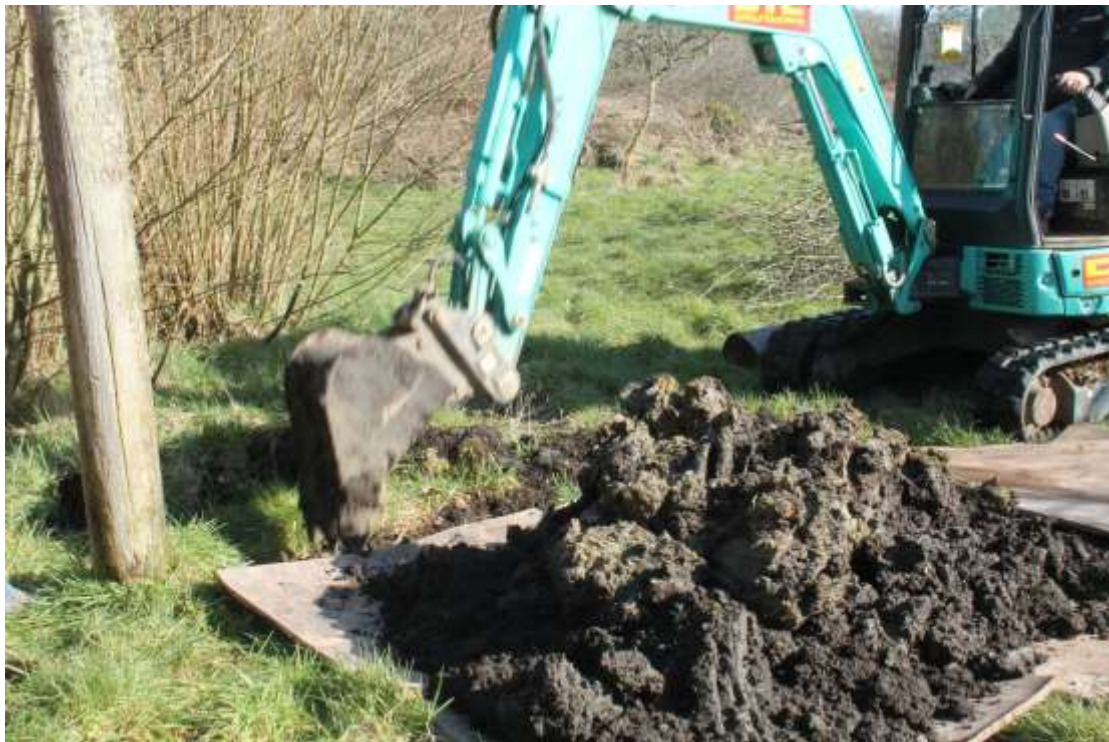
Photo 1: Looking north-northeast at excavation of the trench for replacement Pole 5
