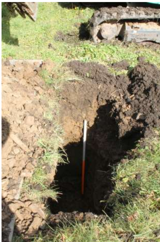
Photo 7: Looking west-southwest at the trench for the new anchor stay for Pole 6, with a 1m scale
