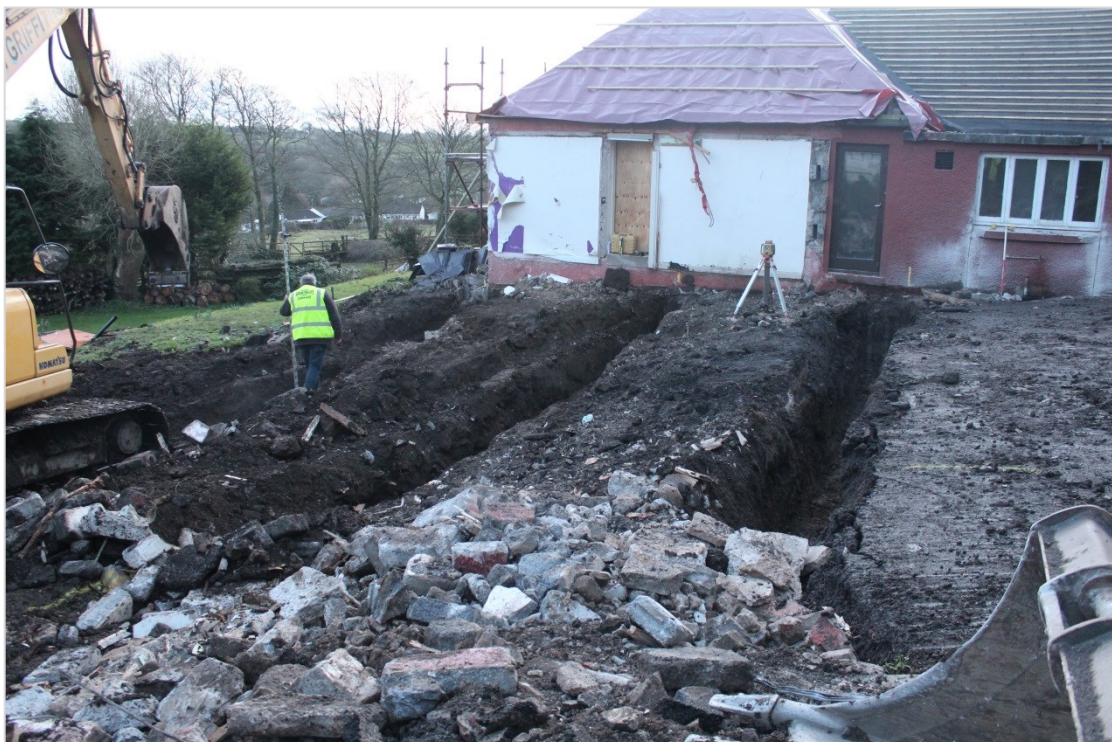
Photo 7: View roughly west-southwest across the footprint of the proposed extension following the excavation of the three foundation trenches.
