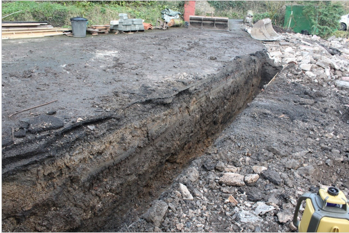
Photo 6: Northern foundation trench excavated along the length of the extension showing layers of redeposited material above natural subsoils.
