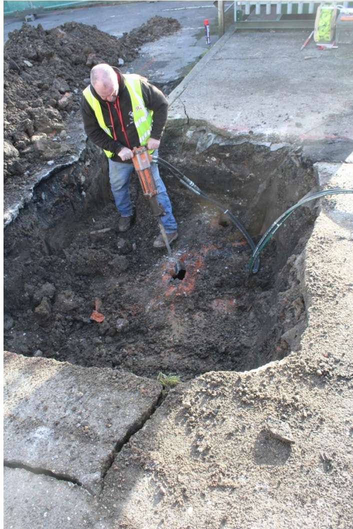
Photo 14: Drilling into the top of the vault within the extended trench area
