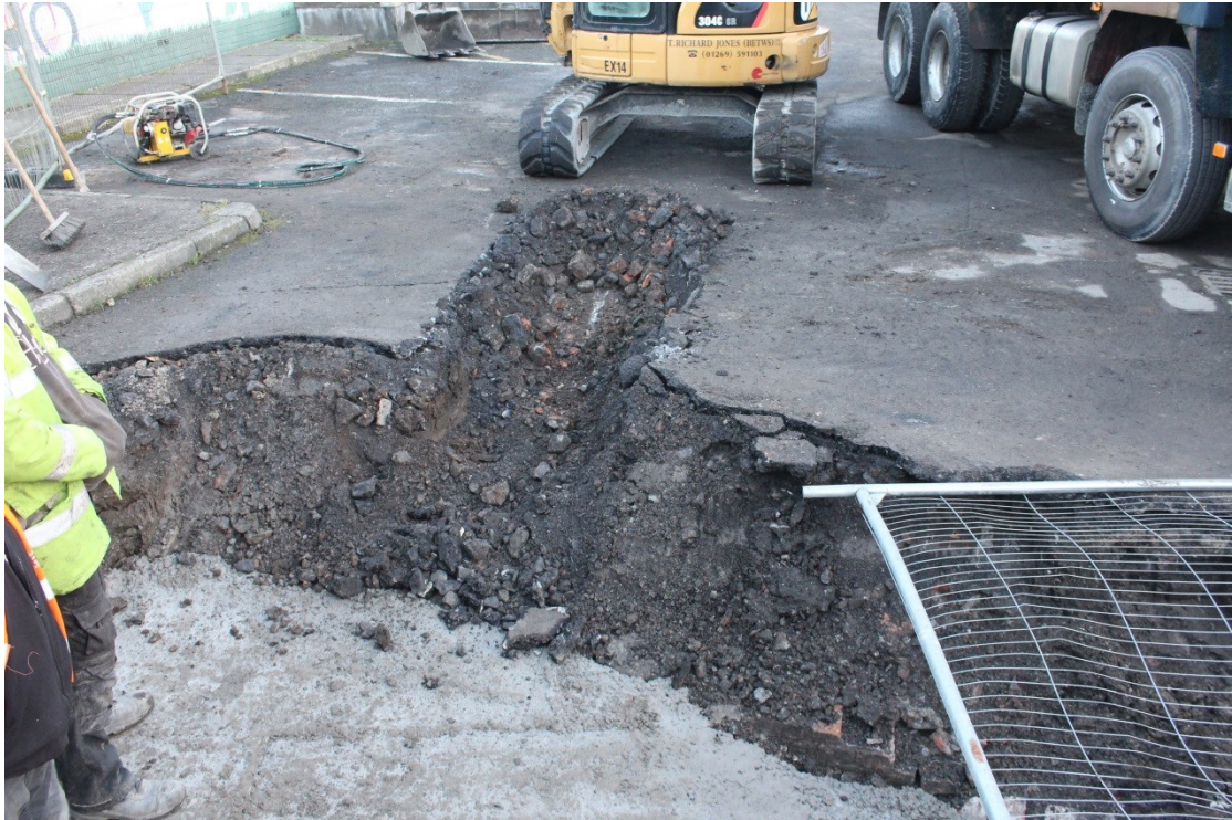
Photo 22: Excavation of trench to the east of the archway, showing concrete backfill of northwestern chamber
