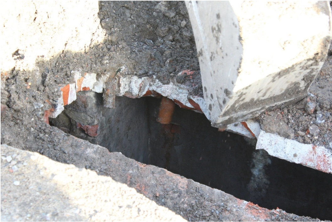
Photo 15: Machine breaking into the vault
