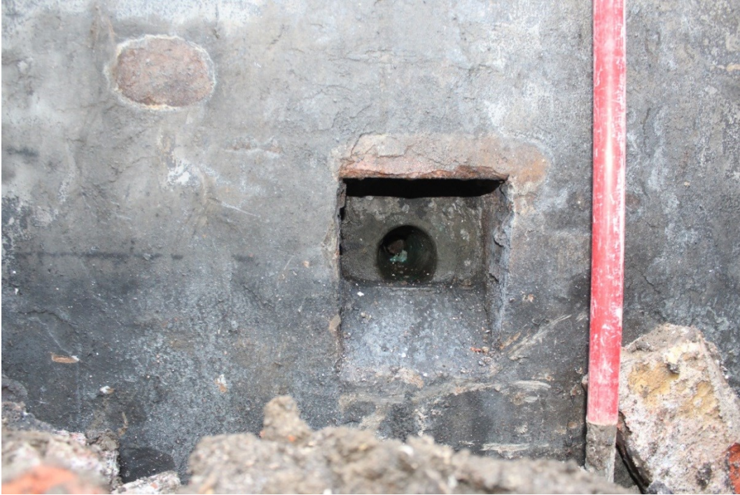
Photo 18: detail of pipe leading through wall between the two chambers
