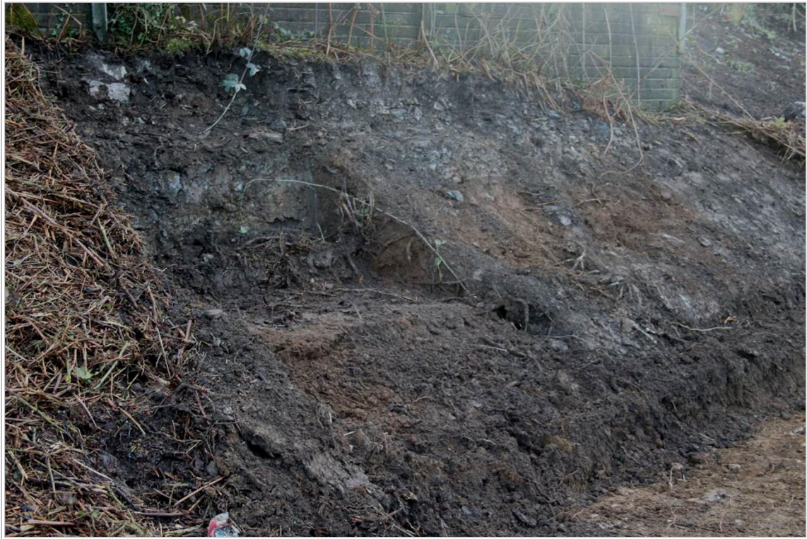
Photo 6: Looking south-southwest at stepped-slot excavated through made-up ground embankment just north of Co-op store.
