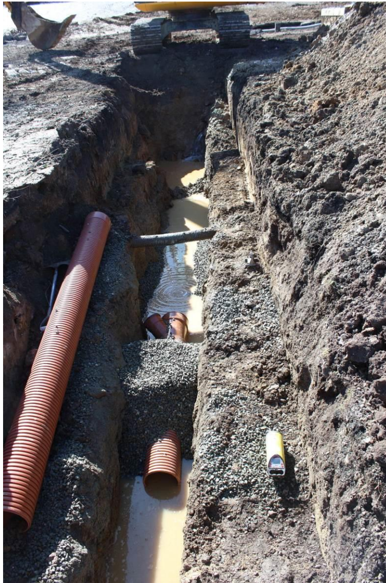
Photo 19: Looking southwest along the excavated trench during insertion of new pipes, with previous services crossing the trench.
