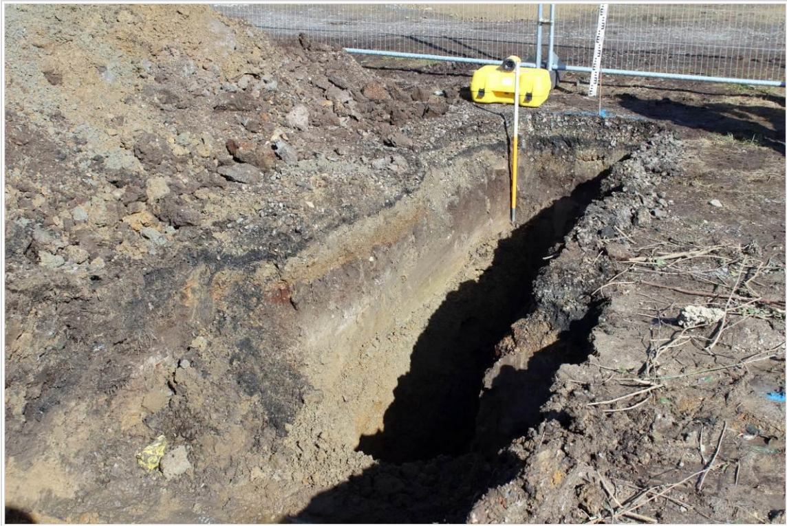
Photo 17: Looking north at north end of trench after excavation showing in section the layers of made-up ground, with 1m scale
