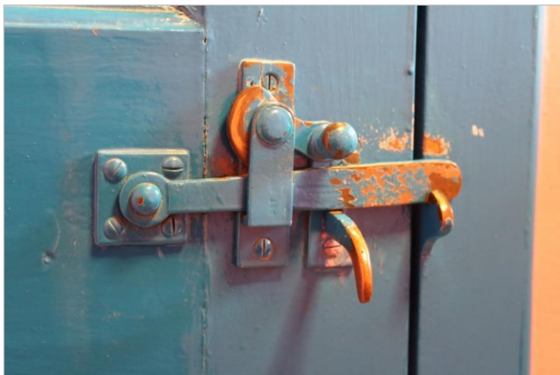
Photo 29: Latch mechanism for toilet door.
