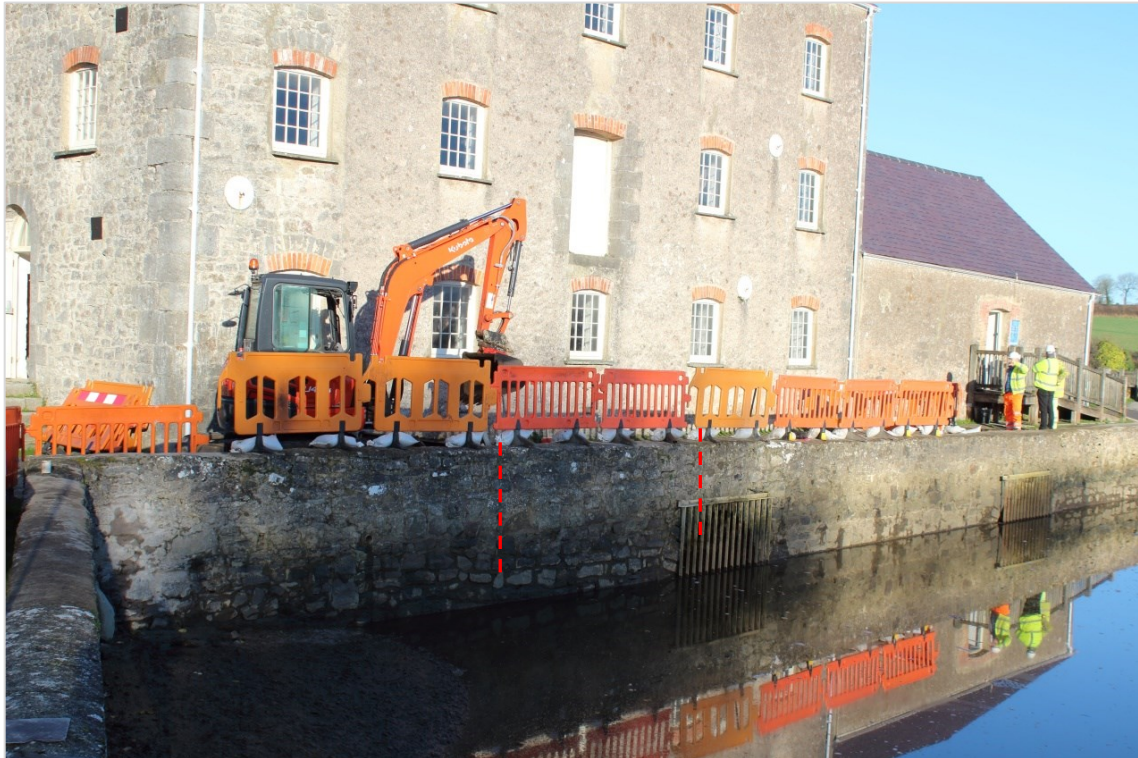
Photo 1: Illustrating the location of the inspection trench over the sluice leading to the south mill wheel (red dashed lines mark approximate location of inspection trench).
