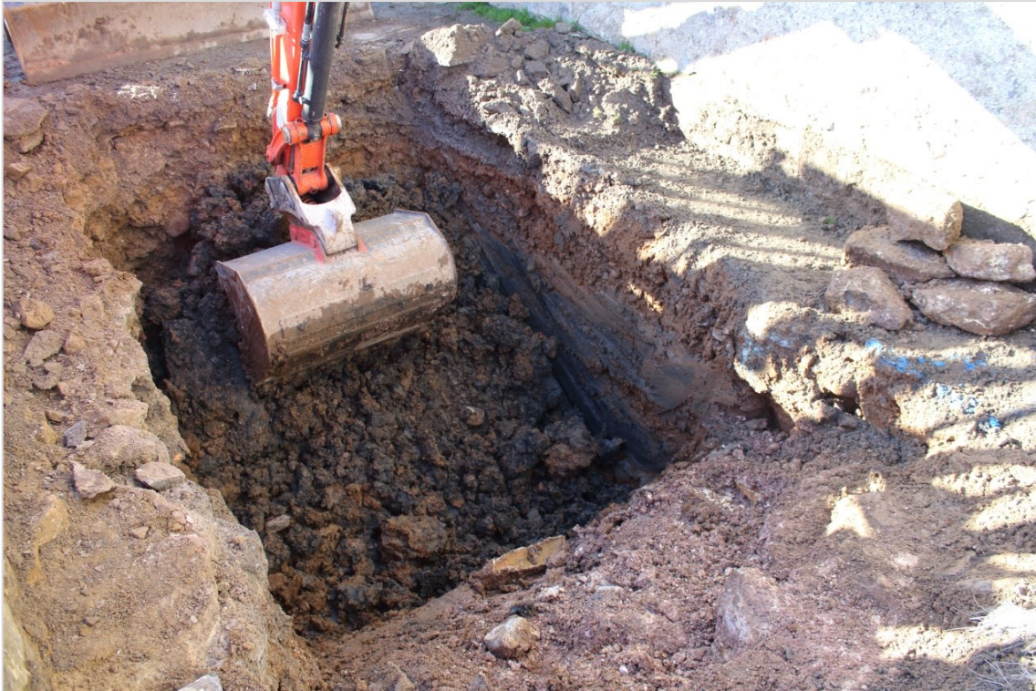
Photo 2: The stratigraphic sequence observed in the southeast facing section of the inspection trench.
