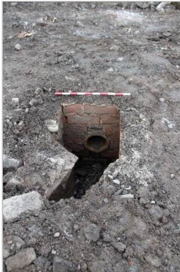
Photo 15: View north: brick inspection chamber of drain. 1m scale
