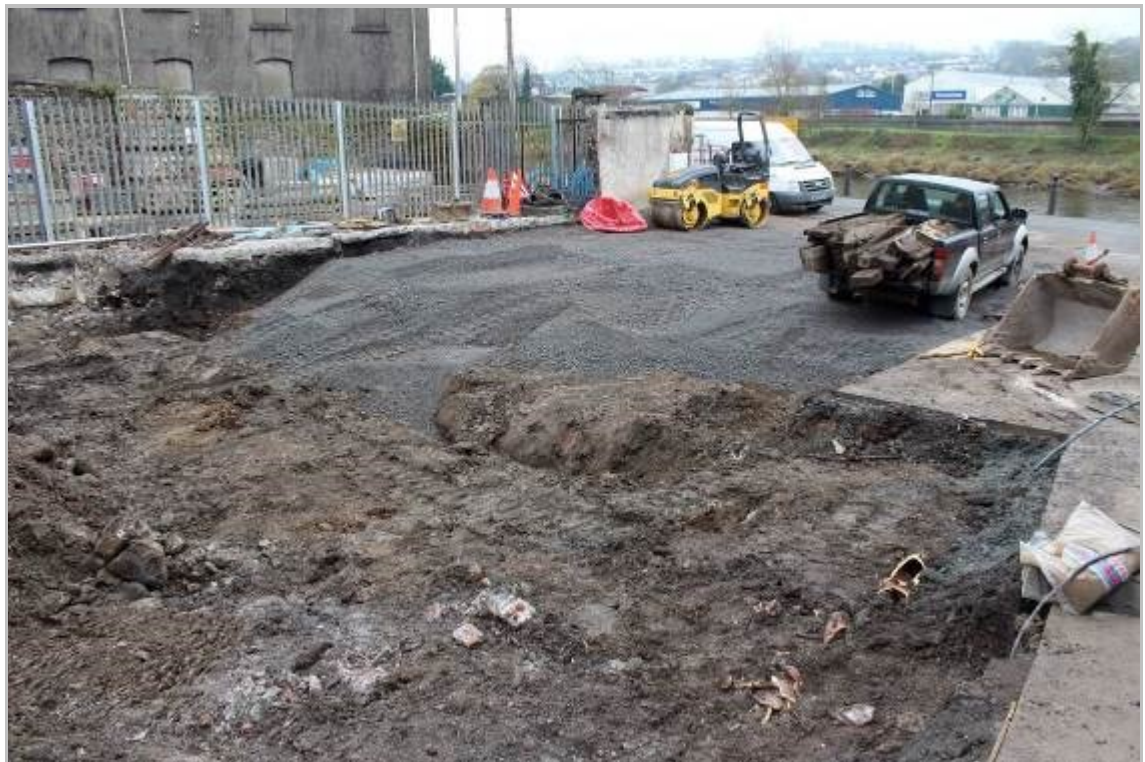
Photo 17: View southeast; clean stone in the process of being spread over site prior to piling.
