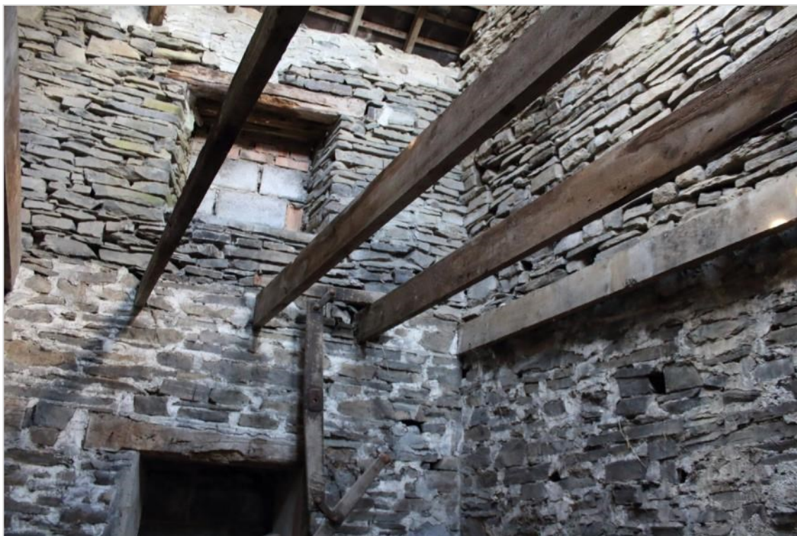
Photo 13: Internal shot showing blocked upper north window and wooden joists.
