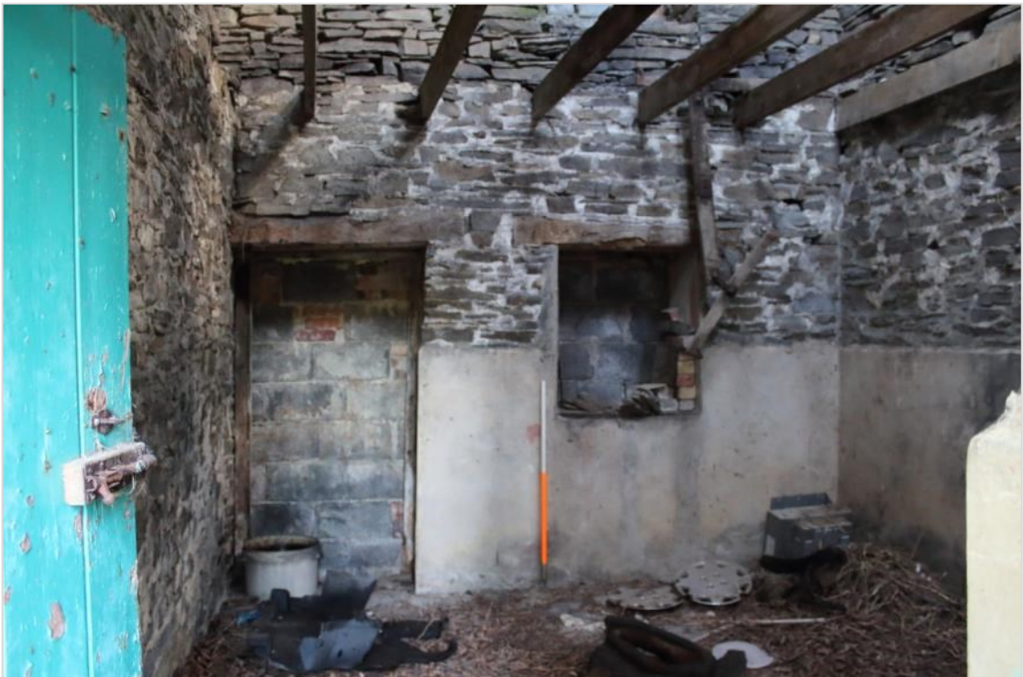
Photo 10: Internal shot showing blocked front door and ground floor north window. 1m scale
