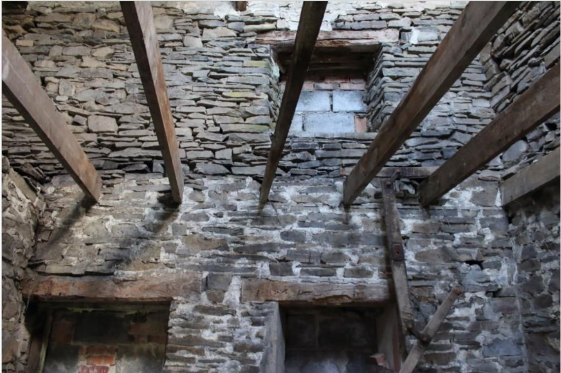
Photo 11: Internal shot showing blocked front door and ground and 1 st floor north windows and wooden joists.
