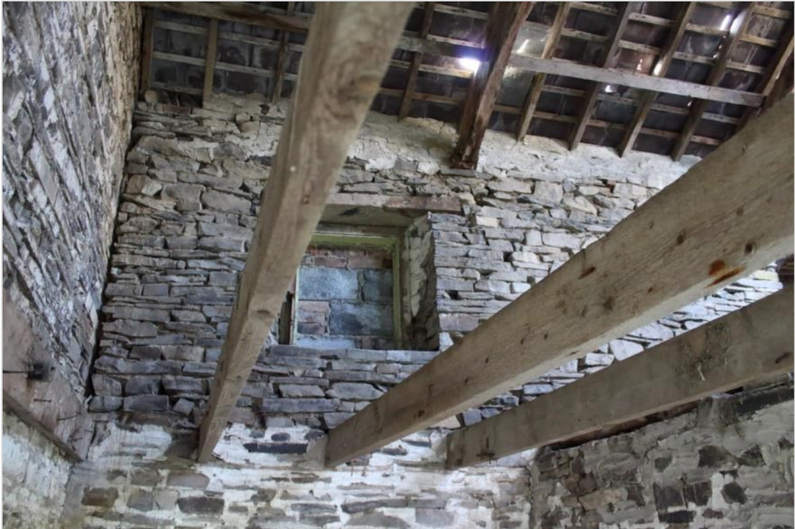
Photo 7: Detail of blocked 1 st floor south window.
