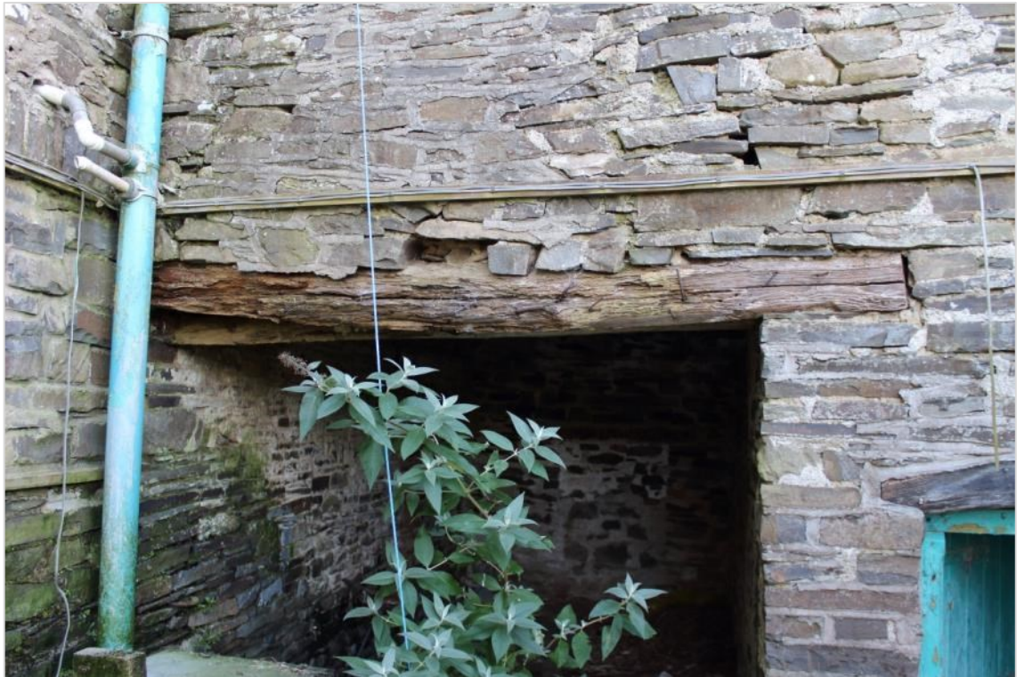
Photo 5: Detail of wooden lintel inserted into outer wall.
