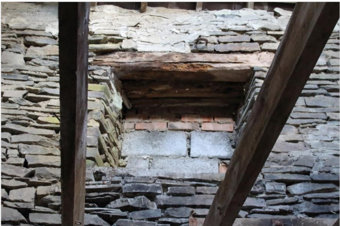
Photo 12: Detail of blocked 1 st floor north window.
