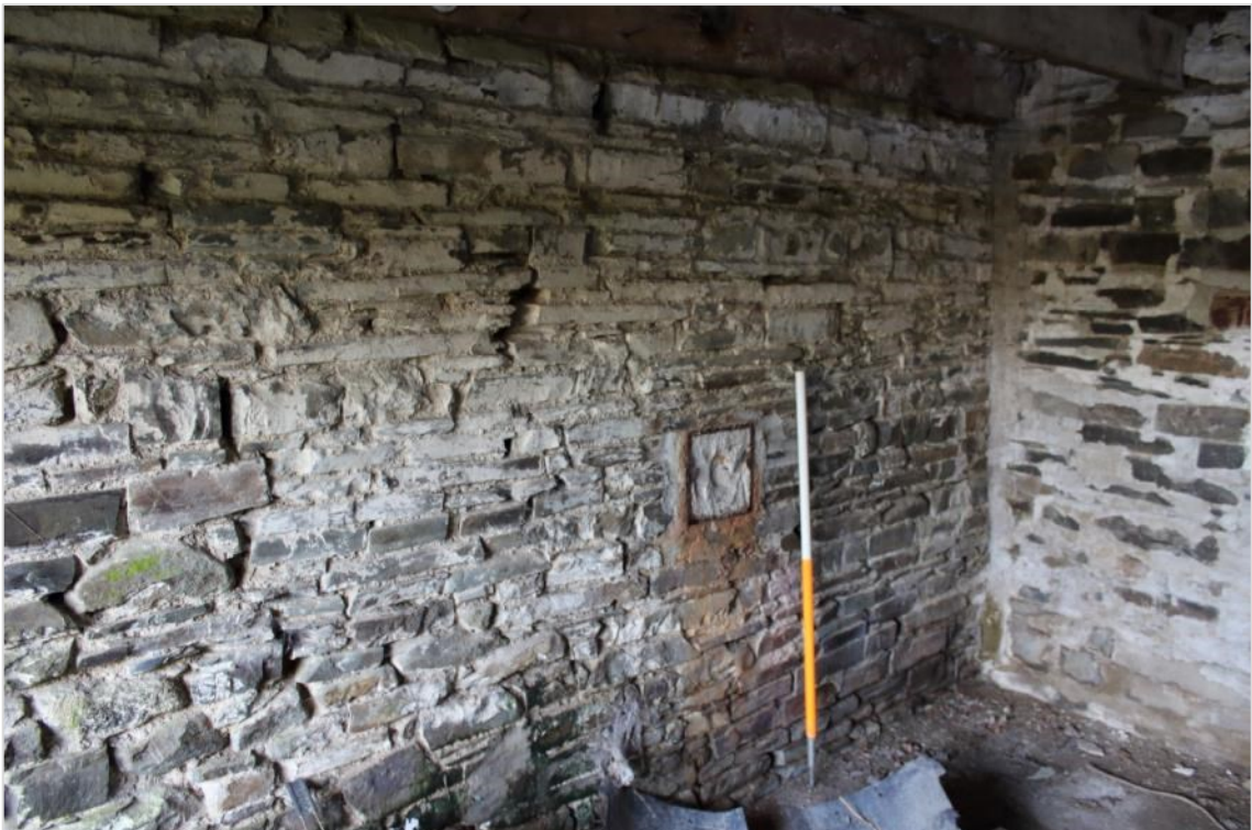
Photo 8: Detail of blocked heating vent(?) within southern party wall with Commercial Inn property. 1m scale
