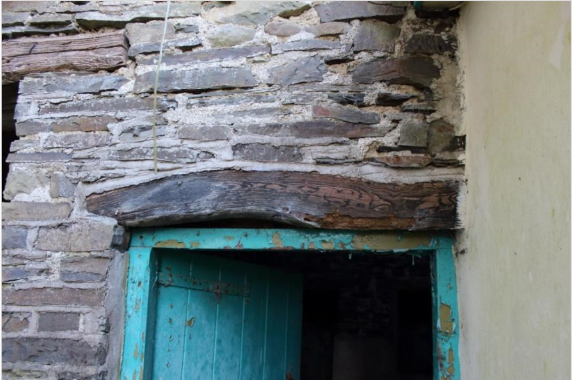
Photo 9: Detail of wooden lintel beam above rear door.
