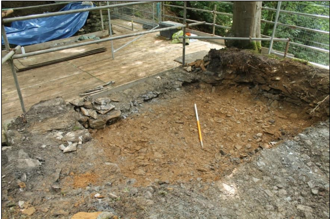
Photo 19: An overview of the final extent of excavations in the fill of the north-western abutment (DAT Photo 110511_0049).
