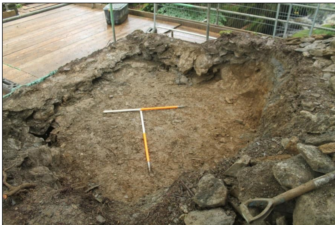
Photo 10: An overview of the final extent of the excavations in the south-eastern abutment showing the partially dismantled western and northern walls of the abutment (DAT Photo 110511_0030)
