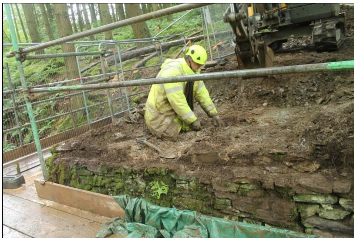
Photo 6: The insert for the bearing beam on the western face of the south-eastern abutment. The height of this wall was reduced by hand (DAT Photo 110511_0014).
