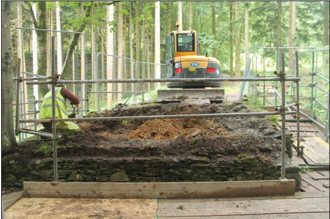
Photo 15: The bearing beam inset revealed on the eastern wall of the north-western abutment (DAT Photo 110511_0035).
