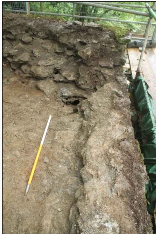
Photo 9: The partially dismantled western wall and southern return wall of the south-eastern abutment (DAT Photo 110511_0028)
