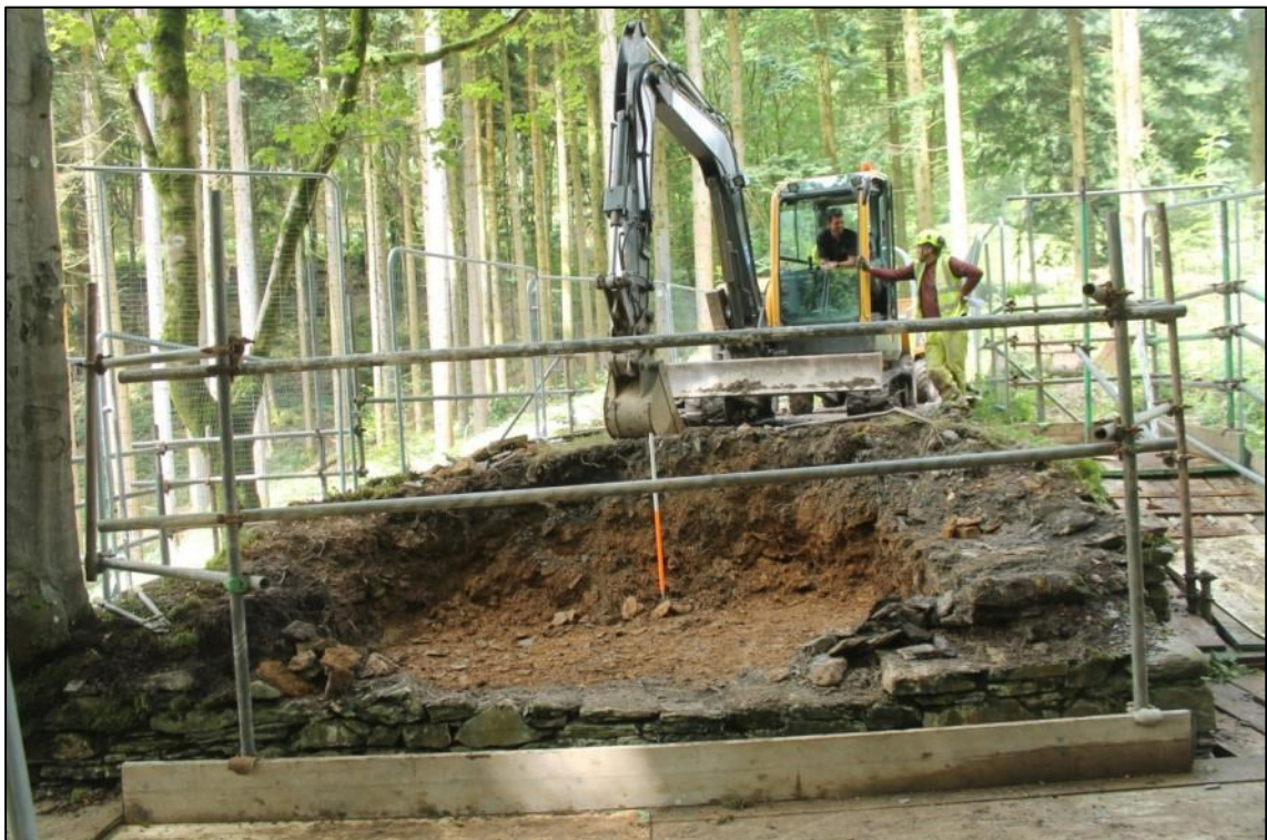
Photo 20: The section of the abutment infill and the reduced walls at the end of the excavations of the north-western abutment (DAT Photo 110511_0038).
