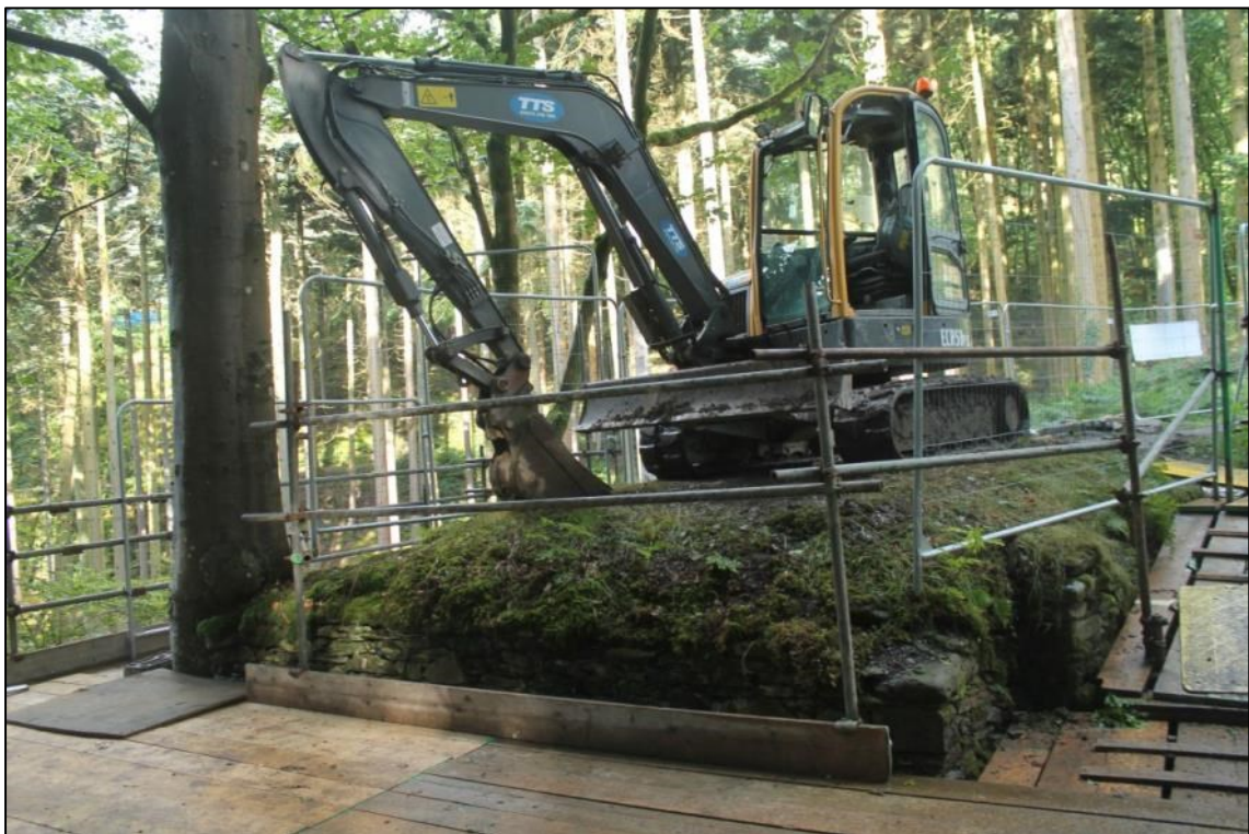
Photo 12: The north-western abutment prior to the start of works. Note the dogleg inset along the northern wall of the abutment (DAT Photo 110511_0031).
