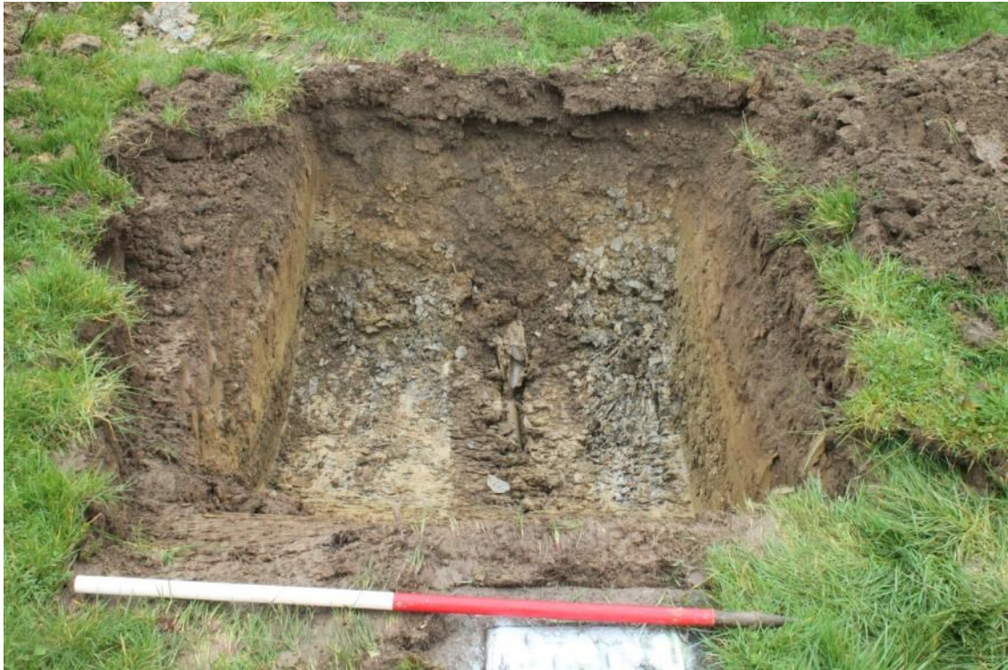
Photo 10: The trial trench upon completion of excavation. The trench was excavated to a depth of approximately 0.80m to the existing water mains. The natural (undisturbed) ground was exposed at this depth. View south, 1m scale.
