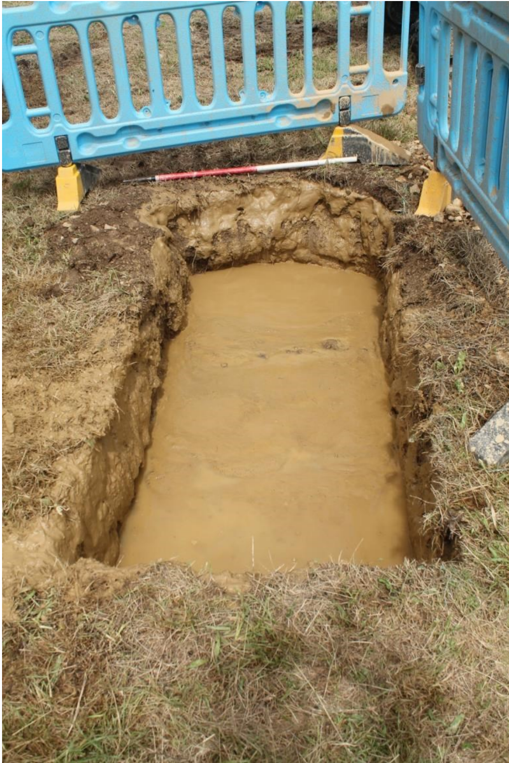
Photo 5: Looking north along T3. Bore hole leading to trench has been 'reamed', creating fluid mud in the trench. 1m scale
