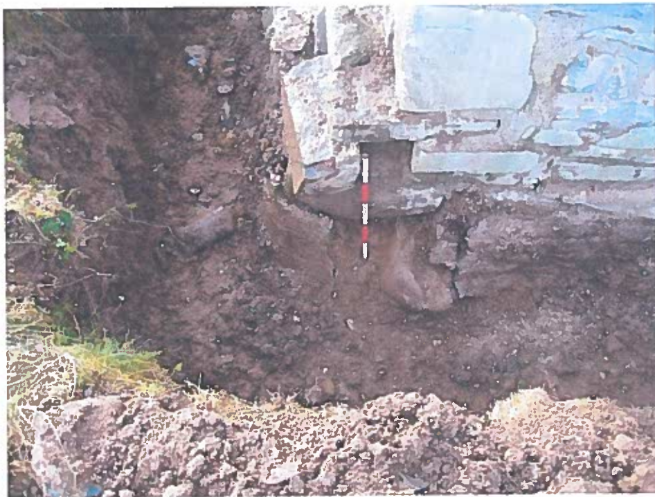
Plate 4: South corner of chancel showing early boulder foundation along south wall and 19 th century foundations below east wall
