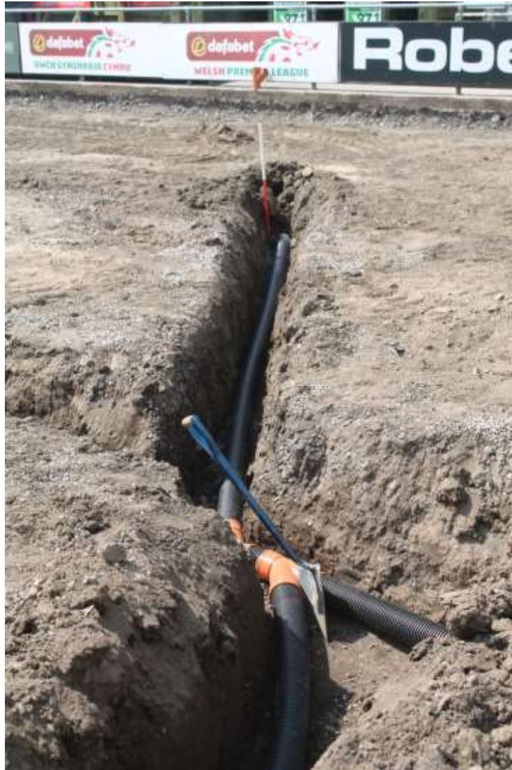
Photo 26: View south along re-excavated drainage trench at northern end of TB (Figure 9). 1m scale
