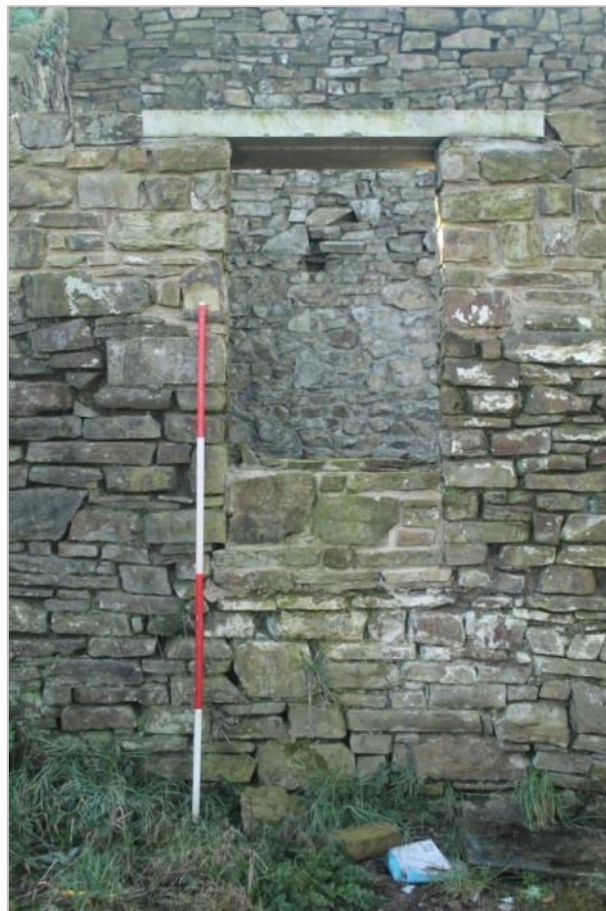
Photo 8: The infilled and partially rebuilt single window at the south-eastern end of the east facing elevation of Crundale Mill (DAT Photo 110325_0006).
