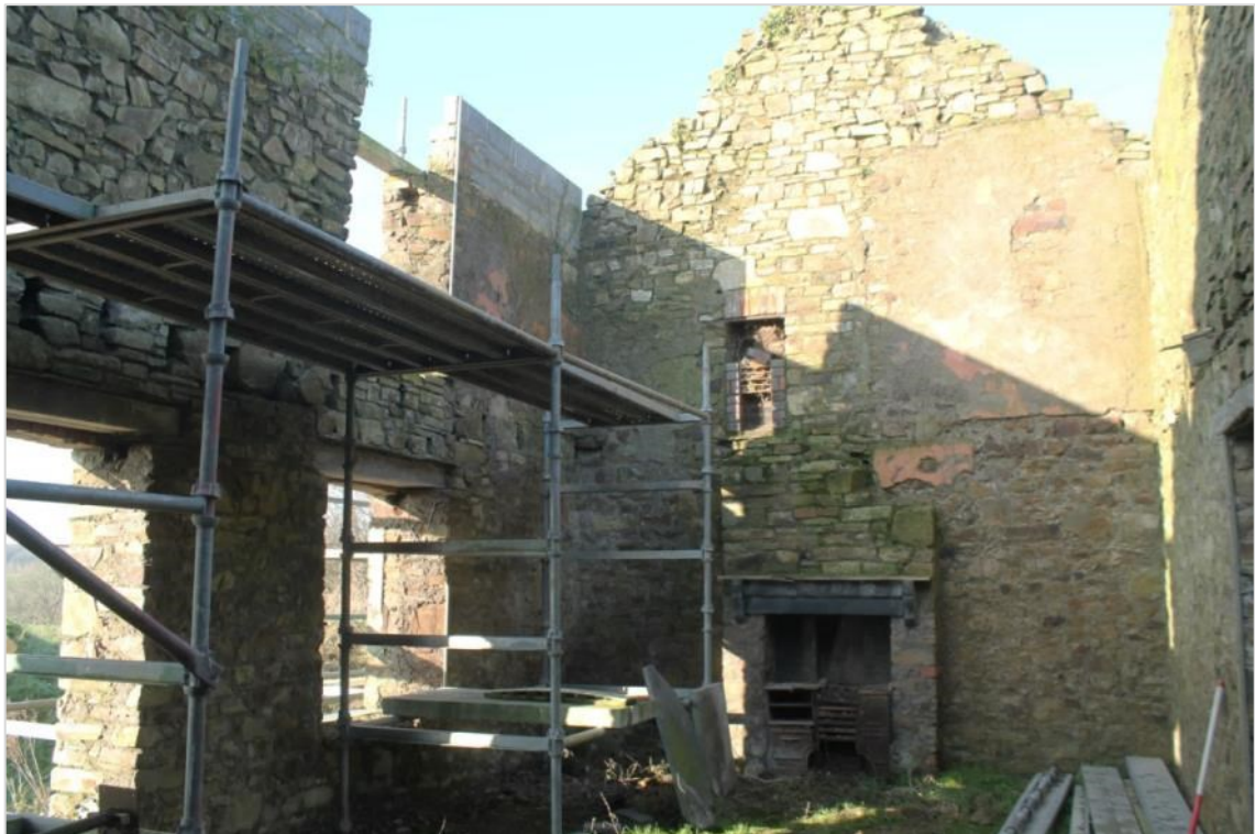
Photo 11: The internal face of the northern gable end with its in situ fireplaces (DAT Photo 110325_0035)
