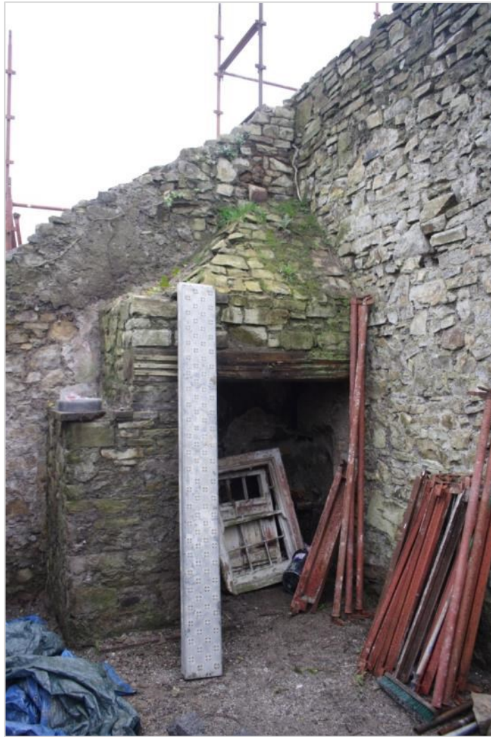
Photo 5: Remains of larger fireplace built into eastern part of building (southwestern corner) with remains of bread oven
