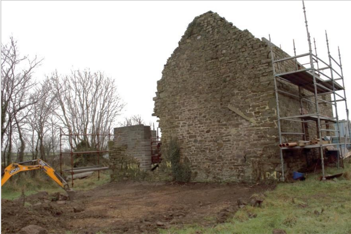
Photo 20: The stripped footprint of the proposed extension at the northern gable end of Crundale Mill (DAT Photo 110325_0048)
