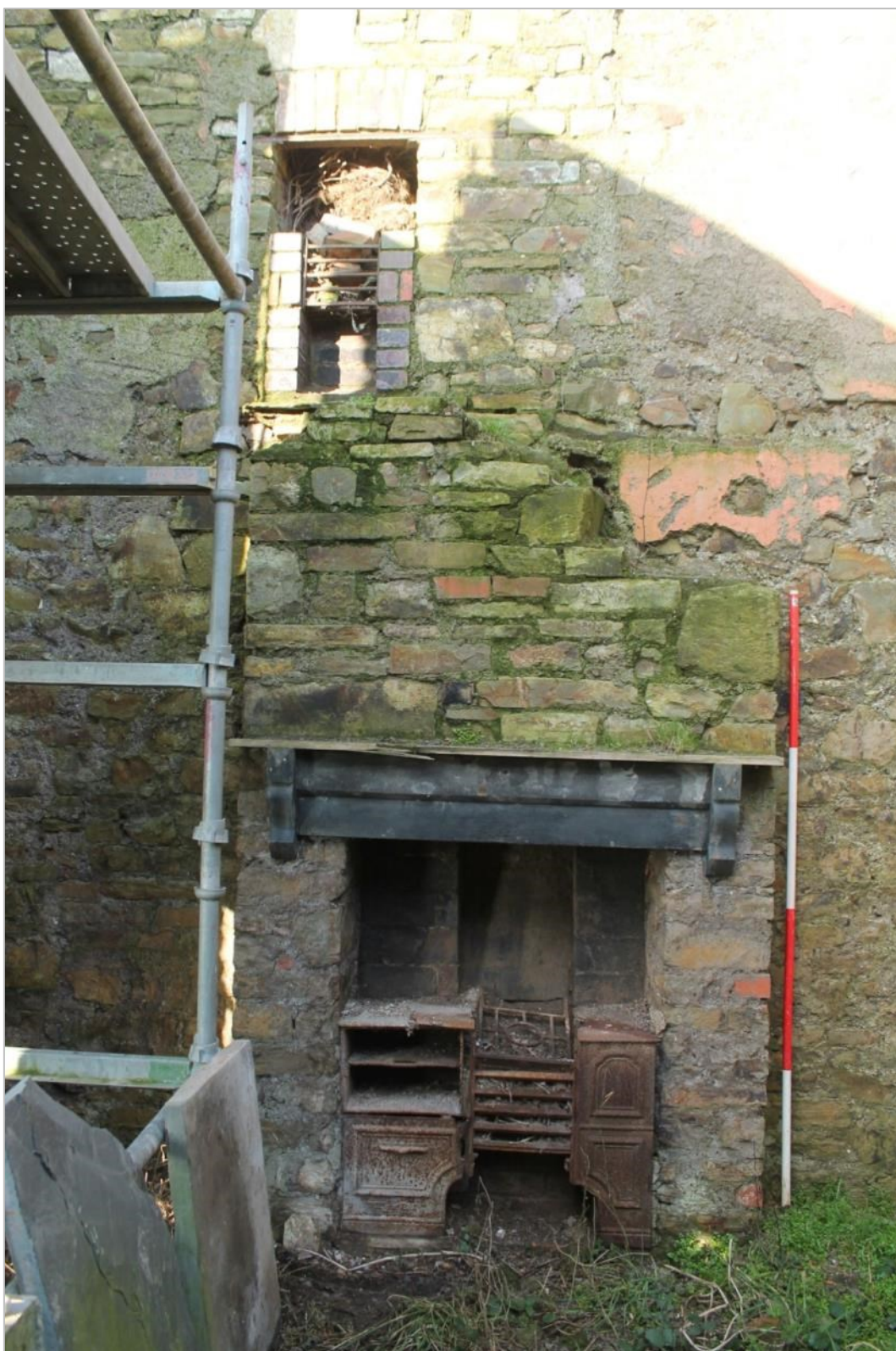
Photo 12: The iron range, firebrick lined flue and corbeled chimney breast of the ground floor fireplace in the northern gable end (DAT Photo 110325_0018)
