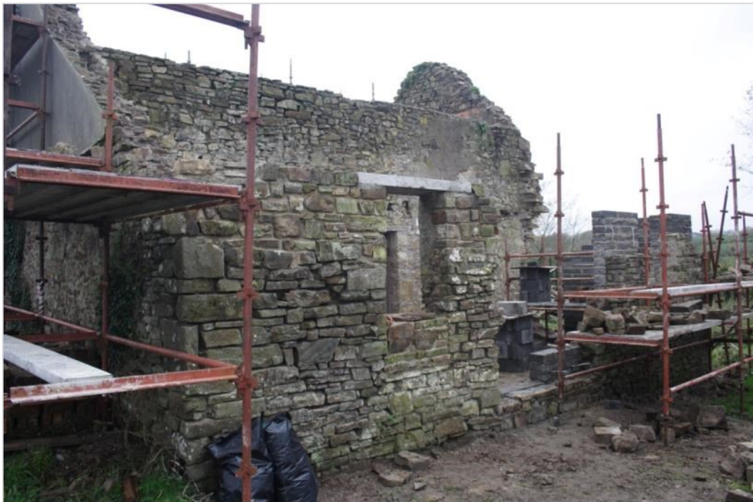
Photo 2: Eastern façade of the building, where some dismantling and rebuilding of the wall has been undertaken
