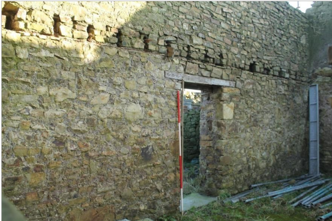
Photo 14: The west facing internal elevation of the partition wall in Crundale Mill and its central door and first floor beam slots (DAT Photo 110325_0027)
