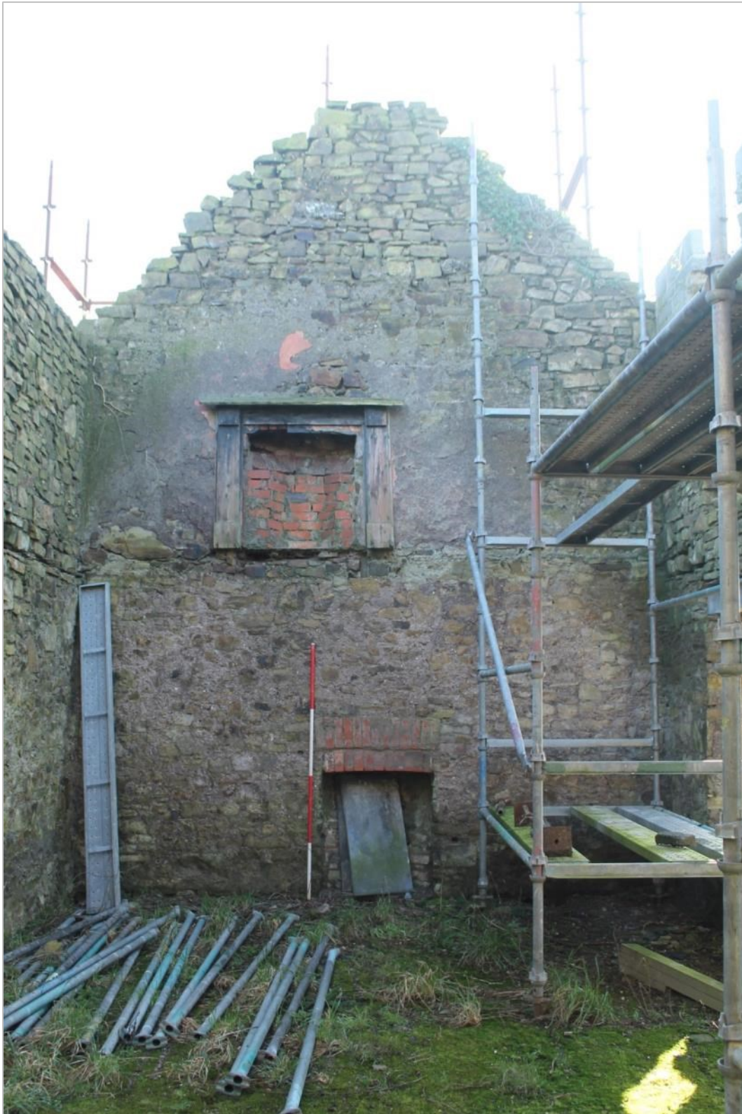
Photo 15: The internal elevation of the southern gable end with its two, in situ fireplaces (DAT Photo 110325_0024)
