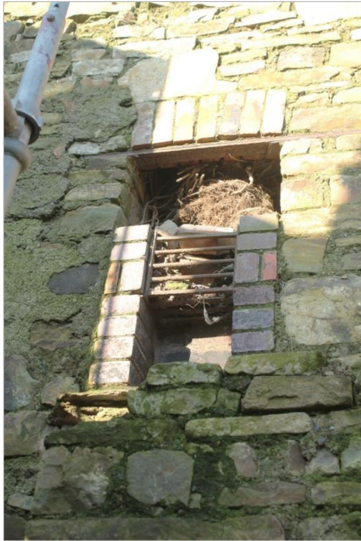
Photo 13: The single, brick lined first floor fireplace in the northern gable end (DAT Photo 110325_0023)
