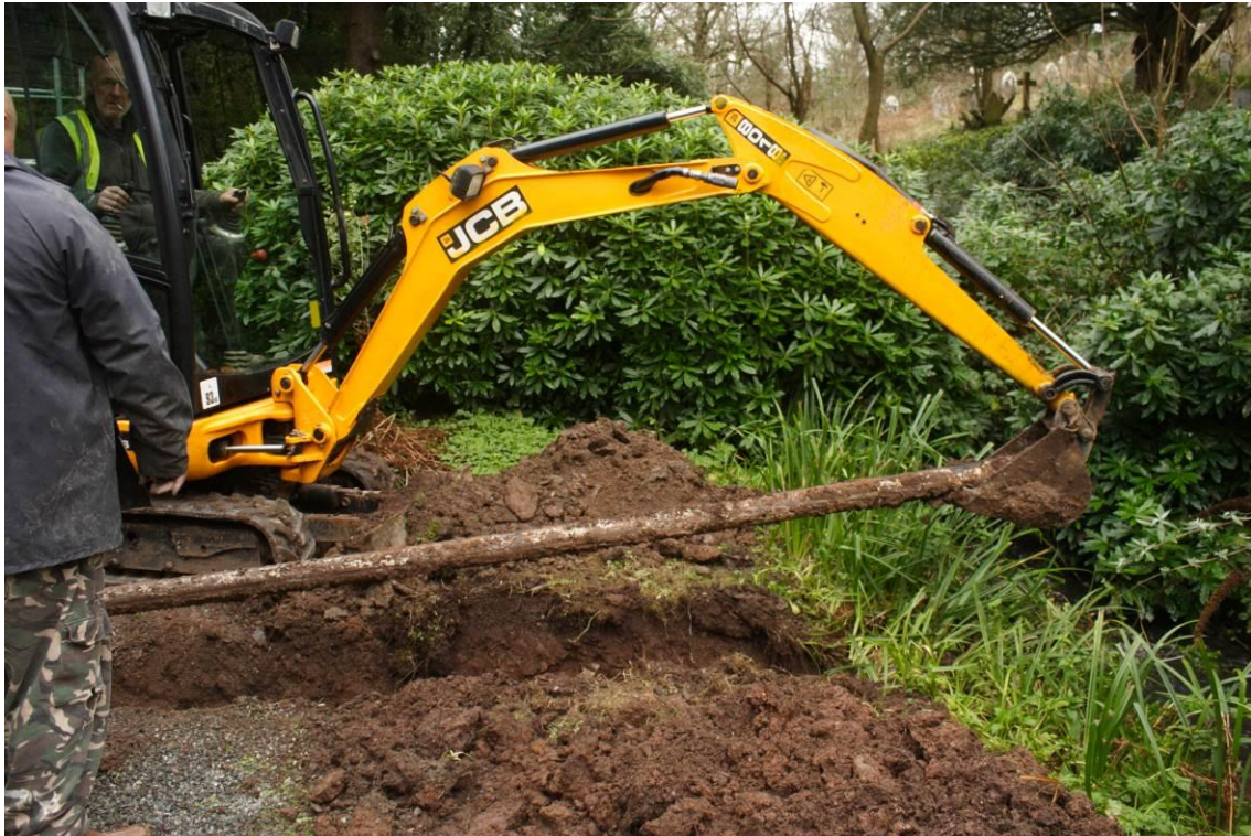
Photo 9: Looking east at removal of the steel drainage pipe in Trench 6.
