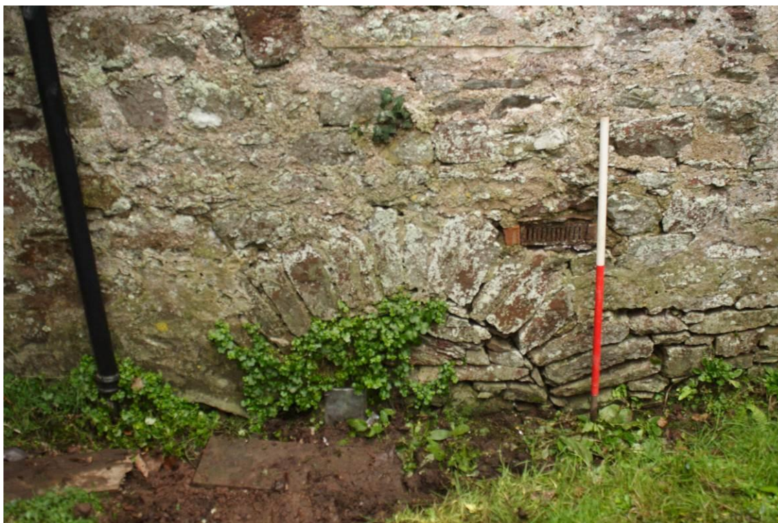
Photo 13: West facing wall of north transept showing blocked entrance to culvert that runs underneath north transept. 1m scale
