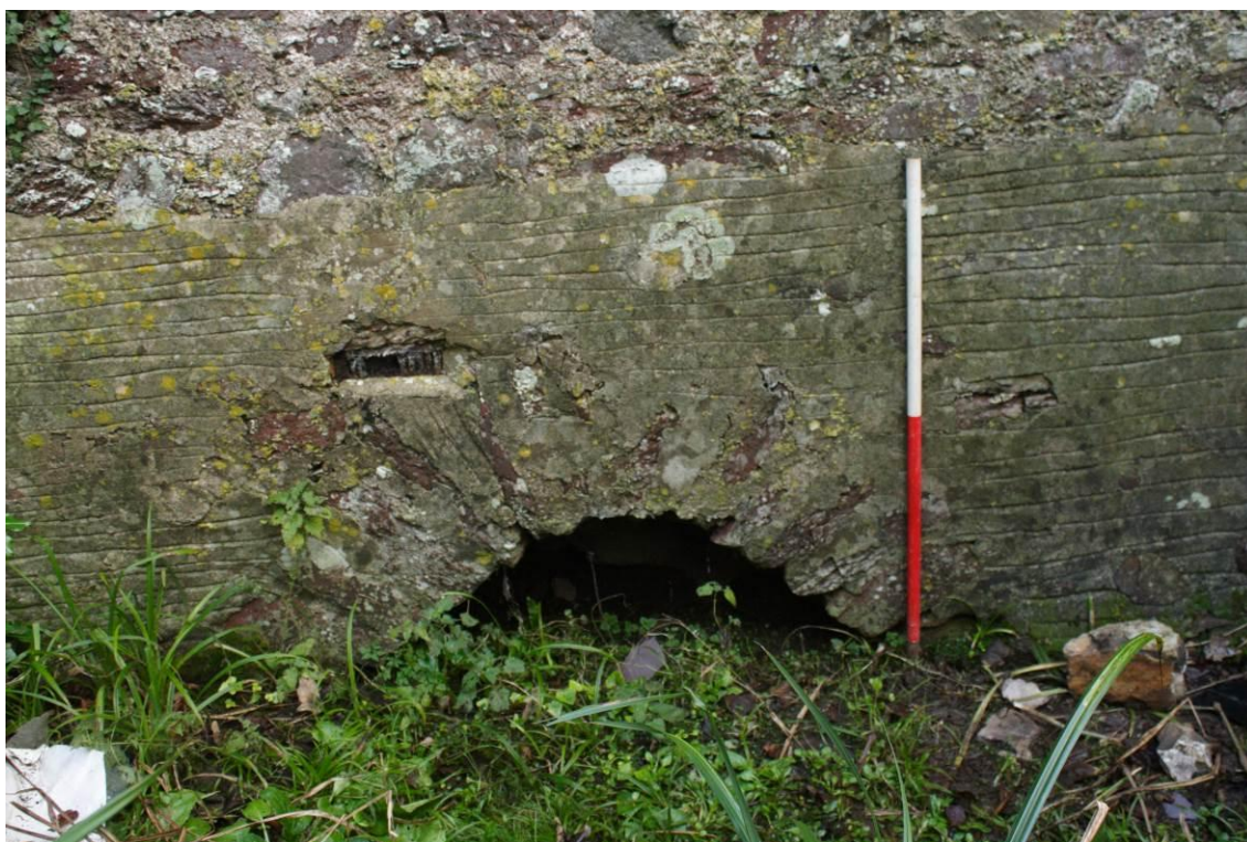
Photo 12: East facing wall of north transept showing culvert that runs underneath north transept. 1m scale
