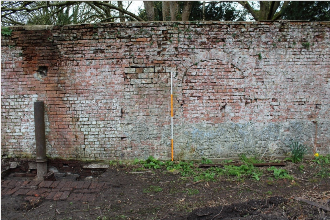
Photo 42: The south facing garden wall showing the blocked arched recess of the earlier Glasshouse 4. It also shows the cast iron cylindrical flue seen in Photo 41 and behind the reddened heat affected brick flue within the wall. 2m scale
