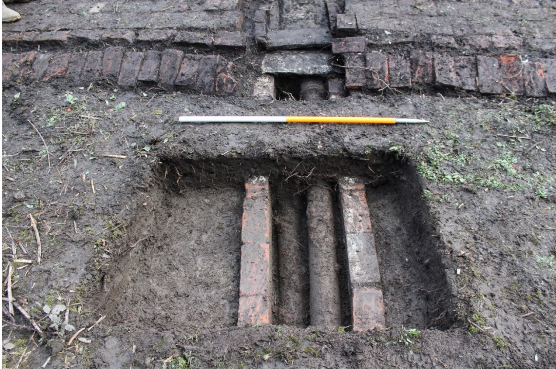
Photo 38: The two heating pipes running underground in a northwest direction from Glasshouse 2. They sit within an uncapped brick edged channel. Looking northwest. 1m scale
