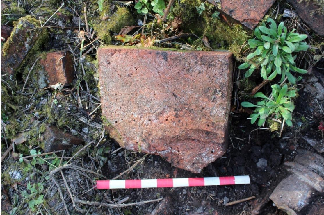
Photo 40: The perforated underside of one of the ceramic slabs on which the heating pipes were placed. 0.5m scale
