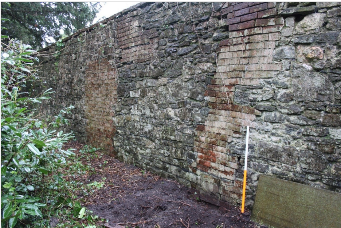
Photo 43: The north facing garden wall showing the other side of the heat affected brick flue seen in Photo 41. Note the blocked square hole at the bottom of the flue. 1m scale
