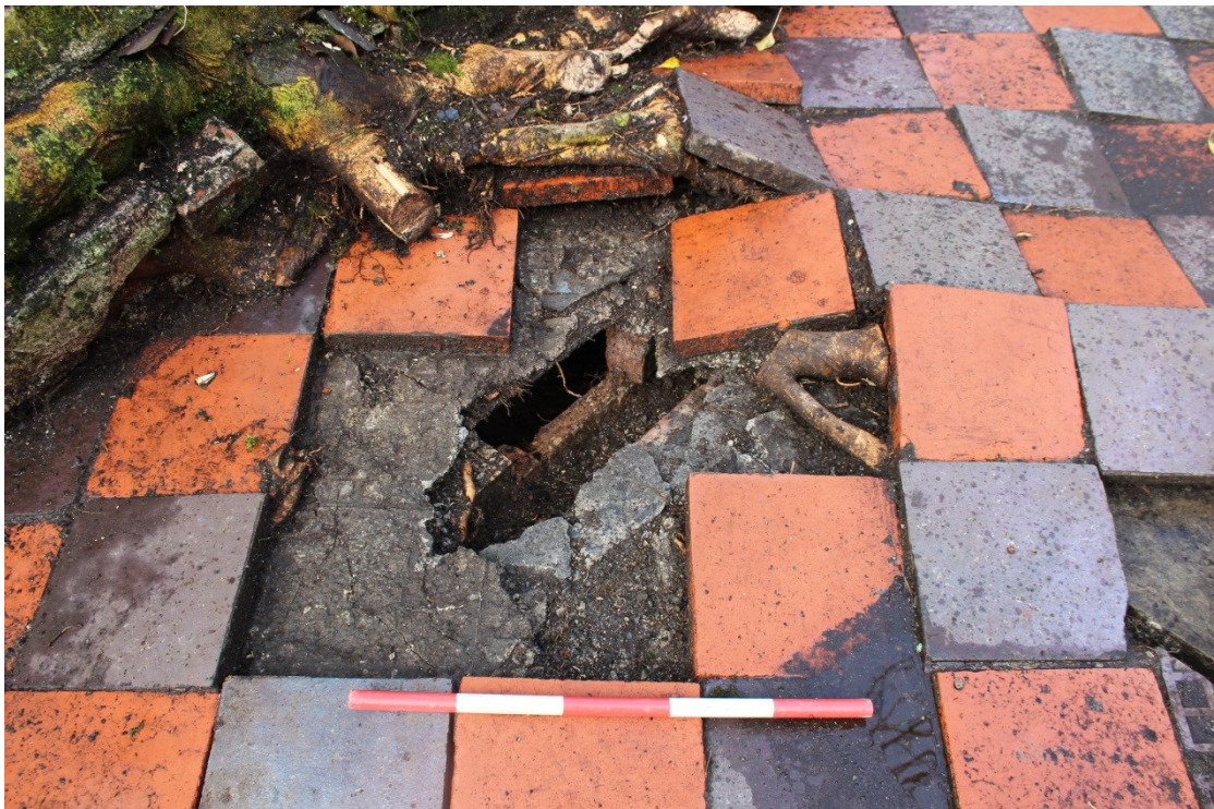
Photo 14: Photo showing the cavity below and brick supporting wall to the earlier stone floor. 0.5m scale
