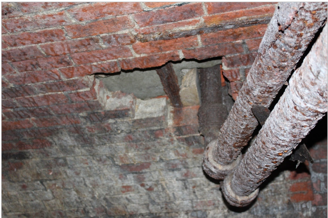
Photo 25: The two cast iron pipes running upwards to the glasshouse above through a hole made in the brick vaulted roof.
