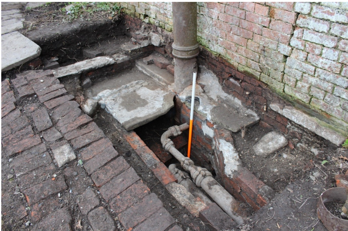
Photo 37: The two heating pipes reduced from 4" to 2" inch that then run under the north garden wall. Note the cast iron cylindrical flue. Looking west. 1m scale
