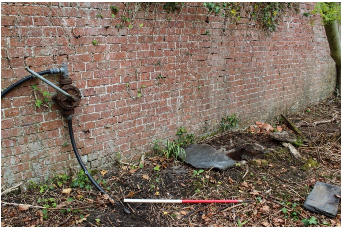
Photo 52: The hand crank pump with the opening to the cistern shaft to the right just after its covering of slabs was removed. 1m scale
