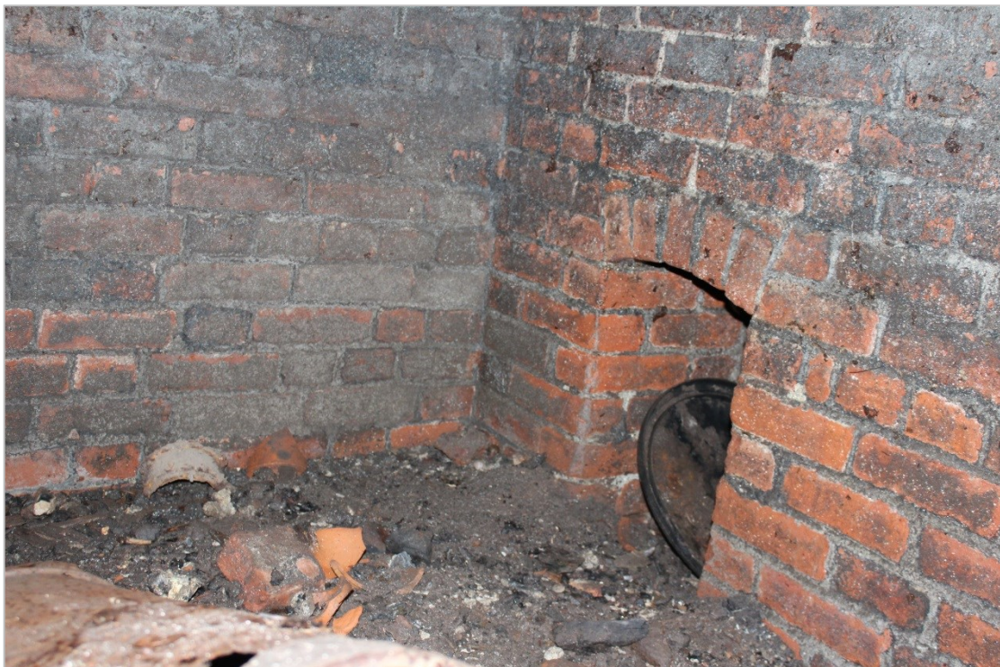
Photo 22: The east wall of the boiler house showing the bricked arched recess at floor level.
