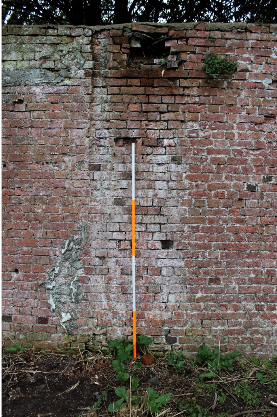
Photo 48: Close up of the brick flue within the north wall that possibly marks the east end of the extended Orangery. 2m scale
