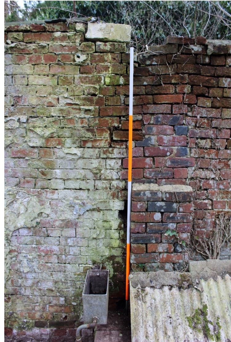
Photo 12: Evidence of a brick flue within the east wall at the south end of Glasshouse 1. 2m scale
