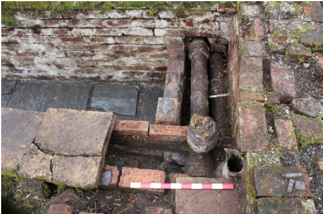
Photo 39: The east end of Glasshouse 2 showing the main heating pipes and the remains of the vertical feed and return pipes. Looking roughly northwest. 0.5m scale
