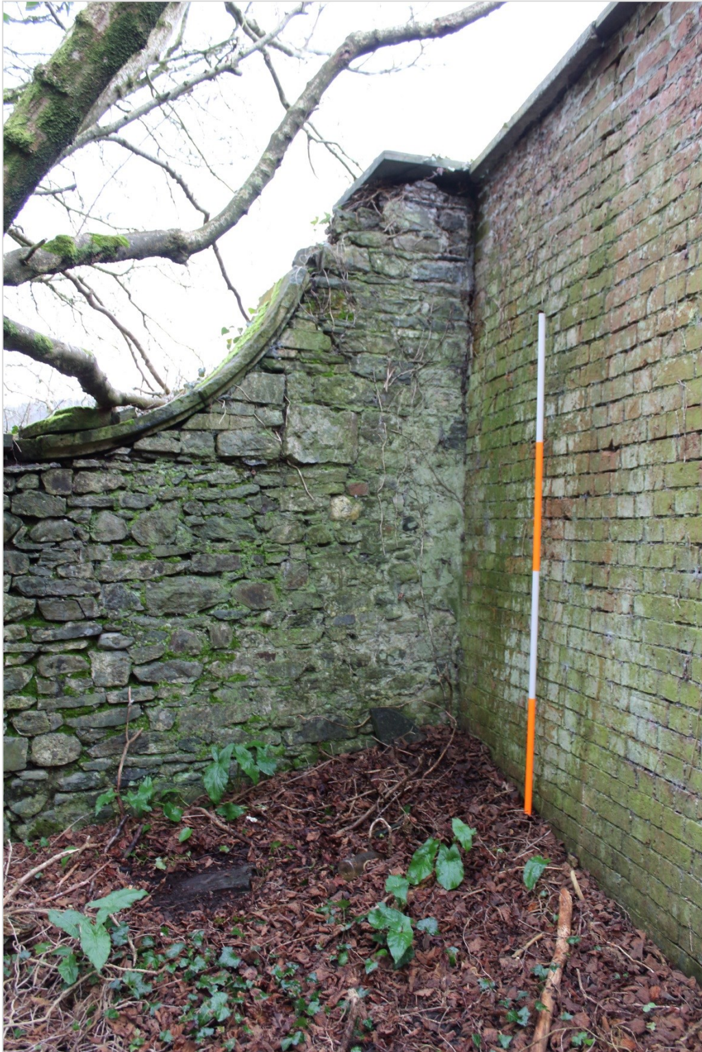
Photo 61: The southwest corner of the walled garden showing the later stone built south wall where it butts the west brick wall. 2m scale
