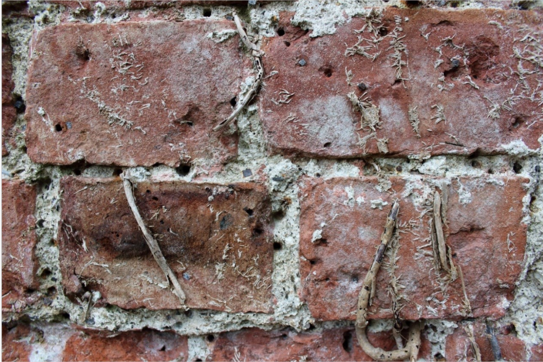
Photo 62: Close up of the some of the many small nail holes (some nails still in situ ) within the south facing wall of the walled garden.
