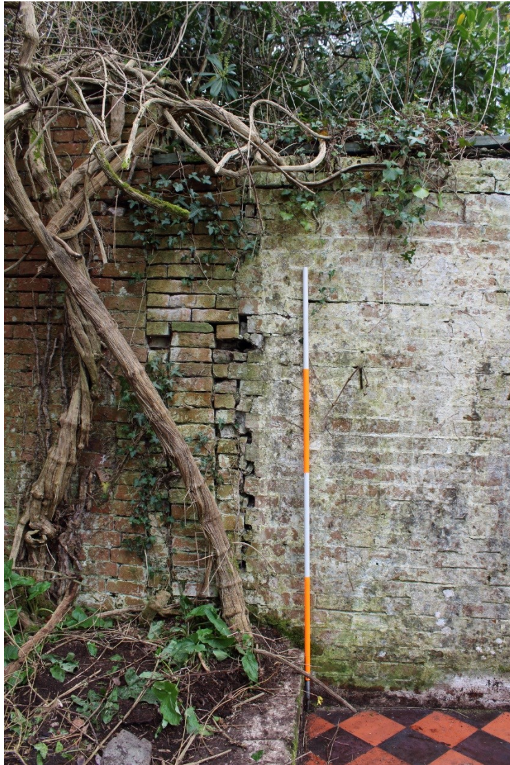
Photo 11: Evidence of a brick flue within the east wall at the north end of Glasshouse 1. 2m scale
