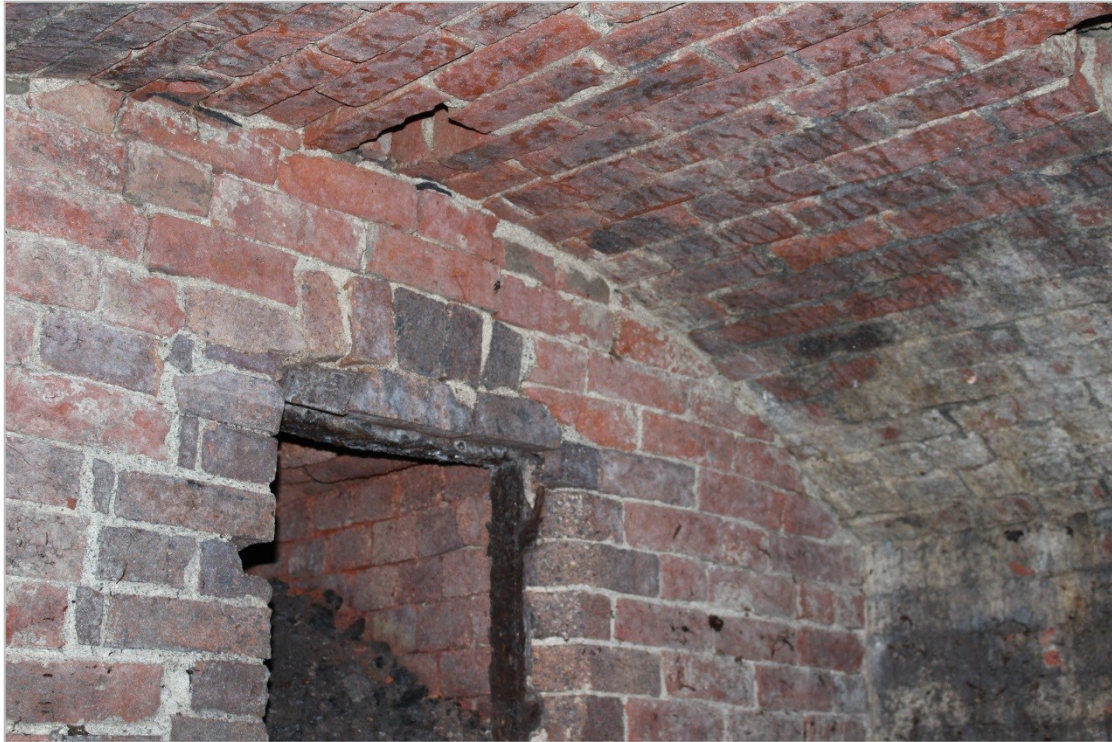
Photo 21: Photo showing the roof and west wall of the brick vaulted chamber of the underground boiler house to Glasshouse 1.
