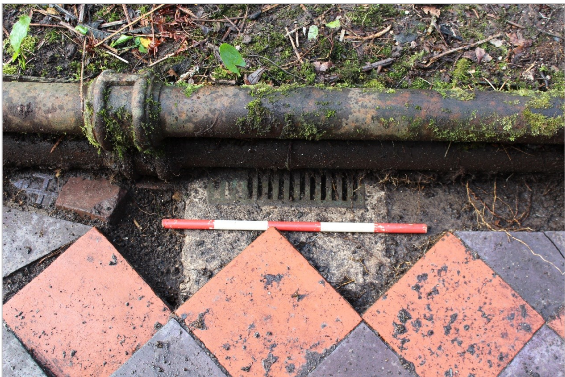
Photo 16: Detail of the rectangular metal vent set into the stone floor on the east side of the central cultivation bed. 0.5m scale
