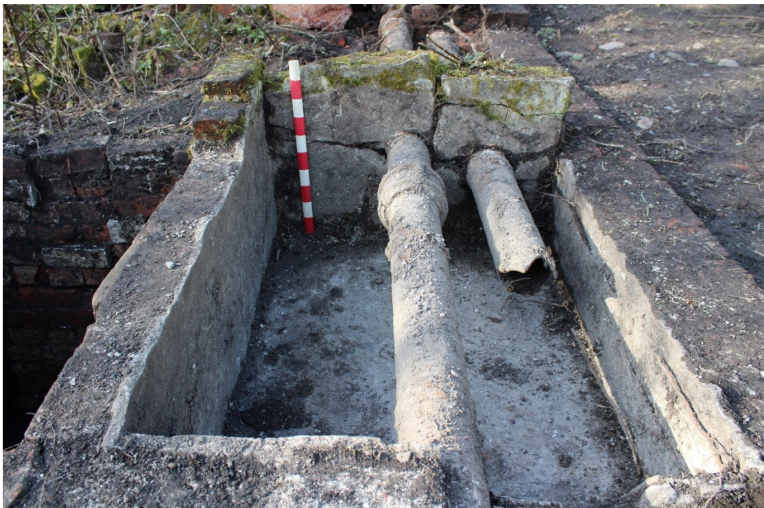
Photo 41: The evaporating tank at the east end of Glasshouse 3 through which the heating pipes passed. Looking roughly northwest. 0.5m scale
