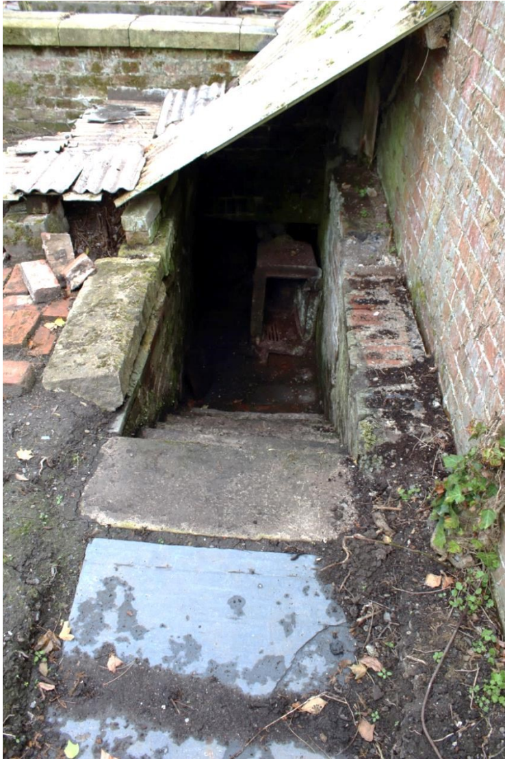
Photo 19: Photo showing the corrugated asbestos roof and steps down to the boiler house of Glasshouse 1. The small cast iron boiler can be seen at the bottom of the steps. Looking north.
