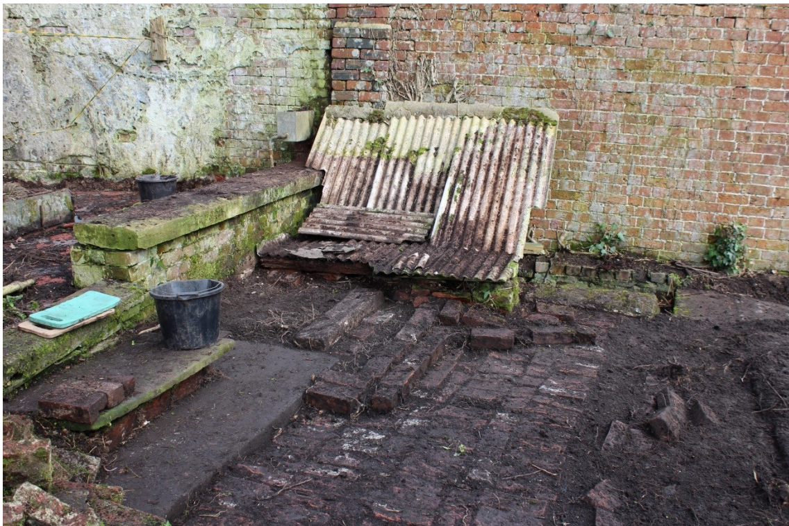
Photo 18: Photo showing the corrugated asbestos roof to the boiler house of Glasshouse 1. Looking east
