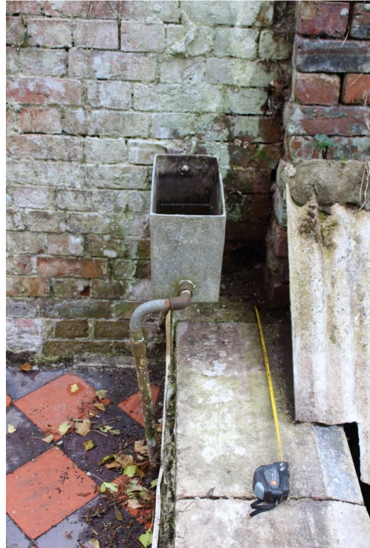
Photo 20: Photo showing the header tank to the boiler house of Glasshouse1. Looking east
