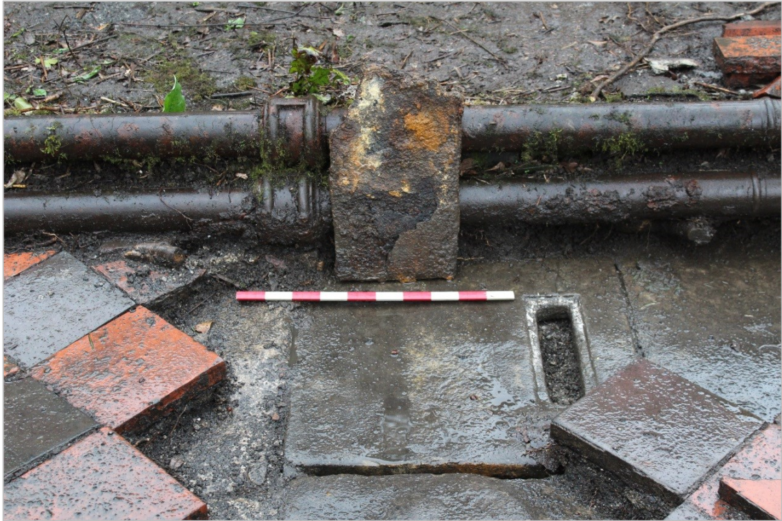
Photo 26: Photo showing the corroded cast iron sheet found within the narrow slot to the west of the possible vent set into the stone floor on the west side of the central cultivation bed. 0.5m scale
