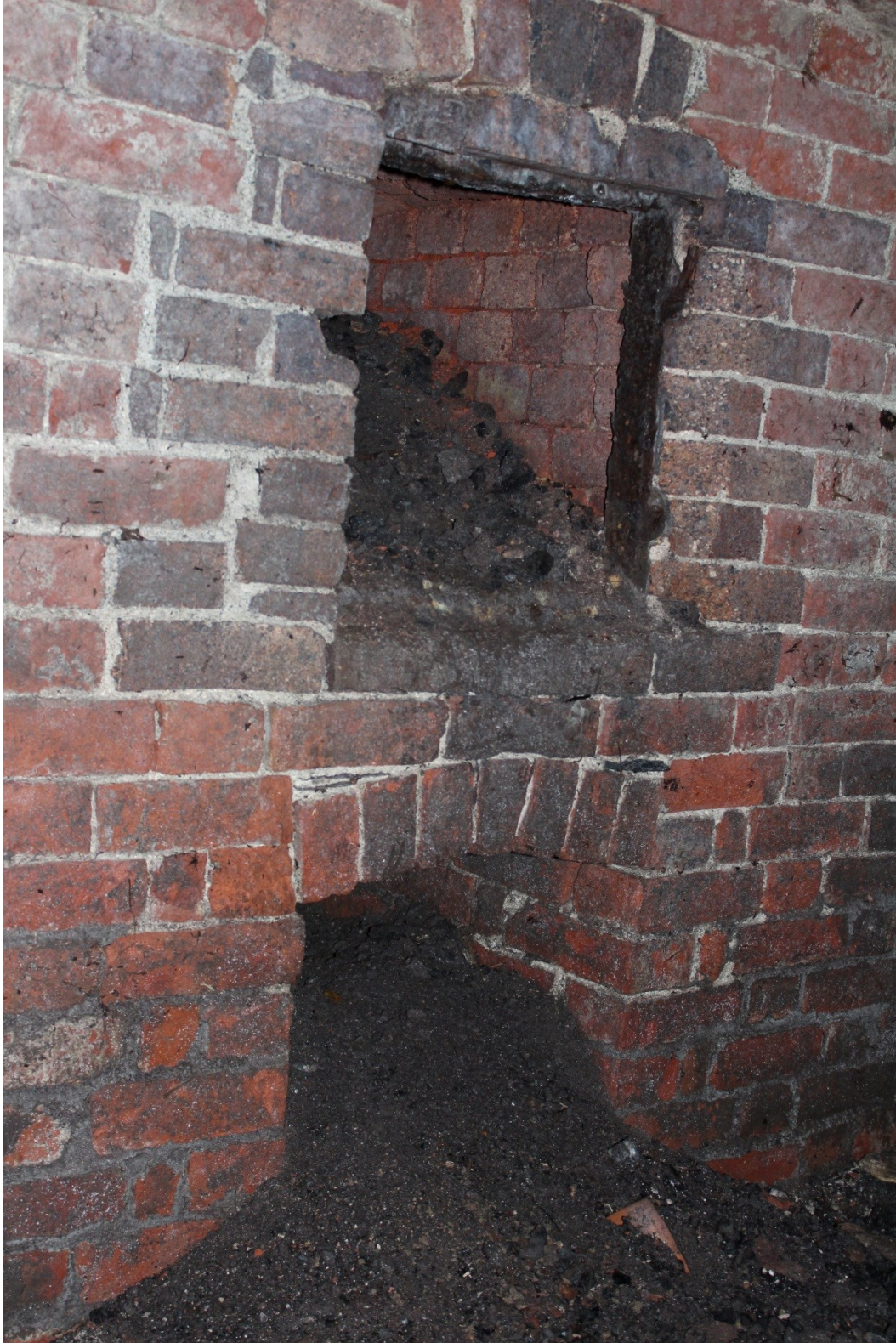
Photo 23: The west wall of the boiler house showing two bricked arched recesses. The upper one would appear to have been a firebox and the lower (at floor level) was probably for ash clean out.
