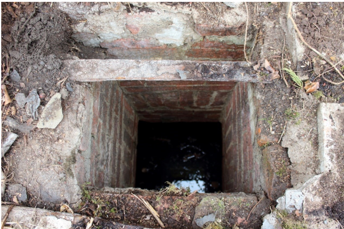
Photo 54: The square brick shaft to the cistern showing water below.
