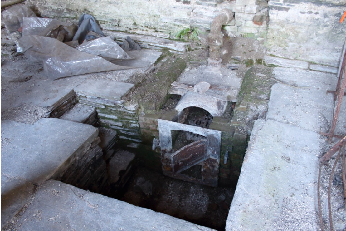
Photo 64: The underground boiler at Glanarberth House, Ceredigion (PRN 57526)
