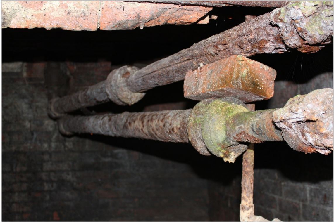
Photo 24: The two cast iron pipes that run northwards from the boiler. Bricks and pieces of wood have been used to separate the pipes. The narrower pipe in the background is from the header tank shown in Figure 10.
