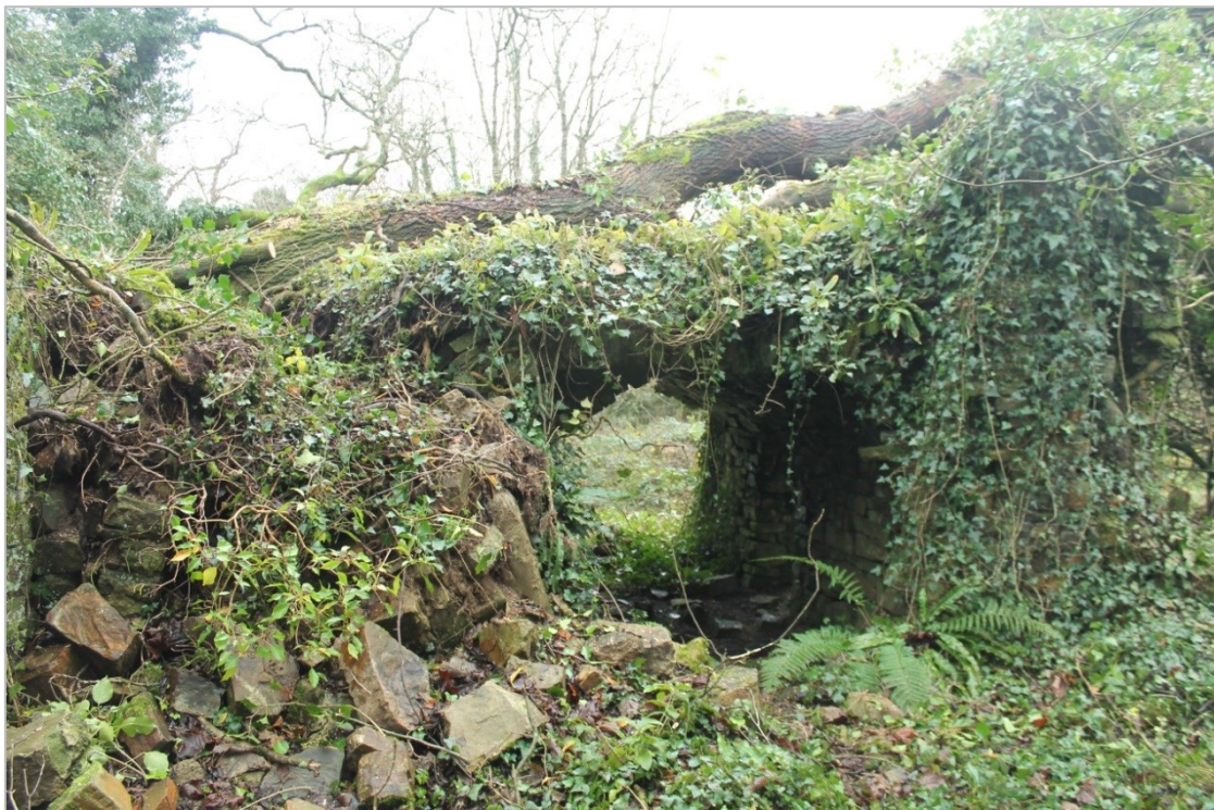
Photo 4: Looking roughly south towards the vaults in 2016 showing the damage caused to the eastern vault by the collapsed tree that can be seen lying across the top of the structure.
