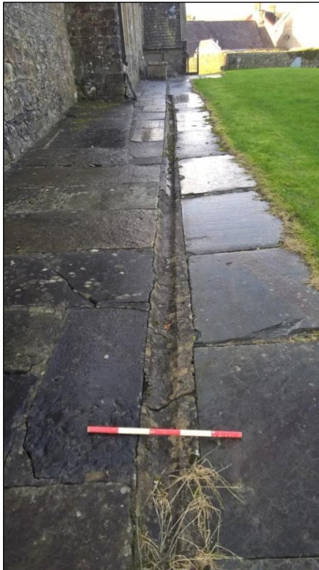
Photo 7: The concrete cast drain running along the northern side of the church. This is due to be demolished and replaced with a new concrete drain. 0.5m scale (DAT Photo 110315-0014)
