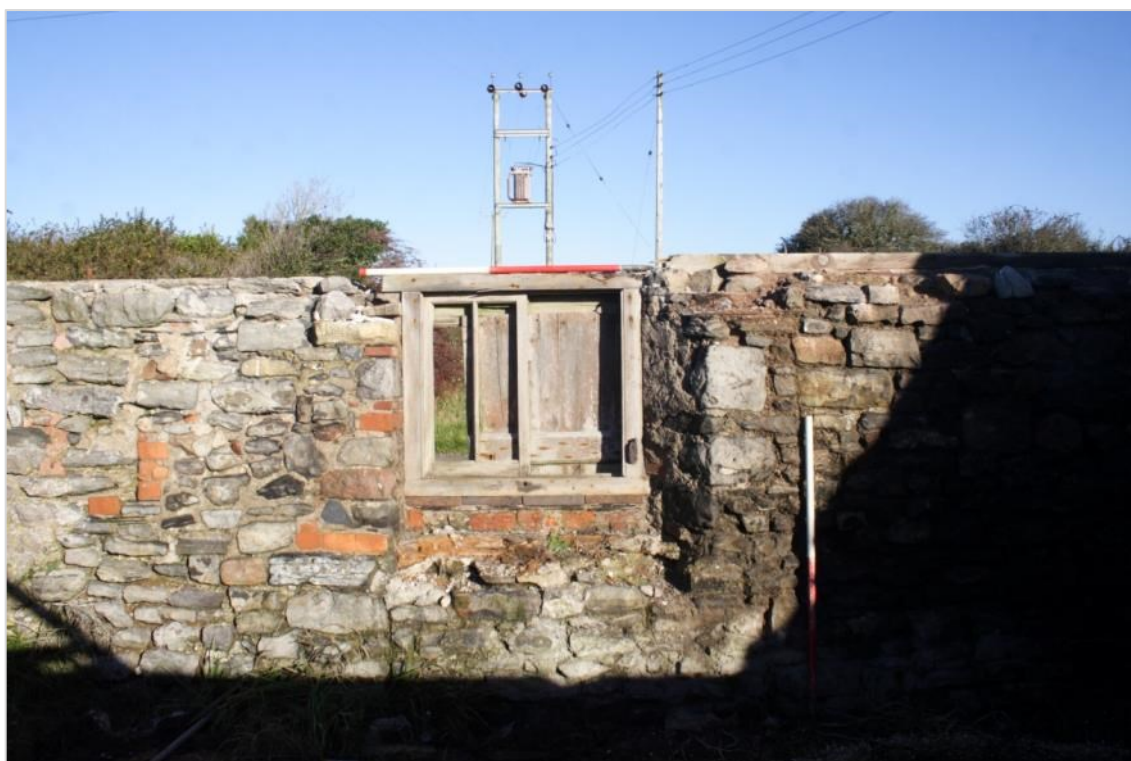
Photo 44: Timber framed window, partially splayed window in smithy. 2 x 1m scales
