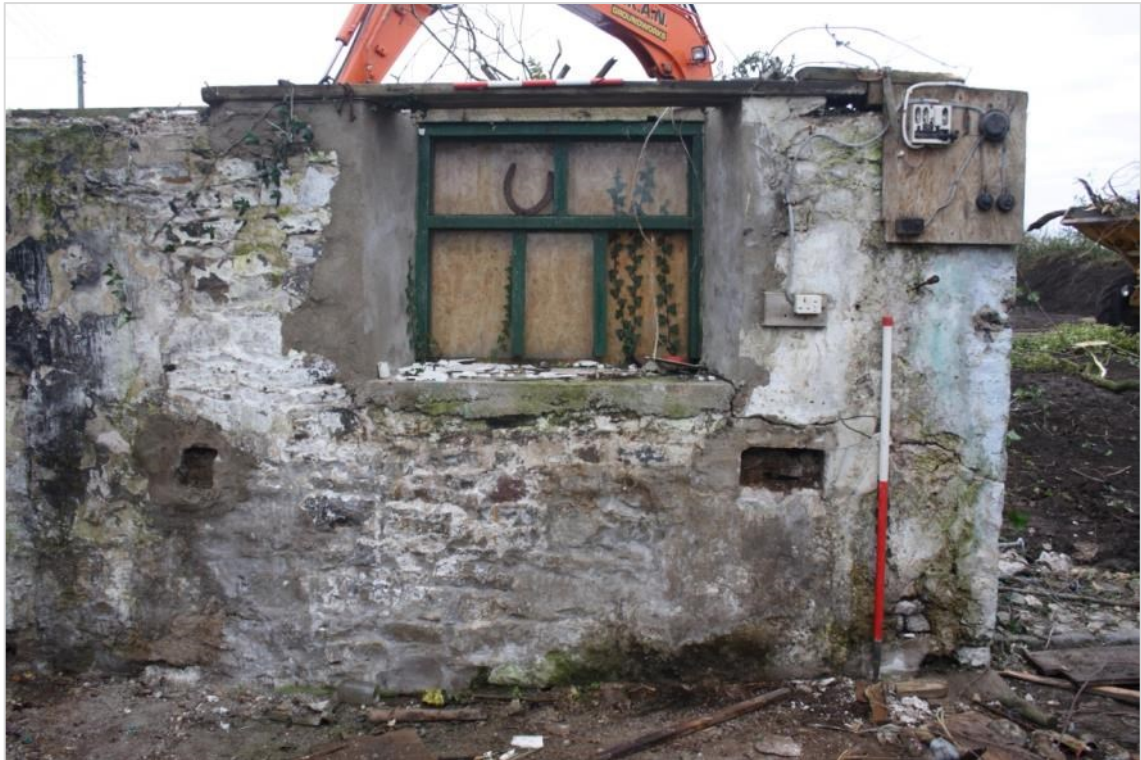
Photo 22: Timber framed window and cemented sockets in wall. 1m & 0.5m scales
