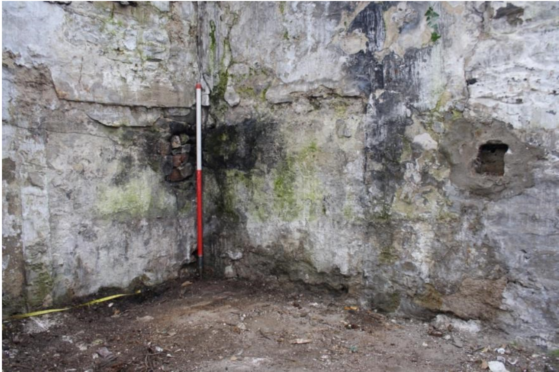
Photo 26: SE corner of cottage; cemented socket and scars on wall. 1m scale
