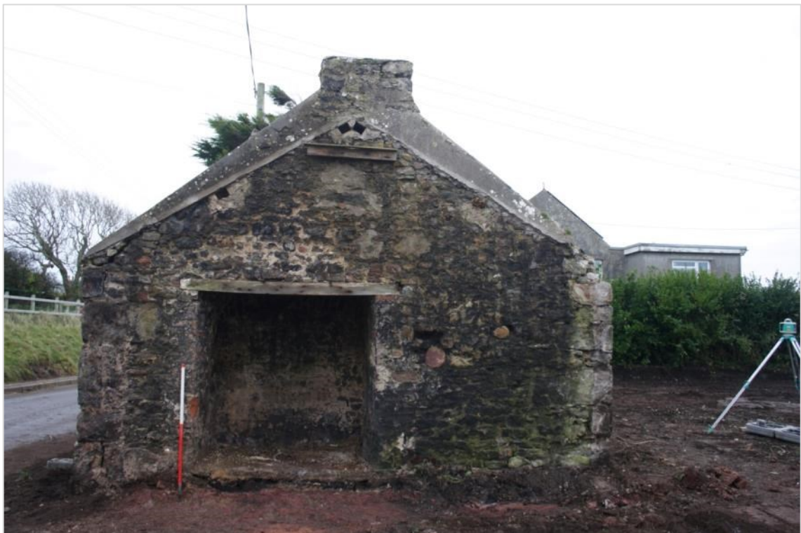
Photo 46: View of fireplace in smithy after removal of walls. 1m scale
