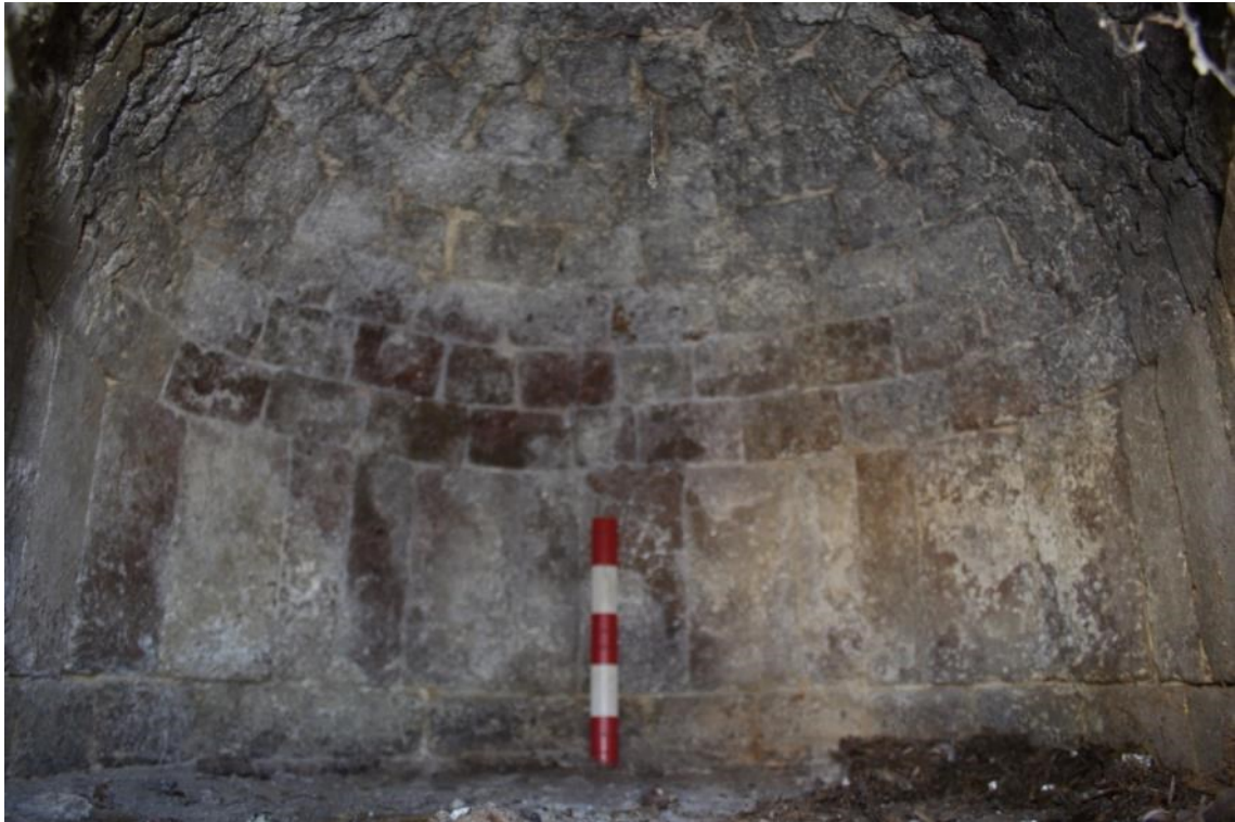
Photo 13: Brickwork inside oven. 0.25m scale
