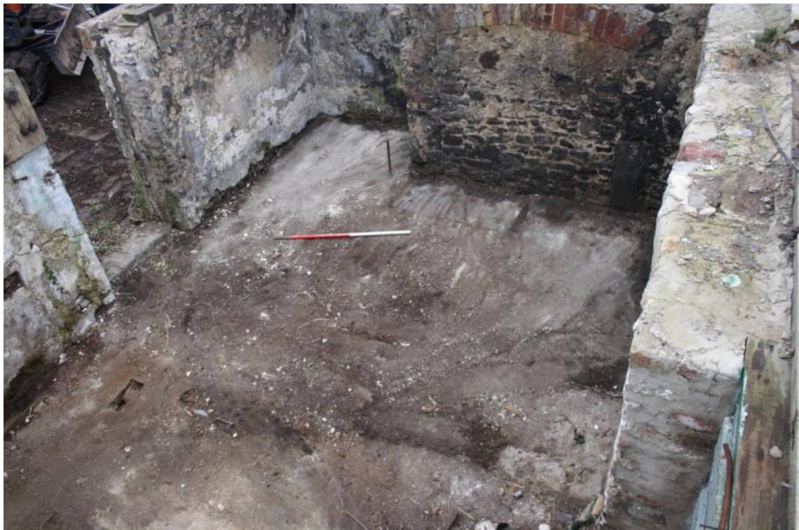
Photo 25: Cement floor, rear doorway and blocked chimney. 1m scale
