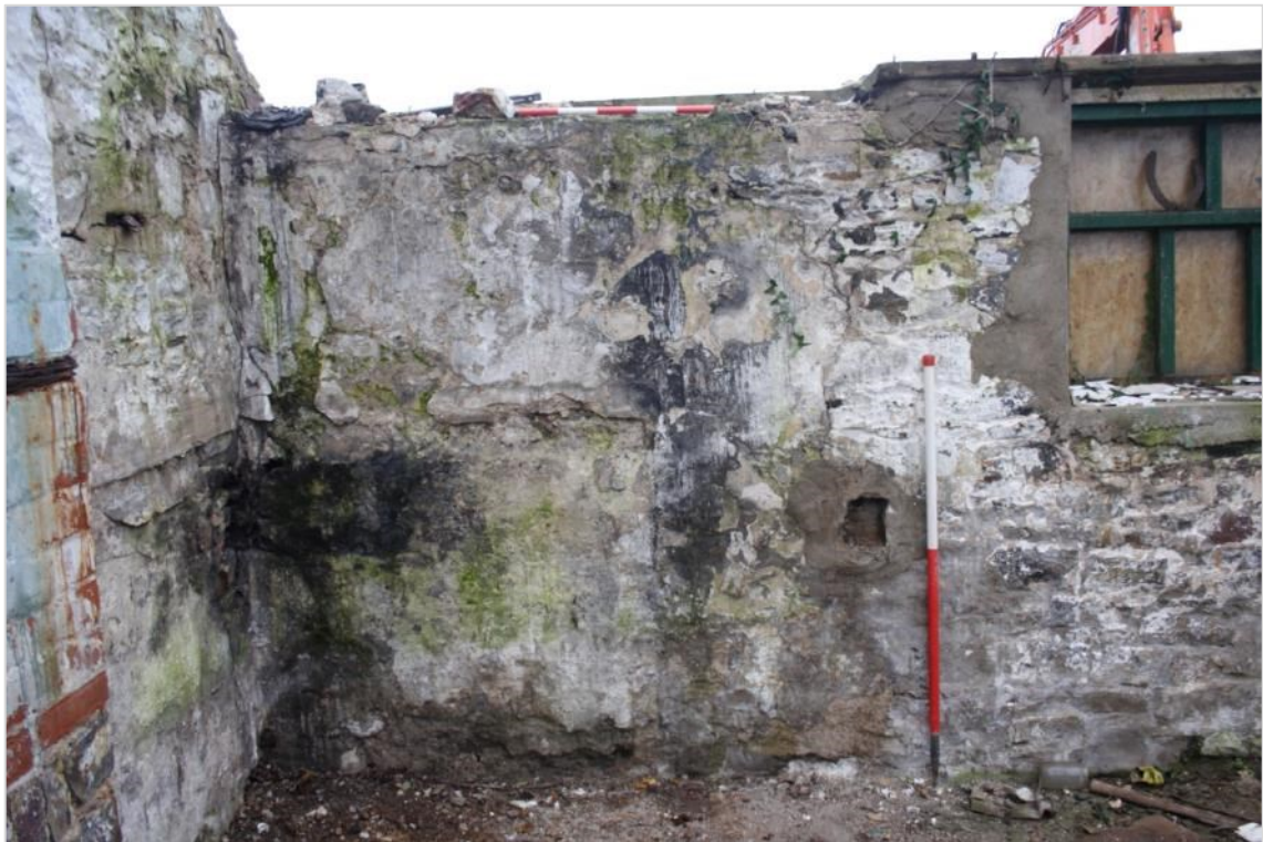
Photo 21: SE end of wall showing scarring and cemented sockets. 1m & 0.5m scales
