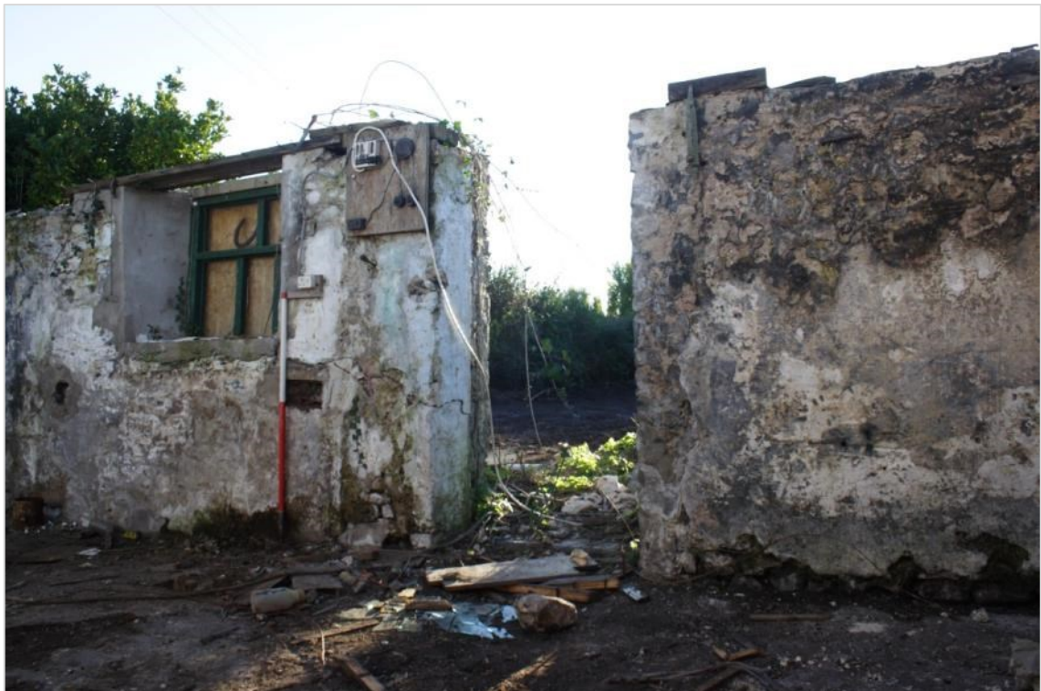
Photo 10: View south of cottage interior showing widened window, later sockets inserted in wall and paint scar possibly indicating former internal wall. 1m scale
