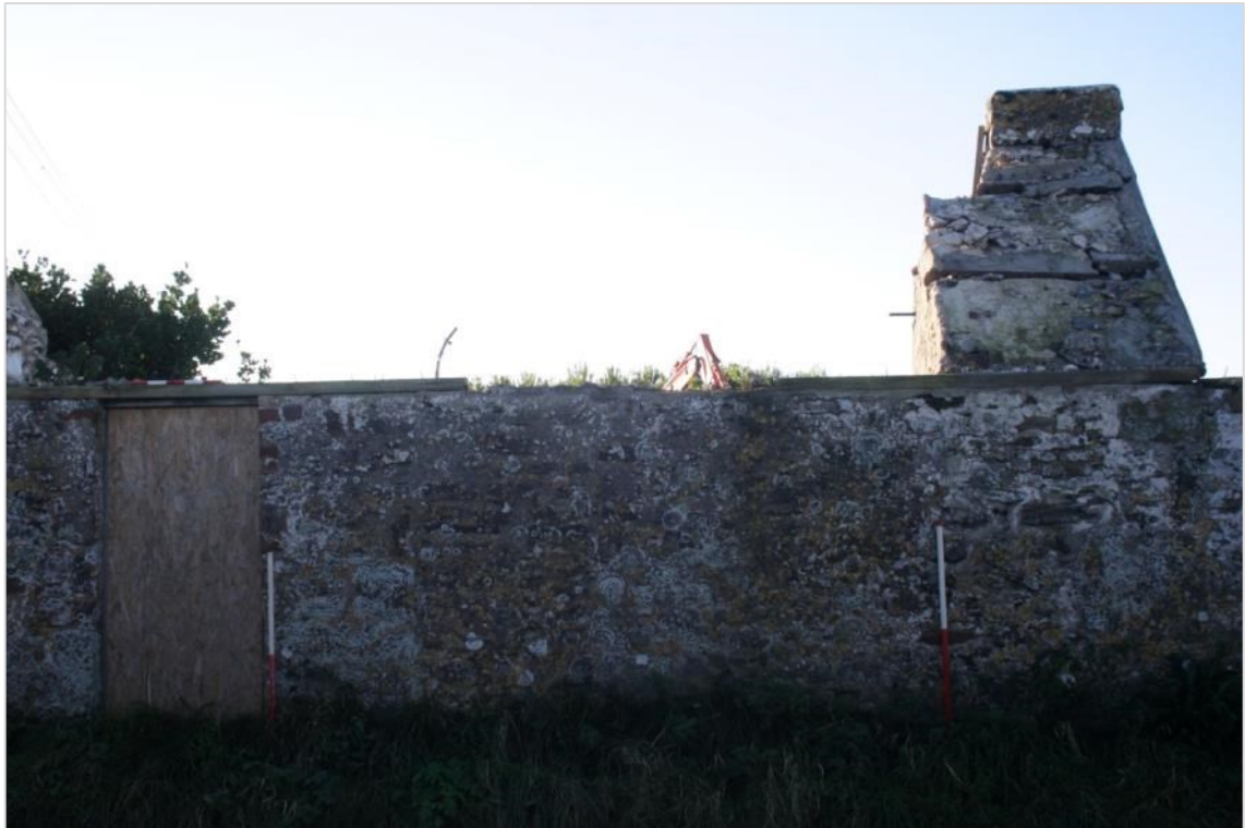
Photo 3: Centre of building showing doorway, blocked window and internal wall dividing smithy and dwelling. 2 x 2m scales
