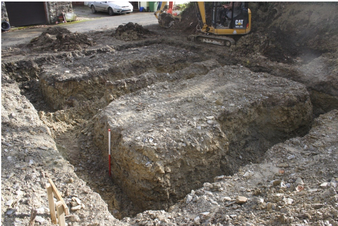
Photo 10: View SE across site showing completed foundation trenches. 1m scale
