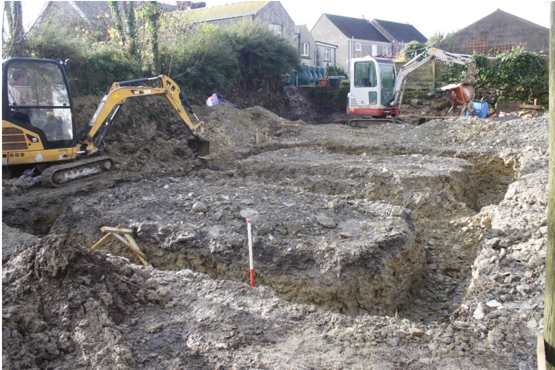
Photo 9: View west across site showing completed foundation trenches. 1m scale
