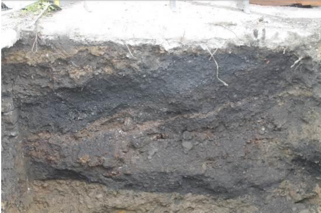
Photo 5: The south-facing section of the trench (quay wall to left), showing the sloping layers of material making up the quay on top of a relatively flat layer of re-deposited river material
