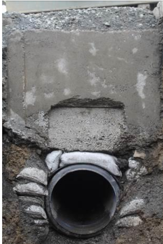
Photo 13: The eastern face of the trench, showing the previously installed pipe, 0.7m in diameter with its top lip at a depth of about 1.8m.
