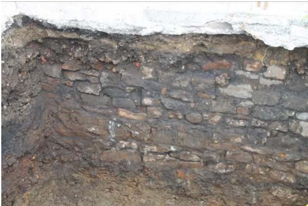
Photo 10: Inner face of the quay wall, southern end of the trench, looking west
