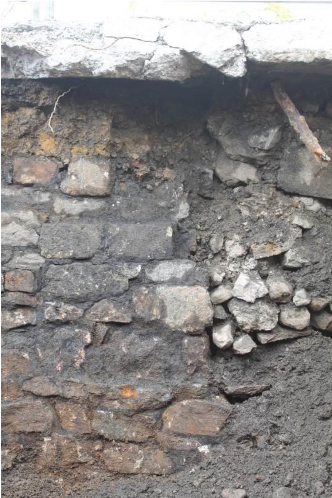
Photo 12: The inner face of the quay wall near to the northern edge of the trench. On the left side of the image the wall's stepped construction can be seen along with the change in coursing towards the base. On the right, the disturbed area of the wall shows, backfilled with stone and with the old metal pipe containing an electrical cable hanging down beneath the concrete.
