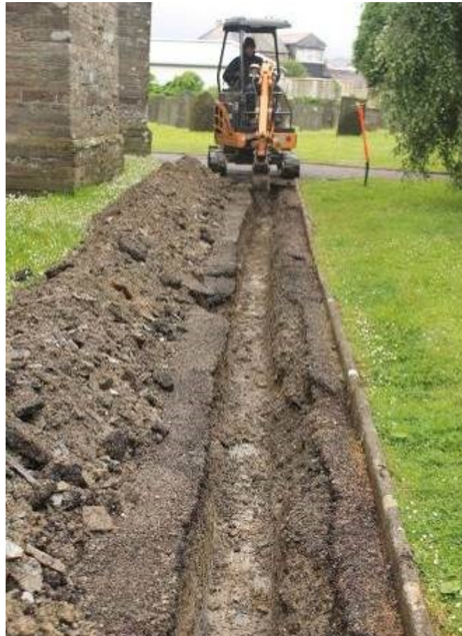
Photo 10: The western end of the long straight section of the new drainage channel cut through the tarmac path along the north side of the church
