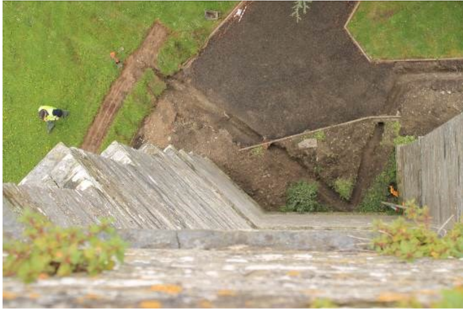
Photo 11: Plan view of the groundworks at the west end of the north side of the church. Two drainage ditches leave the church wall, one heading northwest towards the new soakaway in the grass, and the other heading for the longer drainage channel cut through the tarmac path along the north side of the church
