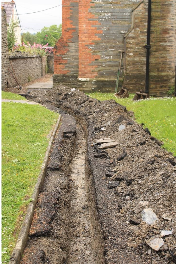
Photo 1: The eastern end of the new drainage channel, cut through the tarmac path on the north side of the church
