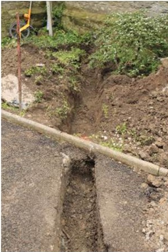
Photo 13: The short section of drainage channel excavated between north church wall near its west end and the soakaway, looking southwest
