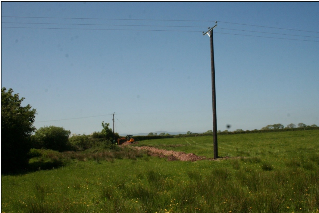
Photo 12: The underground cable trench (T11) running from the newly erected post in T3 in the foreground to an original post alongside the western boundary of the field, visible in the background. (DAT Photo 3995-109382).
