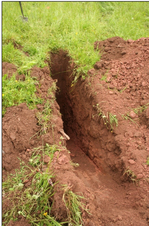
Photo 16: Post-hole T12 showing the depth of topsoil (1201) and pinkish-brown subsoil (1202) in section prior to the installation of the electricity pole (DAT Photo 4025-109382)
