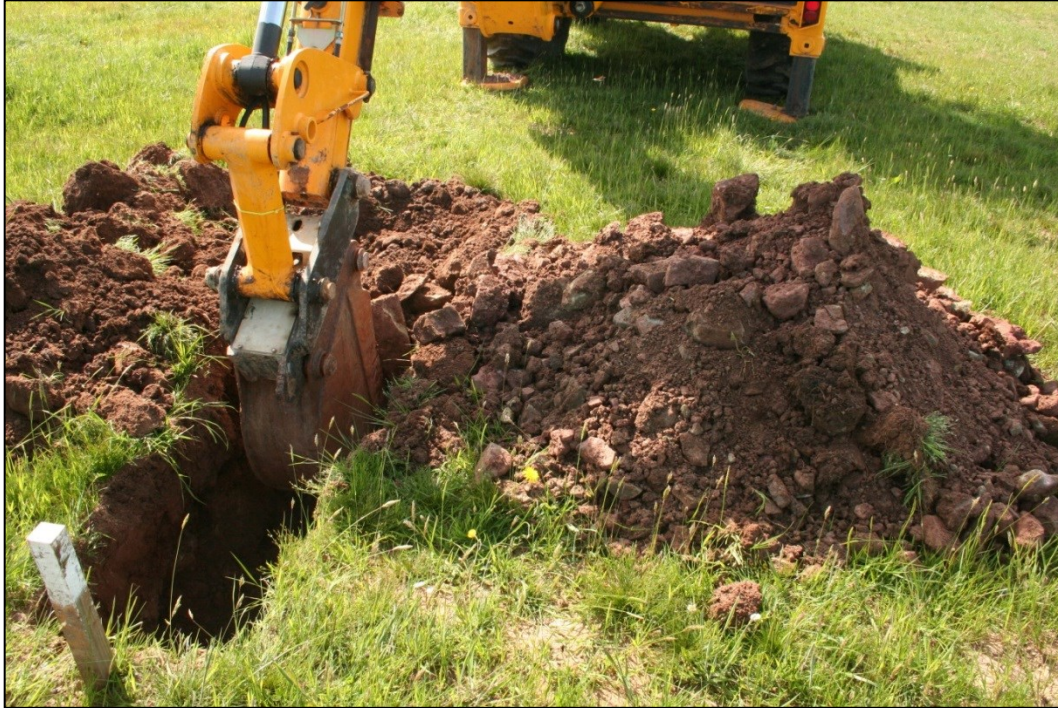
Photo 3: Excavation of T2 to receive the stay for T1's pole. Note the depth of topsoil (101) in the section and the nature of (102) mixed material being revealed. (DAT Photo 3955-109382).
