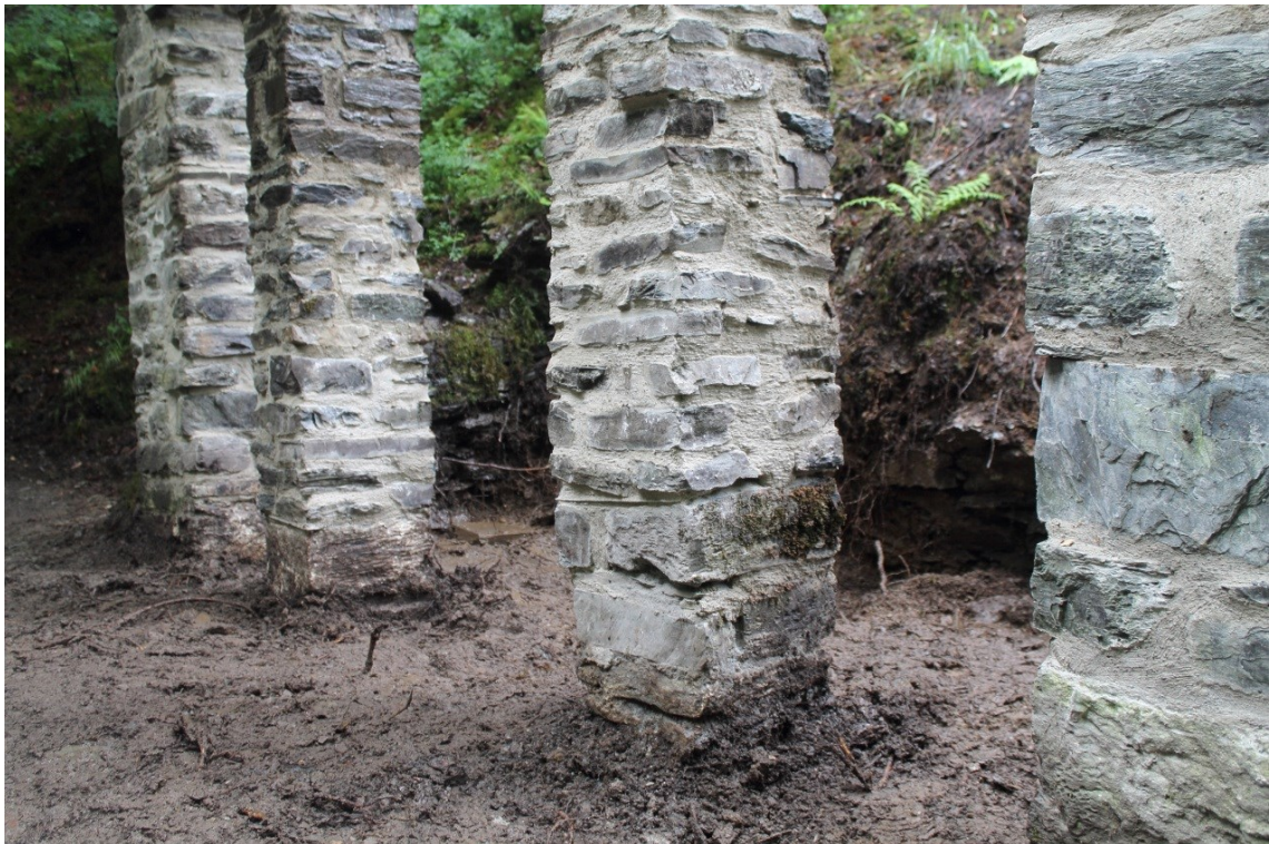
Photo 12: The cleared Gothic Arcade at the end of the excavation – looking south.
