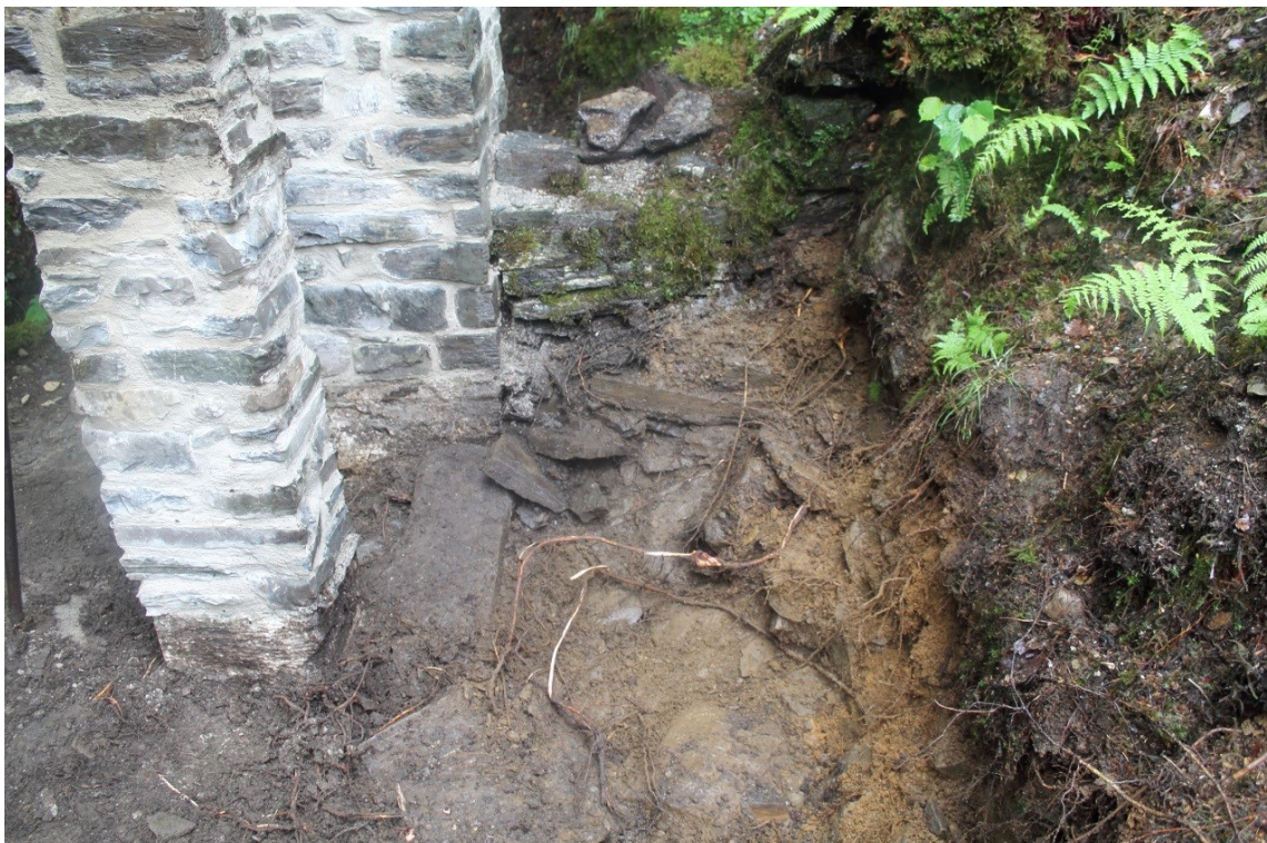
Photo 6: The southwest corner of the retaining wall during excavation of the stone rubble – looking roughly southeast.
