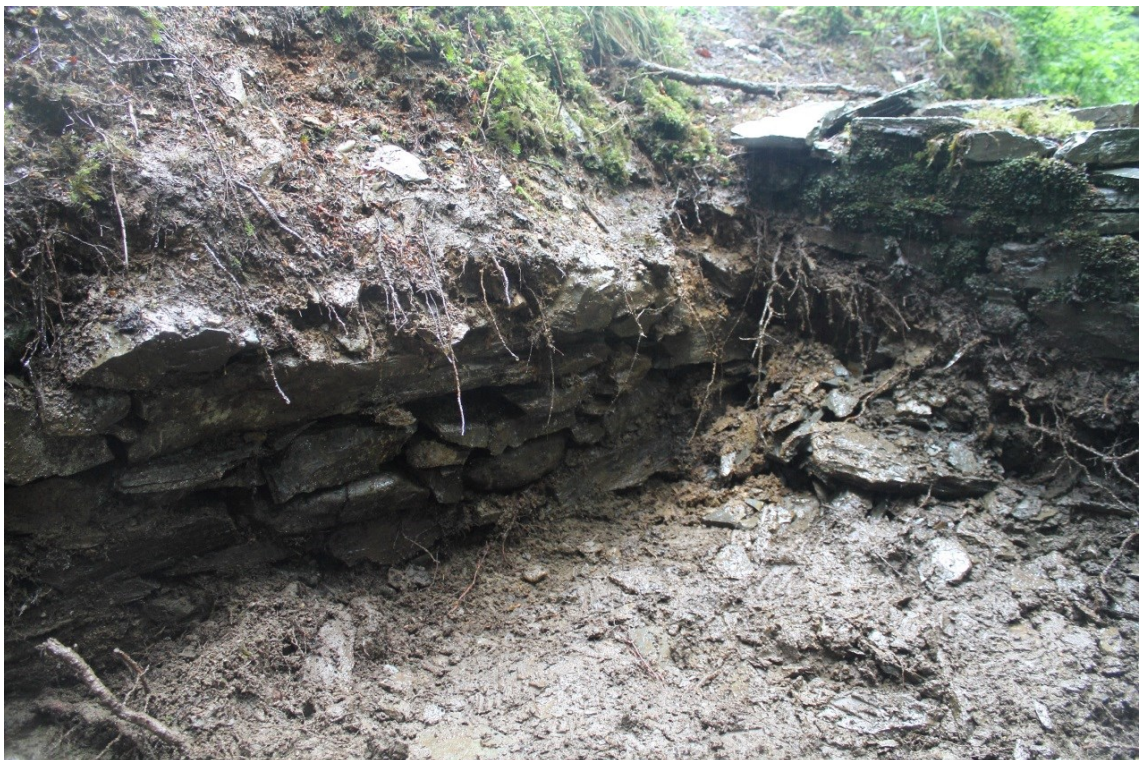
Photo 10: The northwest corner retaining wall at the end of the excavation showing the basic nature of the wall construction – looking roughly west
