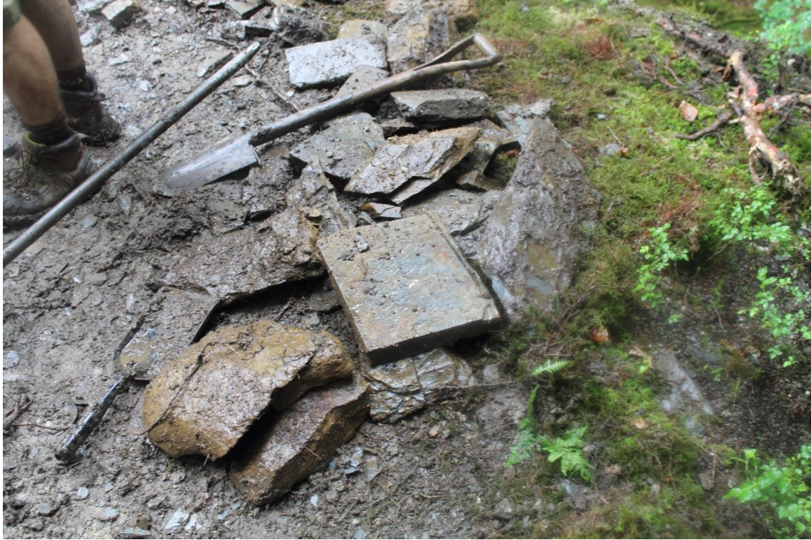
Photo 11: A selection of the roughly worked stone slabs used to construct the wall.
