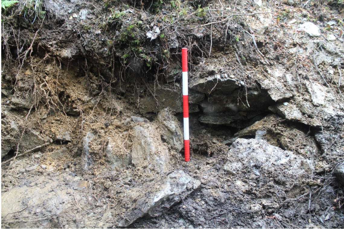
Photo 5: A remnant of the rear retaining wall emerging during excavation of the stone rubble – looking southwest. 0.5m scale
