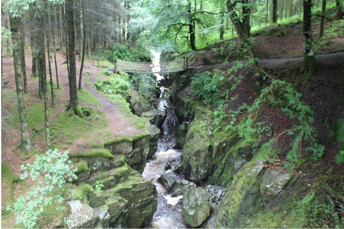
Photo 2: The view from the Gothic Arcade upstream towards the Chain Bridge (PRN 33025).
