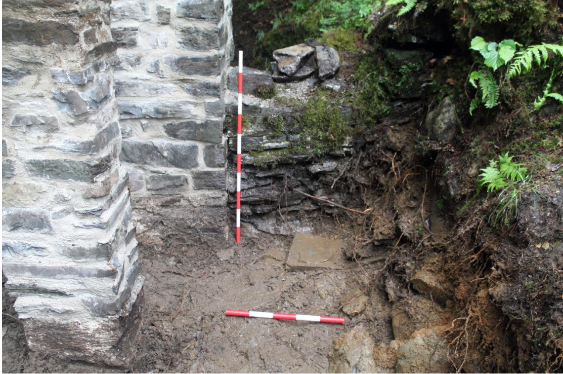
Photo 7: The southwest corner of the retaining wall at the end of the excavation of the stone rubble – looking roughly southeast. 1m & 0.5m scales
