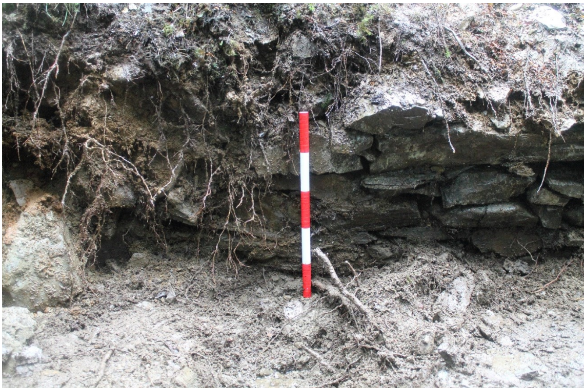
Photo 8: The surviving remnant of the rear retaining wall – looking southwest. 0.5m scale
