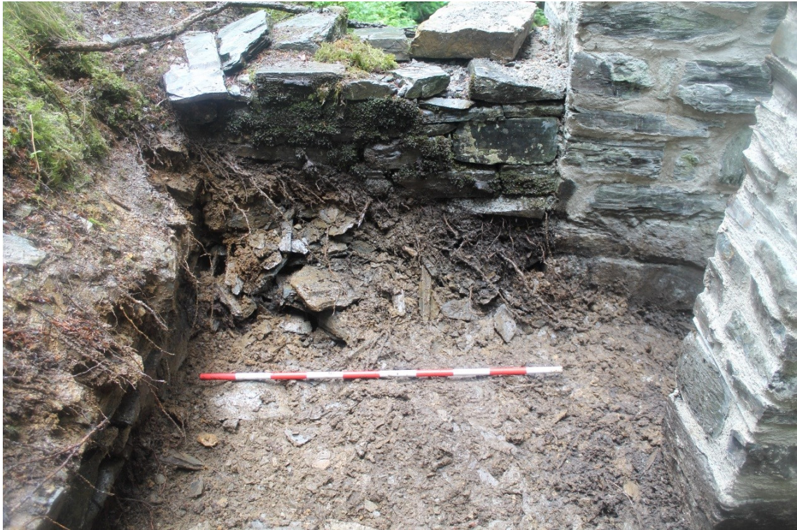
Photo 9: The northwest corner of the retaining wall at the end of the excavation – looking northwest. Note how the bottom section of the wall has collapsed inwards. 1m scale
