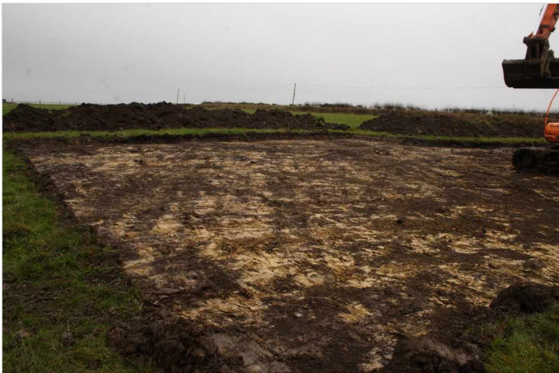
Photo 3: The stripped area of the turbine base showing the sterile clay-silt subsoil. (DAT Photo 109361-3725)
