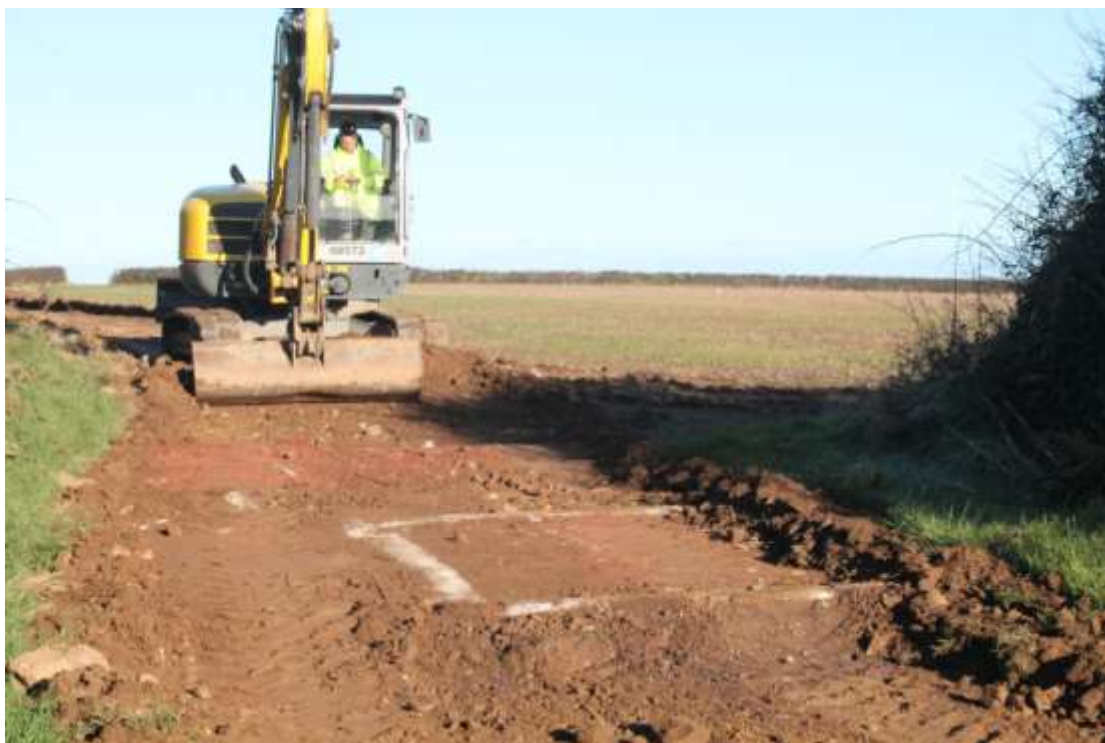
Photo 2: New track at point C, looking north, after excavation to final depth, showing patches of red stone and the rectangular outline left by a former breeze-block structure
