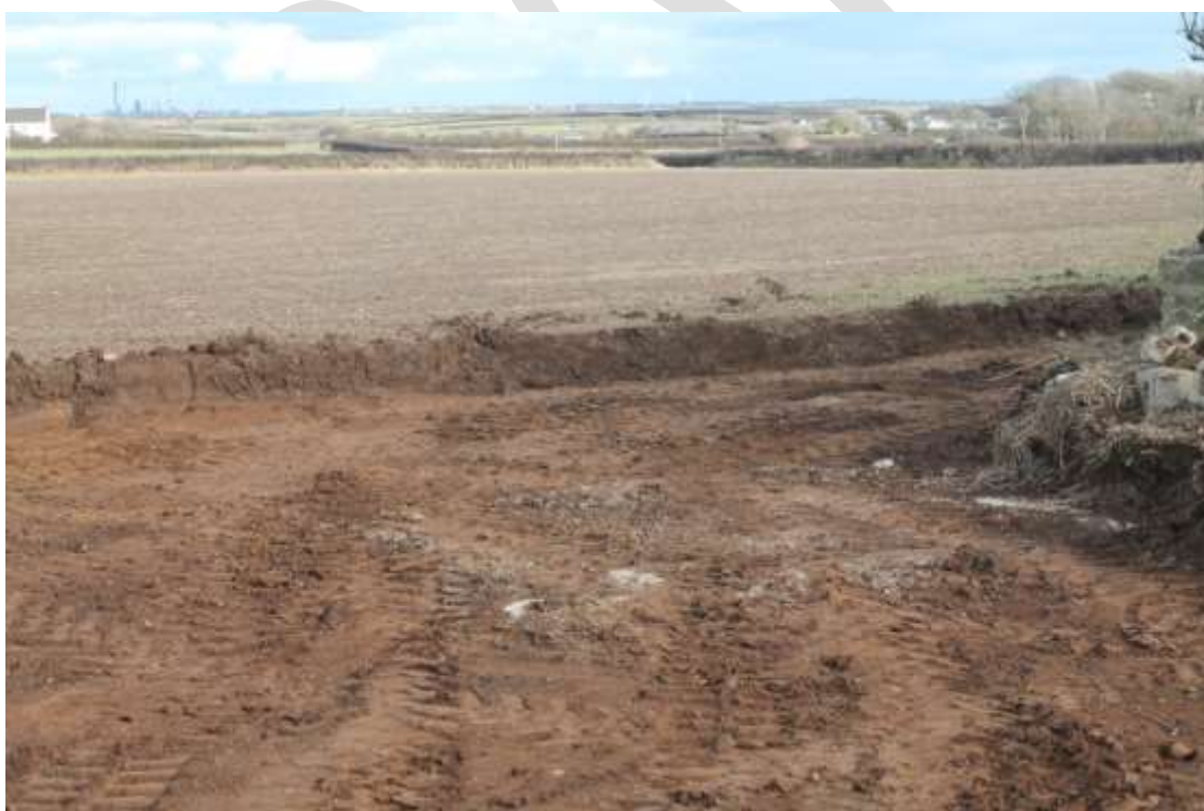
Photo 6: Looking east through the gateway at A, the breeze-block foundations of a former cattle grid after removal to the required depth for the track
