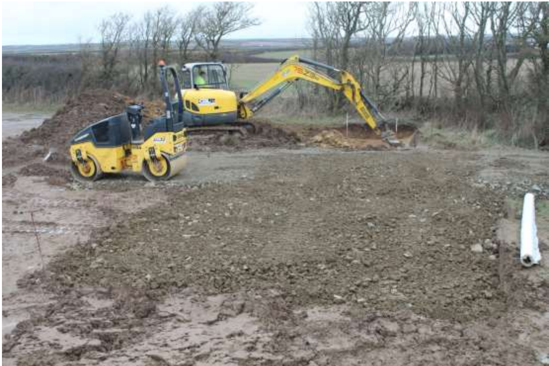
Photo 16: The completed turning place in area J in Figure 10, with the mast stand trench under excavation in the background.
