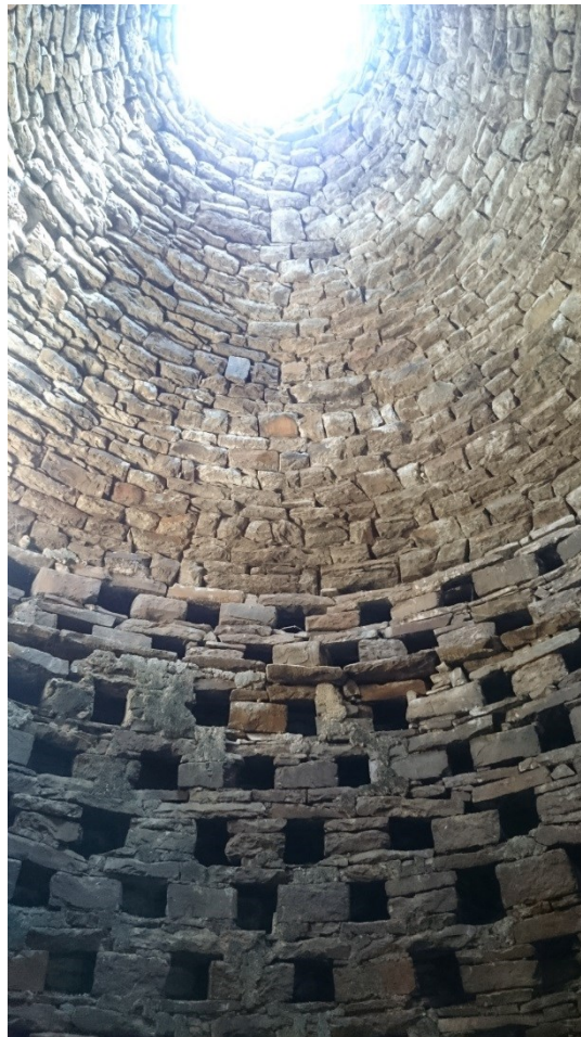
Photo 2: Internal view of dovecote, showing nesting holes in side walls, and domed, stone corbeled roof rising up to the central opening
