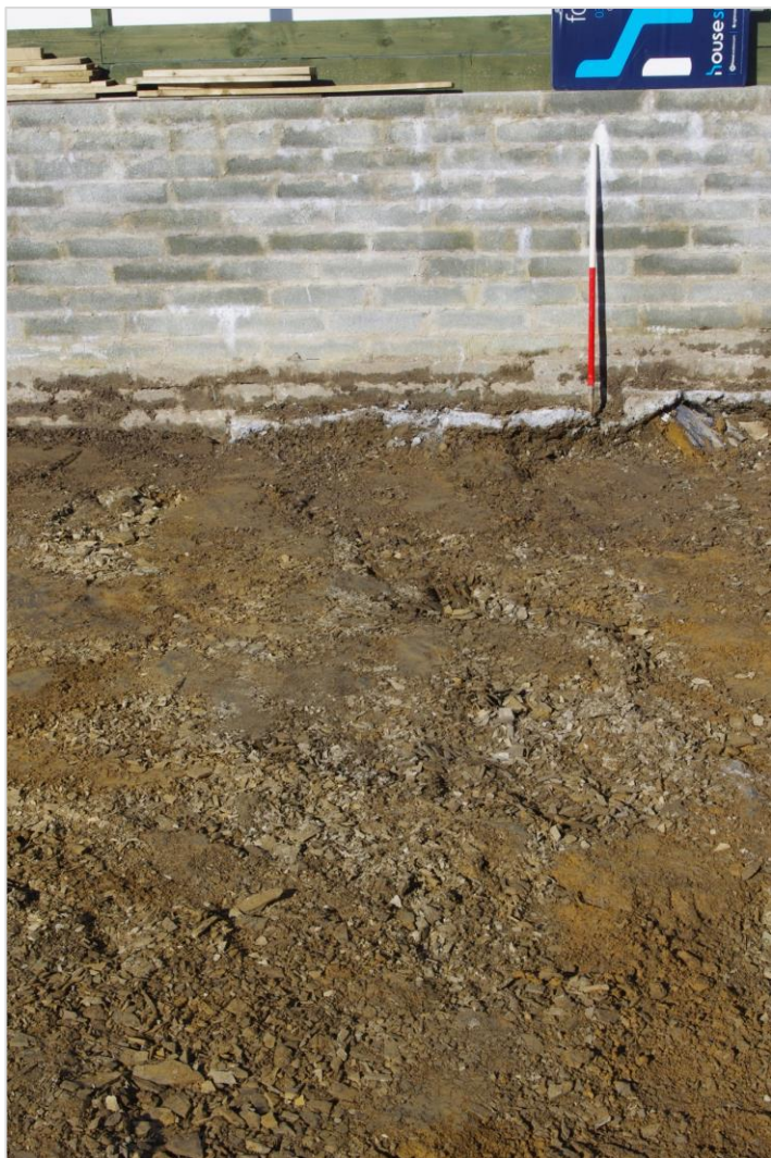
Photo 4: View west showing height of retaining wall to Coed Y Pia and outcropping shale bedrock at base of ground reduction works
