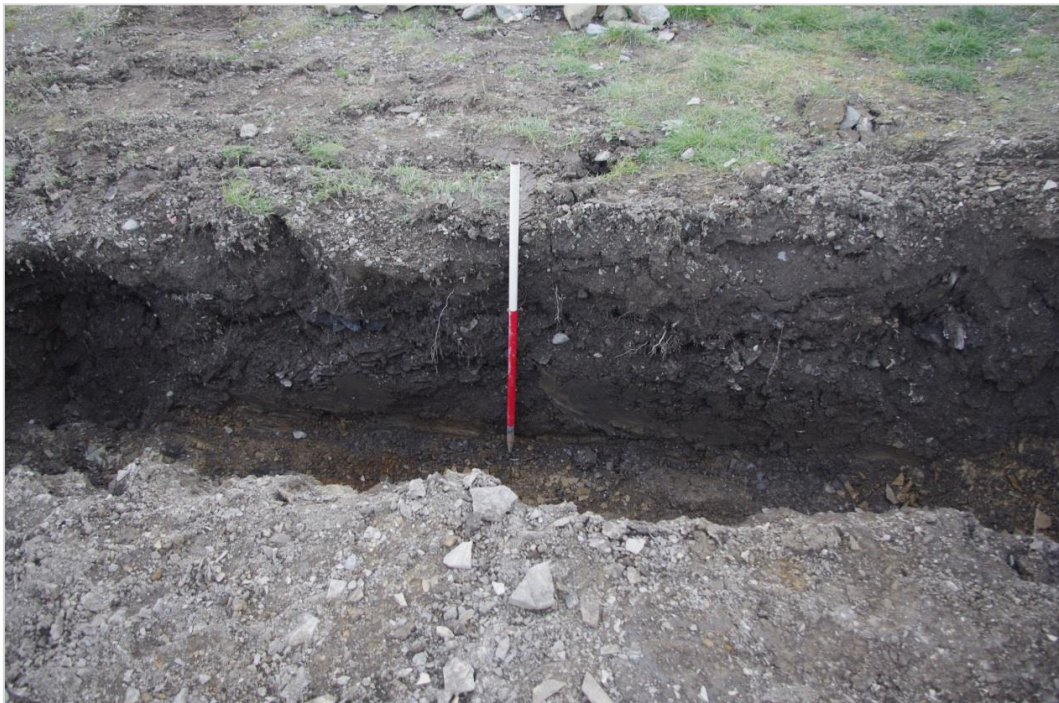
Photo 7: View south of the southern foundation trench for the new building cut through the darker soil area with bedrock exposed in base of trench
