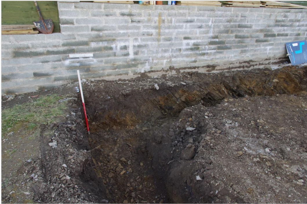
Photo 8: View west along southern end of the new building foundation showing the drop in bedrock level to the south
