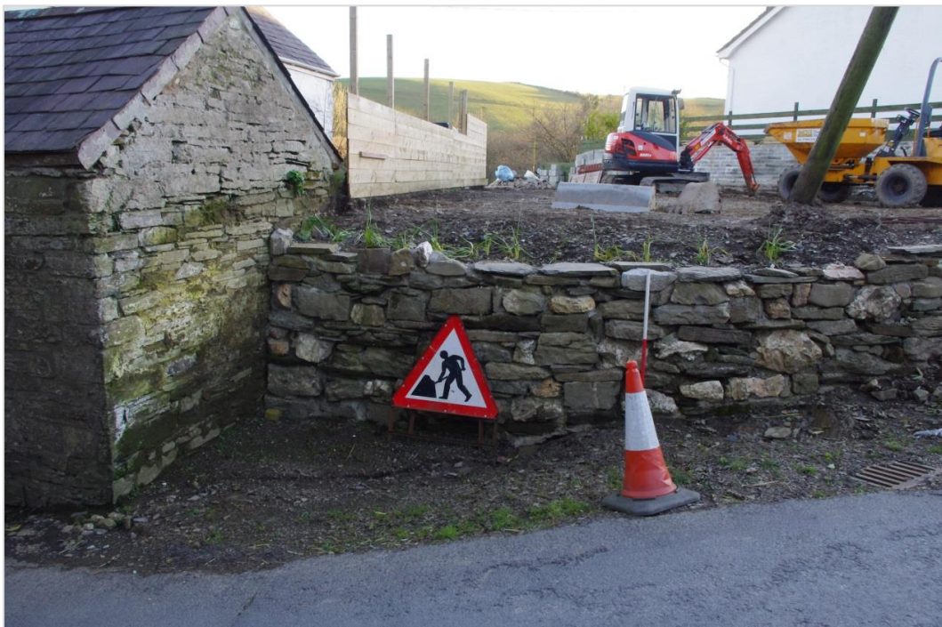
Photo 2: View south across the development site during ground reduction works showing the retaining wall on the Llanboidy Road frontage and ground levels
