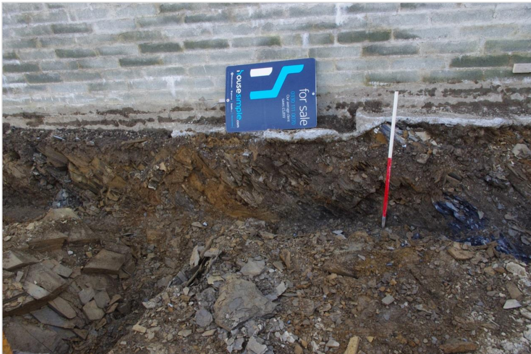
Photo 9: Bedrock exposed in western foundation trench adjacent to Coed Y Pia retaining wall, which sits directly upon the bedrock
