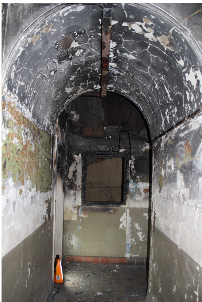
Photo 3: An example of the state of disrepair into which the building has fallen: smoke damage, cracked and peeling wall coverings in a corridor between offices at the west end of the building
