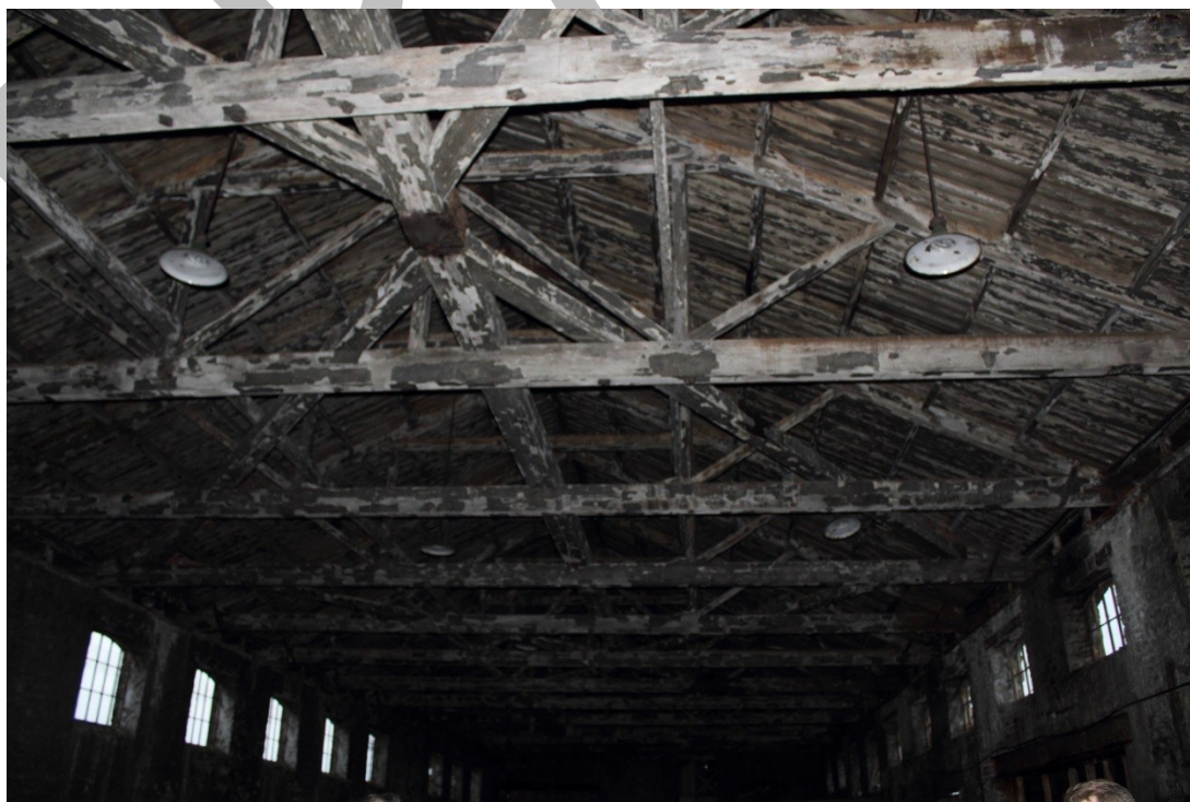
Photo 2: The interior of the goods shed itself, in poor superficial condition, but showing the complexity of the timber work in the surviving roof
