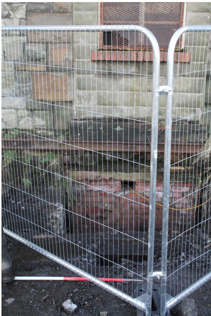
Photo 9: Recent investigation has revealed a bricked-up entrance way below ground level in the north wall of the goods shed. One of the re-used rail tracks that covered this pit can be seen in situ. 1m scale.
