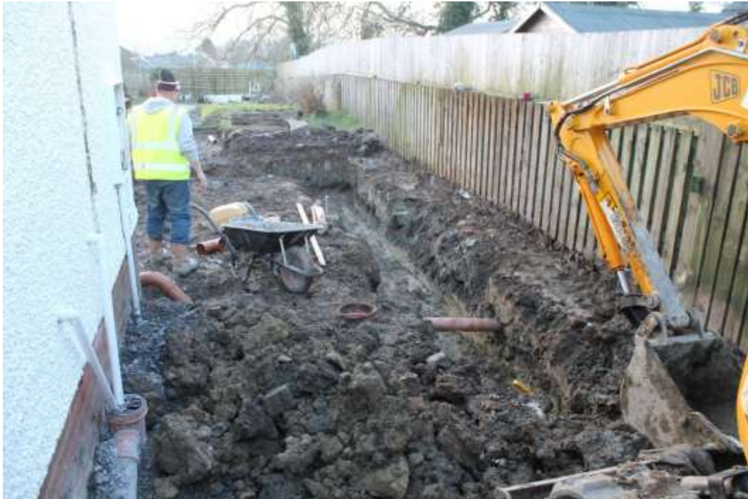
Photo 8: View southwest along northwestern foundation trench, showing clay base to the trench with mixed material above and modern drain and other services
