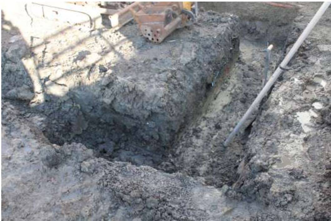
Photo 9: general view of excavation of foundations showing full depth of trench exposing clean grey/brown clays along base and mixed material above
