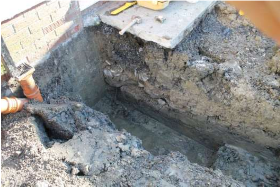
Photo 6: Foundation trench adjacent to 3 Clos Llwyn Ty Gwyn, showing existing foundations of house and adjacent rain water drainage
