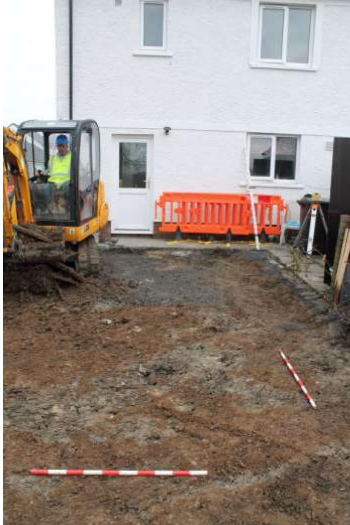
Photo 5: View northeast across stripped site towards 3 Clos Llwyn Ty Gwyn showing the mixed nature of exposed soil and rectangular area of stone sub-base for former patio
