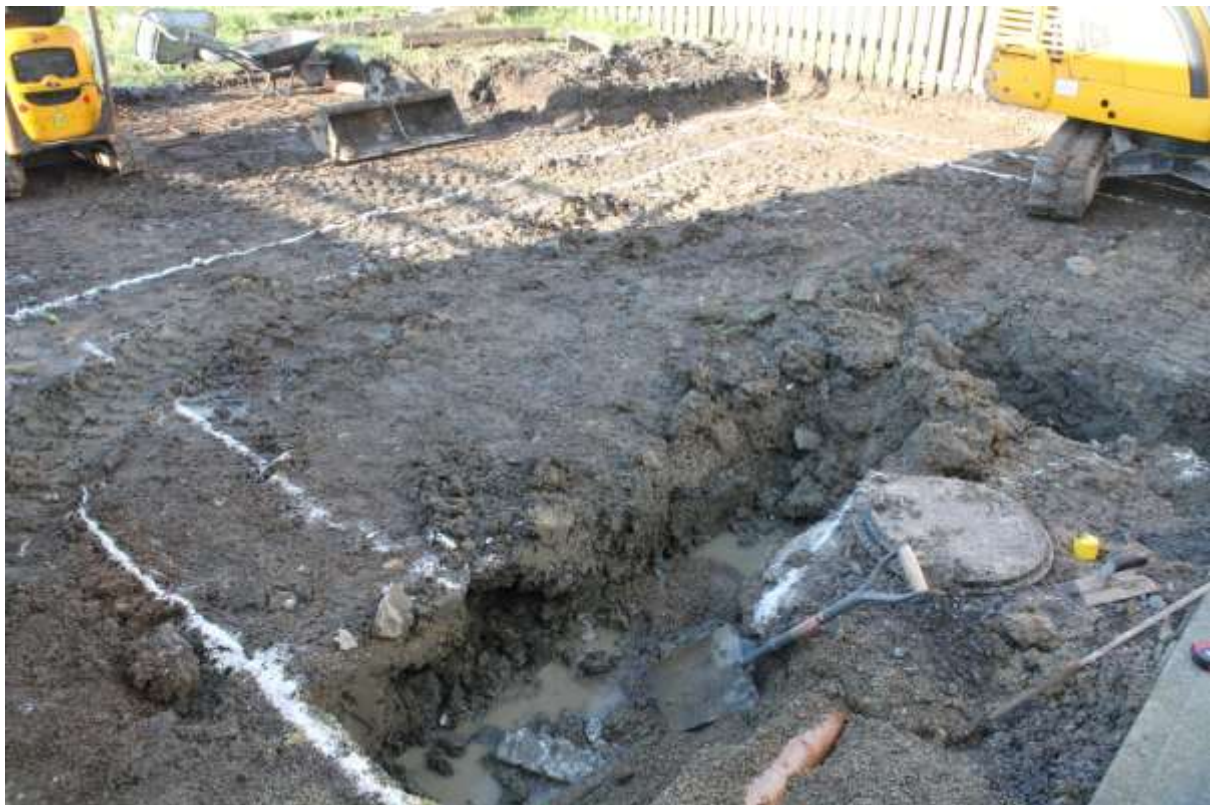
Photo 7: View northwest across extension area showing sewer manhole close to property with pipe trench and gravel backfill along edge of foundation trench
