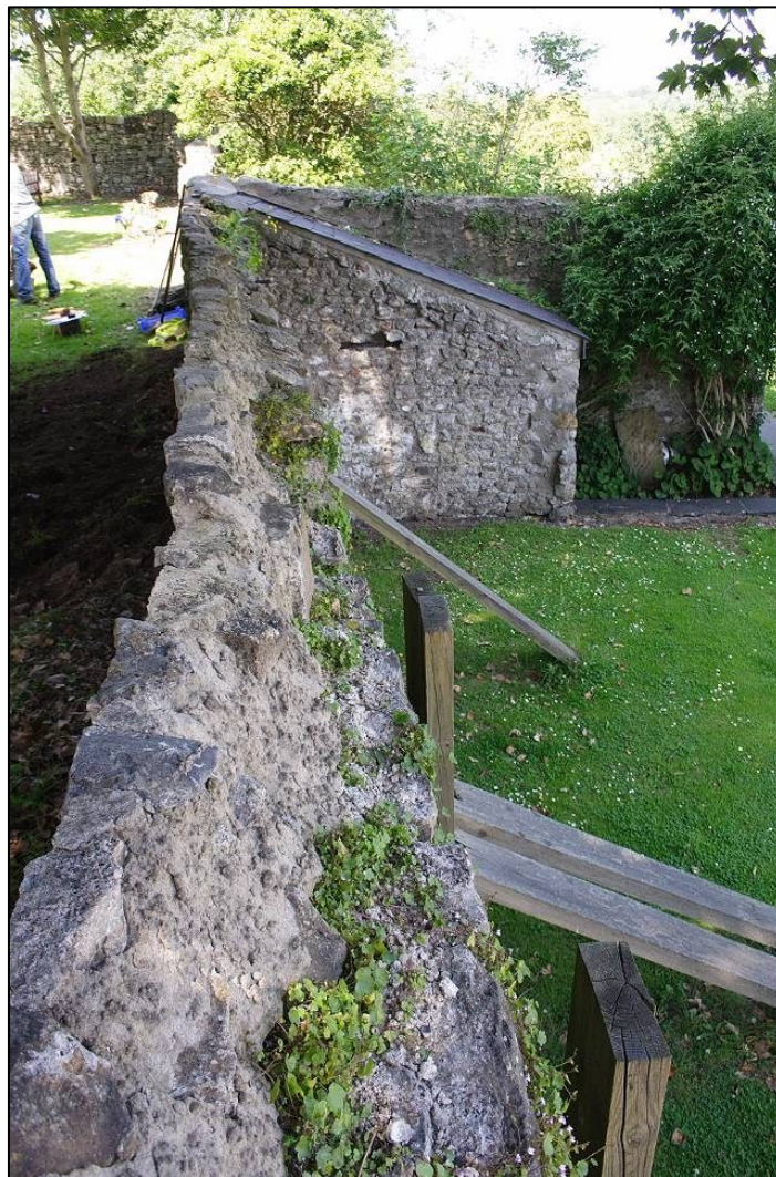
Photo 3: The bulging eastern boundary wall (06) prior to works. Note the temporary shoring. (DAT Photo from 2011).
