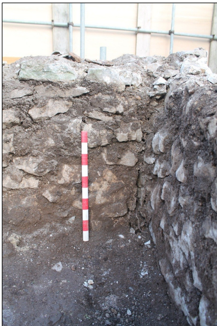
Photo 6: The butt joint of walls (06) (orientated E-W) and (07) (orientated N-S) seen prior to dismantling. (DAT Photo IMG_5734-108990)
