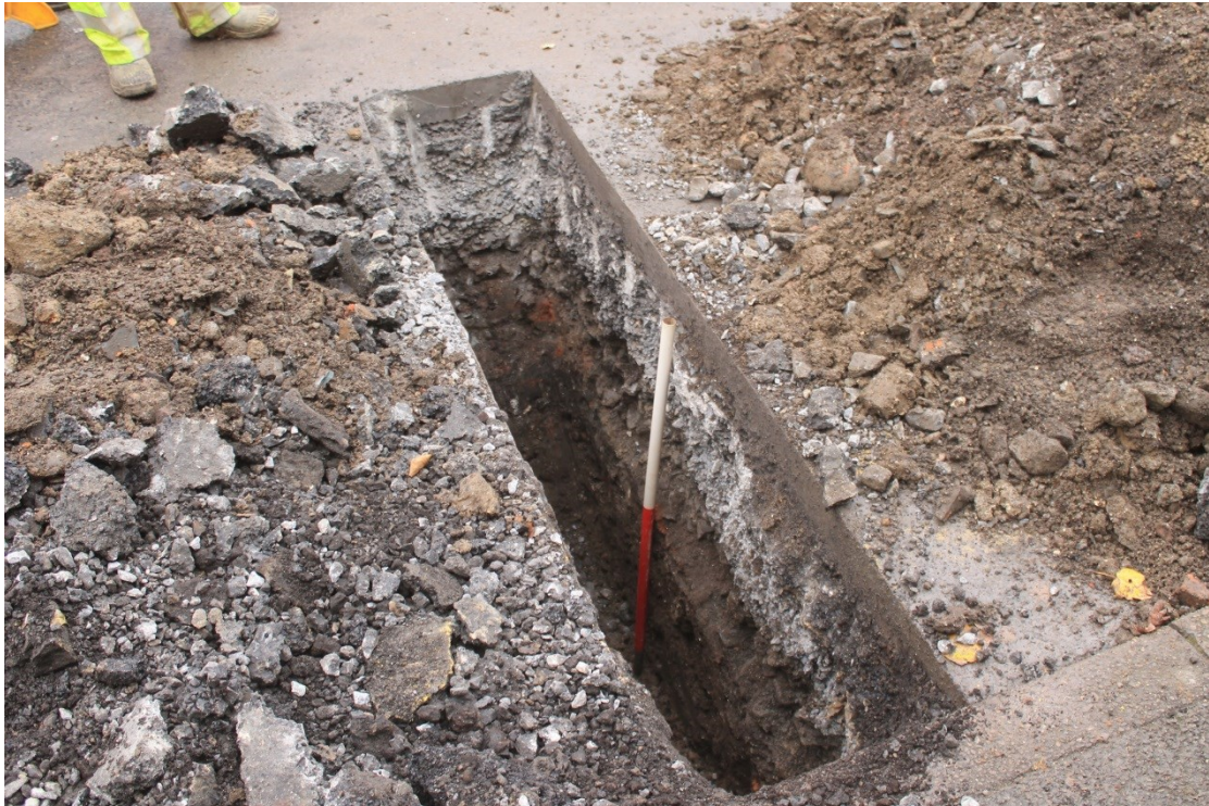
Photo 9: Trial hole T6 after excavation was completed showing the very dark, compacted mixed deposit that lay below hard core and tarmac. Looking approximately northwest. 1m scale
