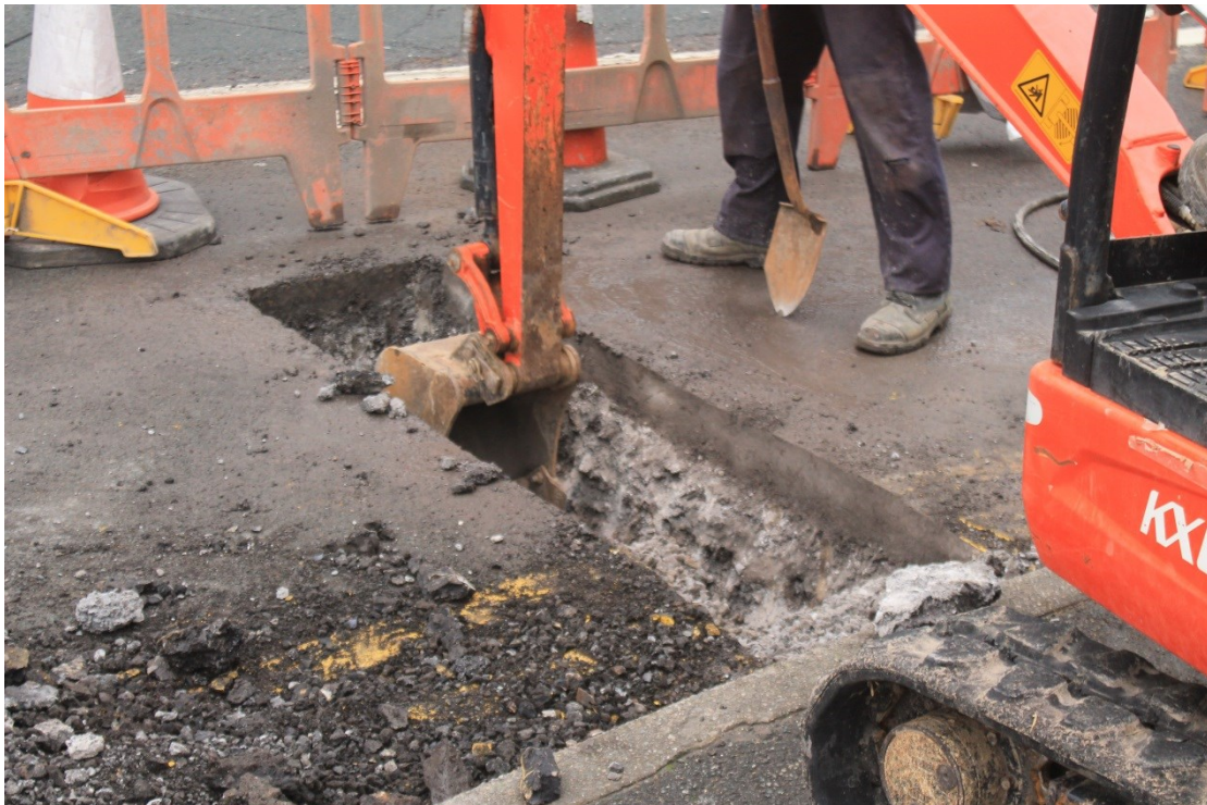
Photo 2: Excavation of trial hole T4. The tarmac and hardcore measured approximately 0.65m deep.
