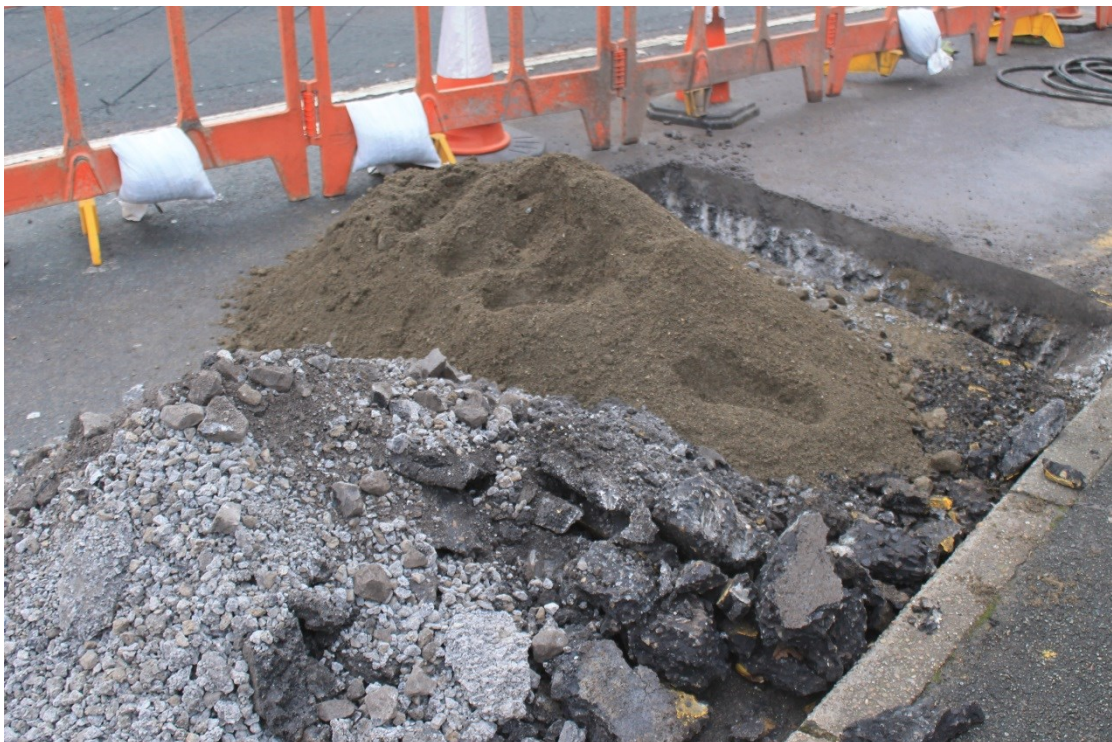
Photo 4: The spoil heap by the side of T4 showing the very clean, distinct natural sand and gravel excavated from the trial hole.
