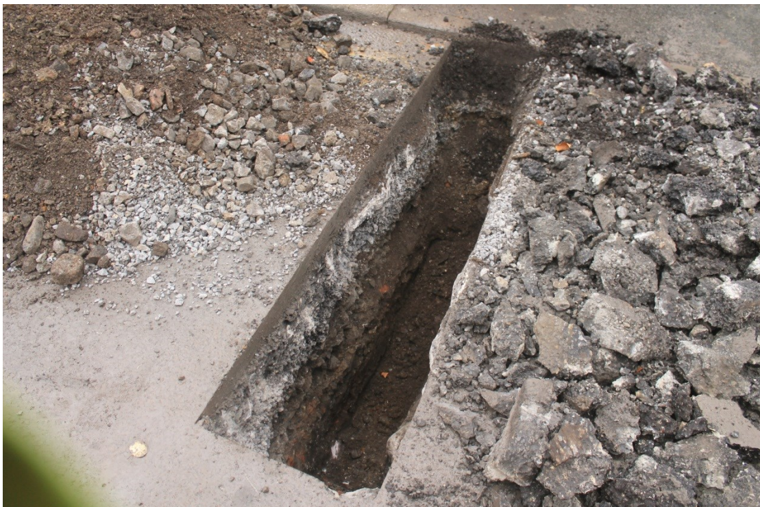
Photo 8: Trial hole T6 after excavation was completed showing the very dark, compacted mixed deposit that lay below hard core and tarmac. Looking southeast
