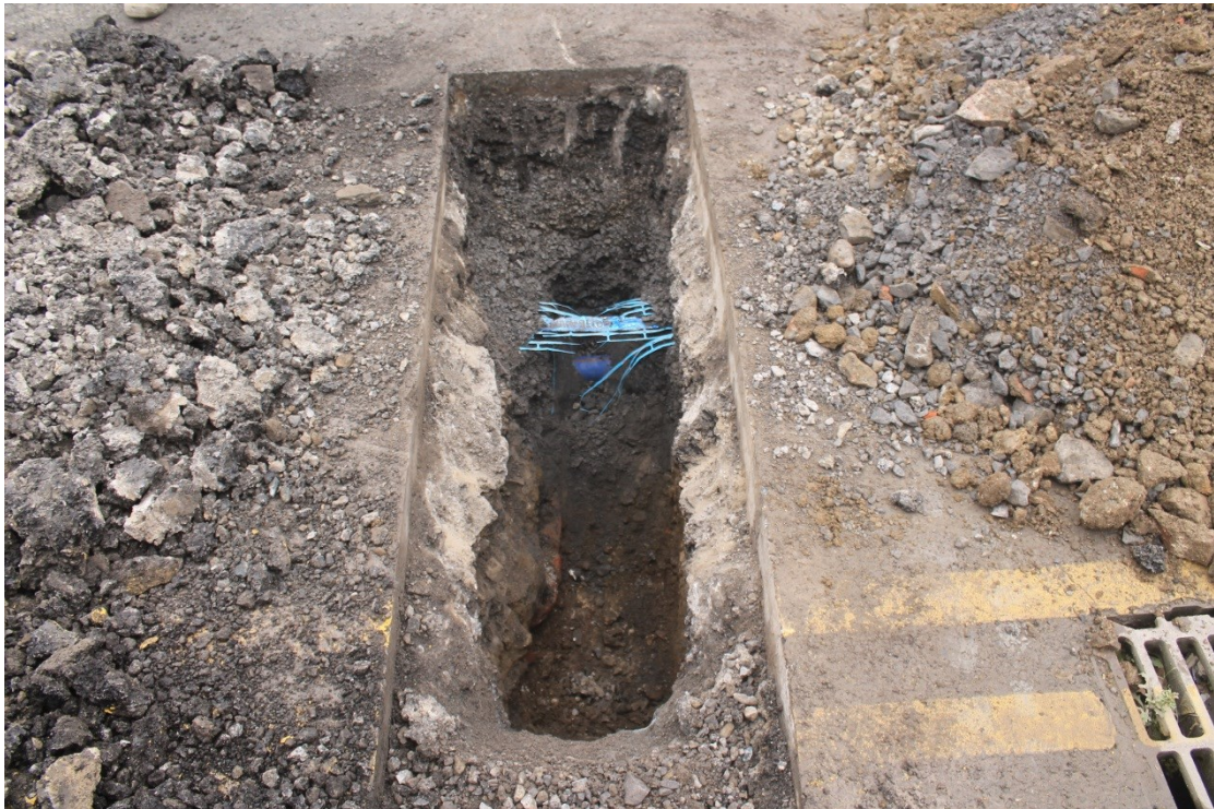
Photo 6: Trial hole T5 after excavation was completed showing what appears to be substantial brick footings at approximately 1.0m depth. A modern water pipe can be seen in the northern end of the trench. Looking north.
