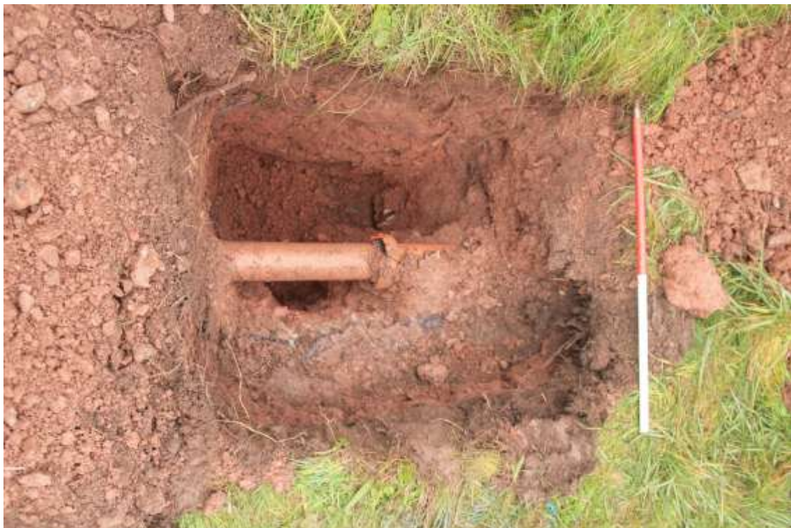
Photo 3: East view of TH10 with BT ceramic conduit and remains of former tarmacadam road surface. 1m scale
