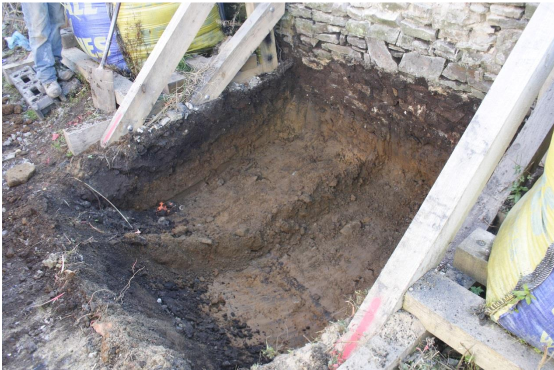
Photo 2: Mid-excavation shot of Buttress 2, showing clearly the relationship of the base of the wall and the encountered deposits.
