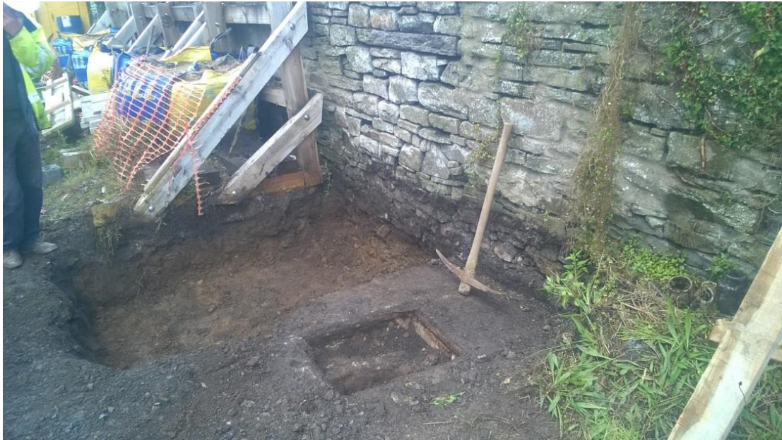
Photo 1: Excavation of Buttress 1. Note the exposed manhole in the foreground.
