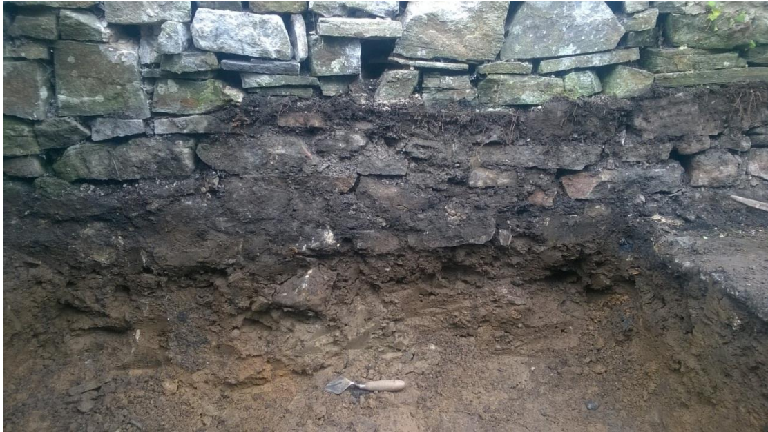
Photo 5: Detailed view of the base of the churchyard wall within area of Buttress 1 showing lack of any foundations, indicating it was built on or close to the original ground level
