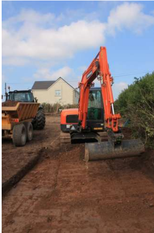
Photo 5: Stripping the area of the driveway for the southeastern house plot, showing the exposed natural geology, viewing northwest
