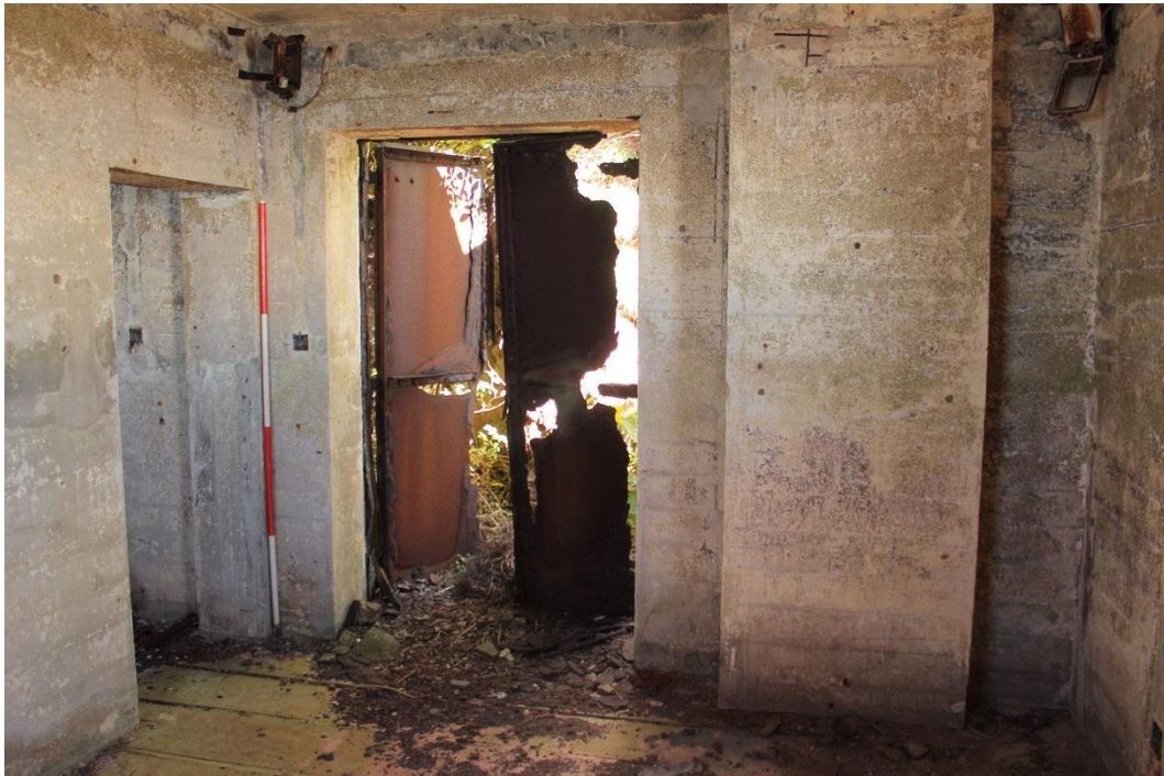
Photo 82: Interior of Transmitter / Receiver Building PE493A, showing badly corroded iron doors on northeastern side
