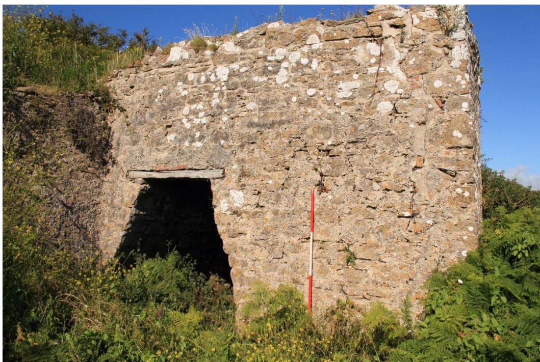
Photo 49: West facing wall of limekiln showing very dry lintel in need of replacement.
