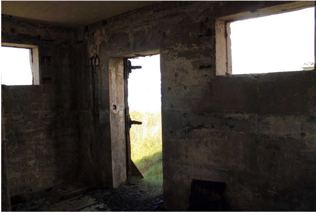
Photo 83: Interior of Transmitter / Receiver Building PE493A, showing almost totally corroded iron doors on northwestern end
