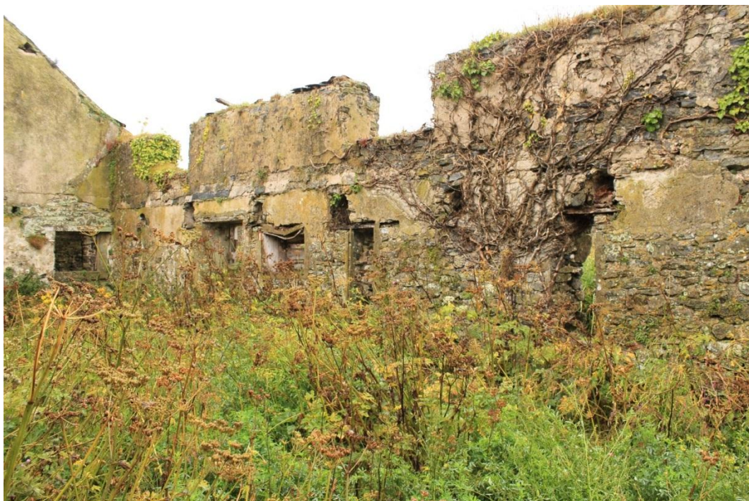
Photo 26: East facing wall of northeastern range, showing damage to internal wall by vegetation.
