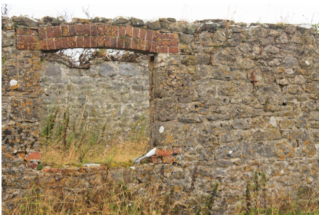
Photo 38: View east of window opening in cowshed showing mortar shell within window opening
