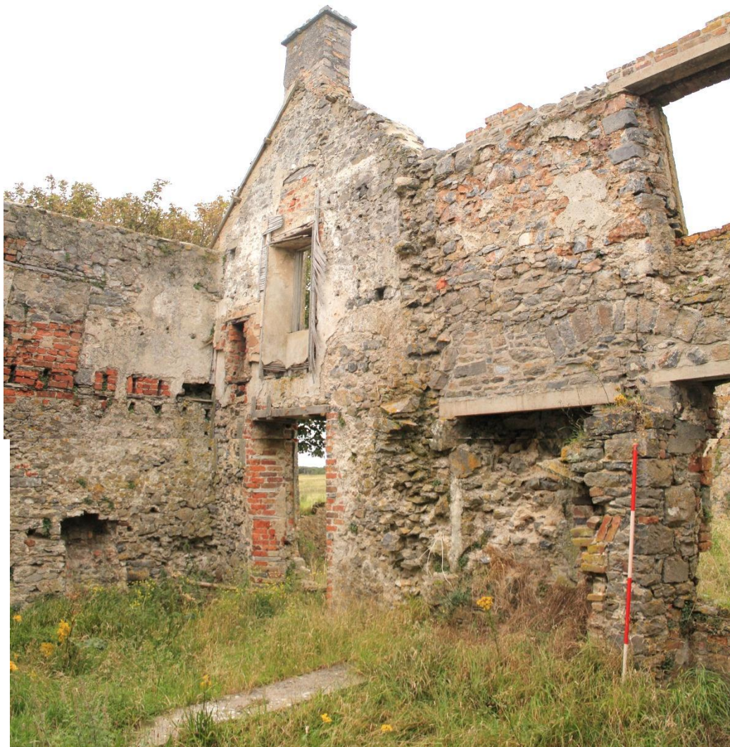
Photo 42: View northeast within northern room of Flimston farmhouse, showing concrete lintel repairs within building
