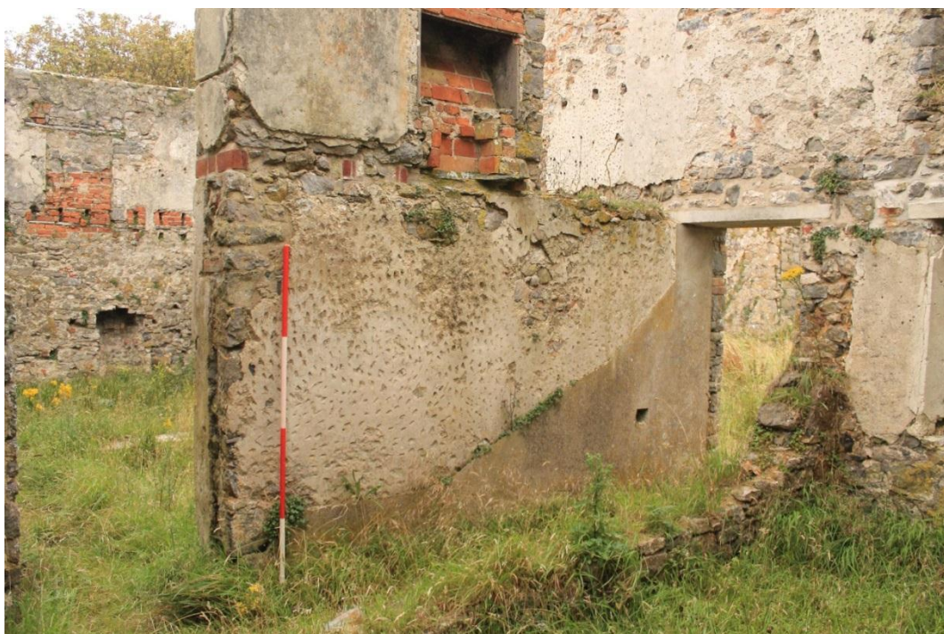
Photo 43: Internal wall showing some plaster damage.
