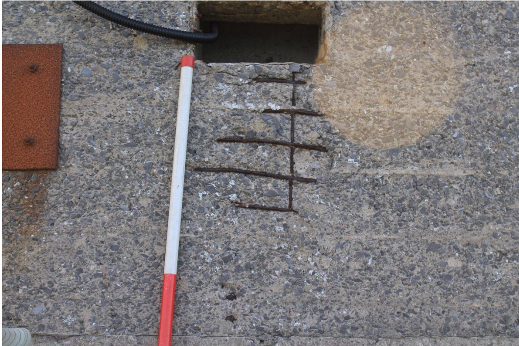
Photo 81: Area of blown concrete on northwestern wall of PE493C showing exposed reinforcing bars underneath
