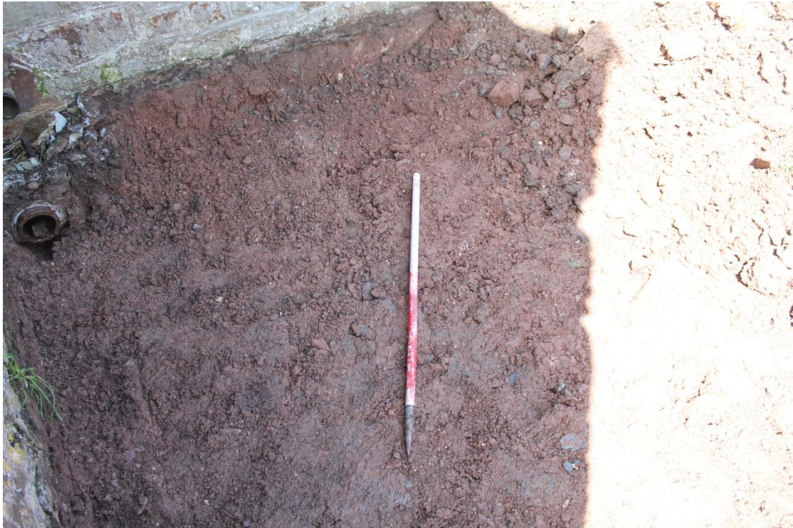
Photo 2: Reduced ground level within the footprint of the new toilet extension showing made-ground material
