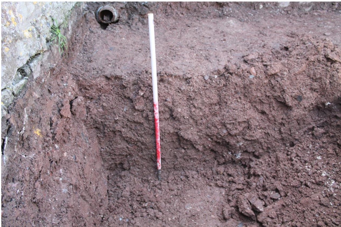
Photo 3: East facing section of footing trench. The trench was excavated to a depth of approx. 0.60m and appears to consist of the same made ground with grit and crushed brick
