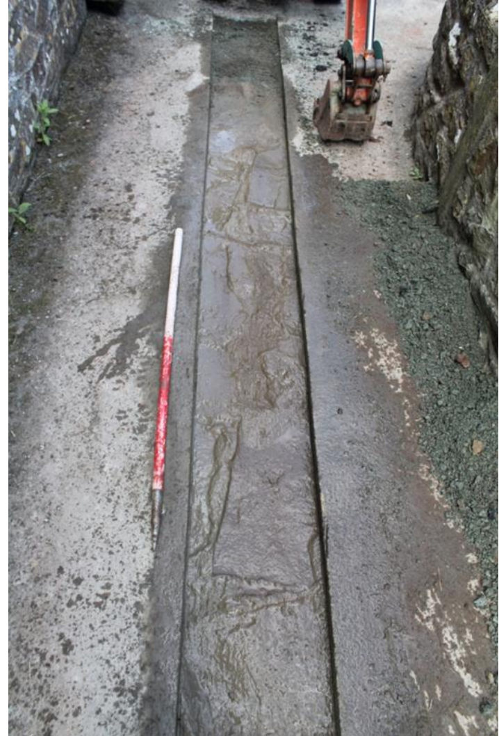
Photo 5: Removal of the existing tarmac path revealed the former stone paved path beneath. Viewing West along the north wall of the north transept.
