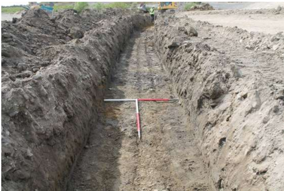
Photo 58: Several wide bands of loosely compacted medium and large pieces of rock were seen running diagonally across the excavated drainage channel (3). Looking northwest. 2 x 1m scales.
