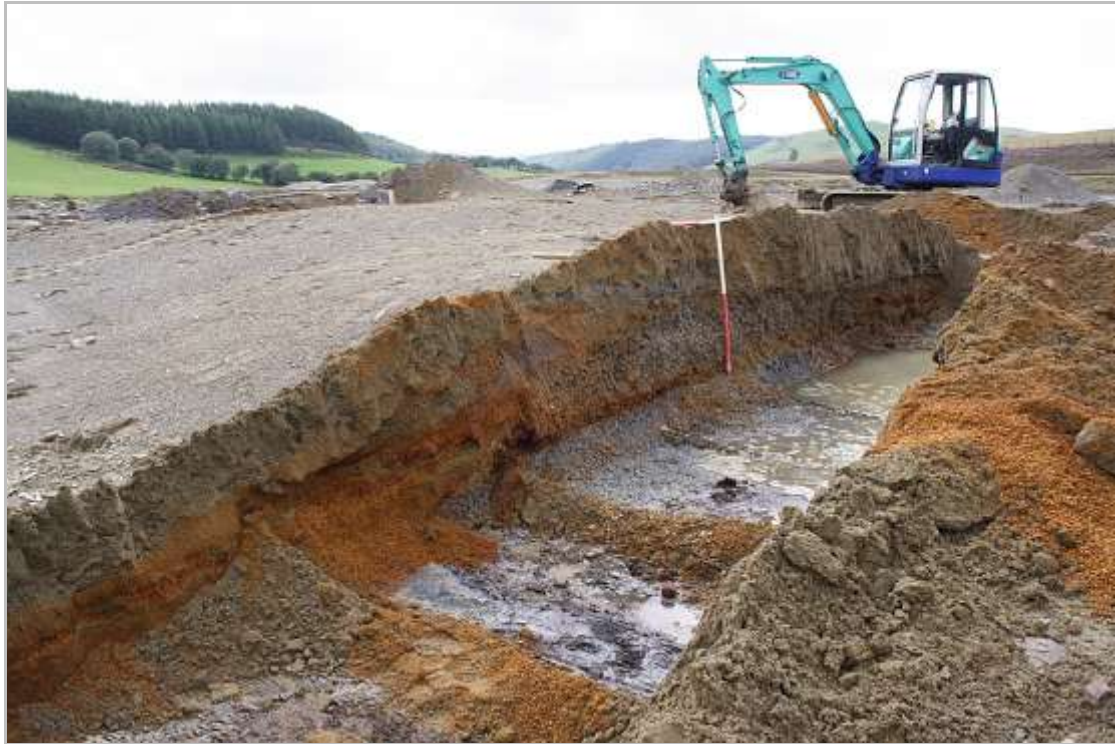
Photo 4: One of a number of trenches excavated during the archaeological evaluation in 2012, showing the deep deposits of mine waste that cover the former dressing floors.
