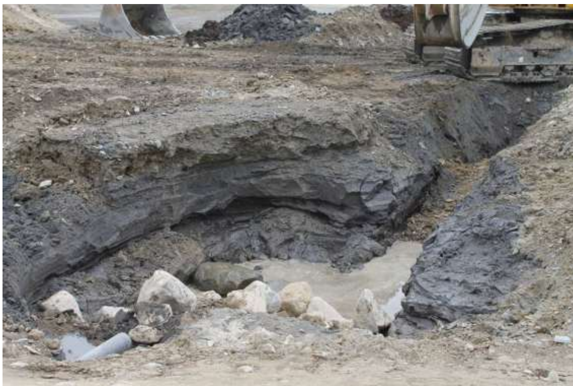
Photo 56: In the exposed sections of the pit, excavated as a sump, could be seen thick layers of dark grey silt that doubtless represent the alluvial deposits that built up within the former mine reservoir. Looking northeast.
