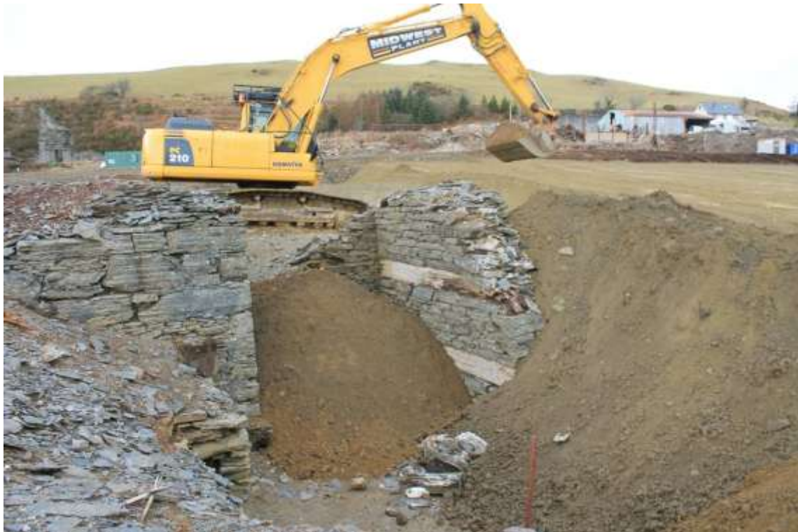
Photo 46: Backfilling the internal area of the Crushing and Stamp Mill with large deposits of mine waste. Looking north.
