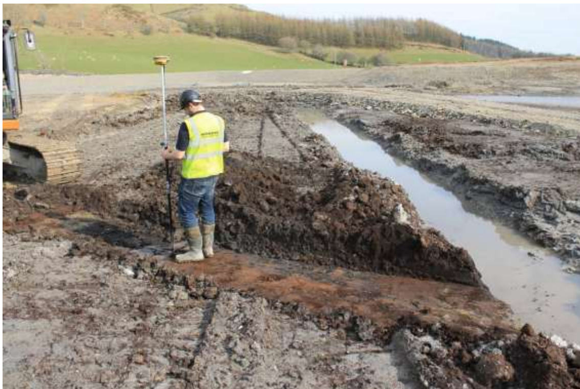
Photo 52: The initial excavation of drainage channel (2). Looking southeast.
