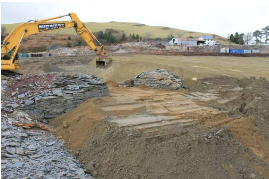
Photo 47: The tops of the Crushing and Stamp Mill walls were left exposed so the position of the mill would still be visible. Looking north.
