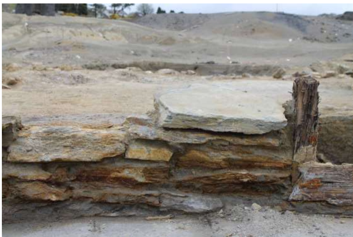
Photo 14: A section of the outer stone wall of buddle (A1) showing its construction. On the right of the picture is the wooden sluice (A4). Looking north.
