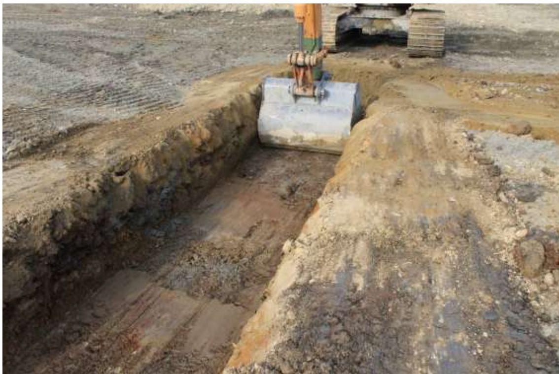
Photo 54: The mixed deposits of mine waste revealed during the excavation of drainage channel (2). Looking north.
