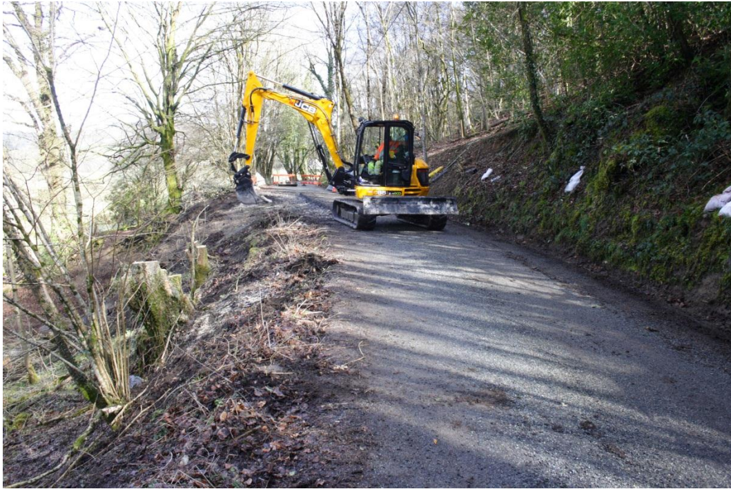
Photo 9: View northwest along the Brunant Highway repair area showing the significant terrace into the slope of the existing road line
