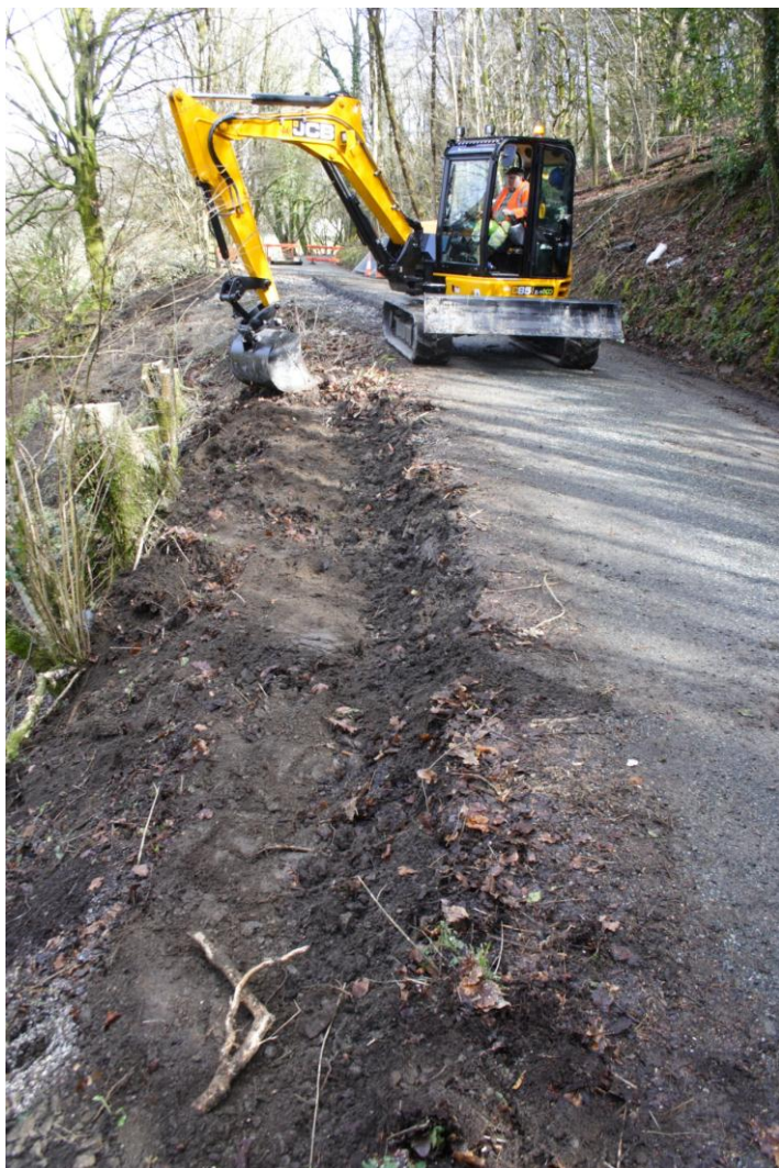
Photo 2: Cleaning the road edge to the southwest of the road repair area
