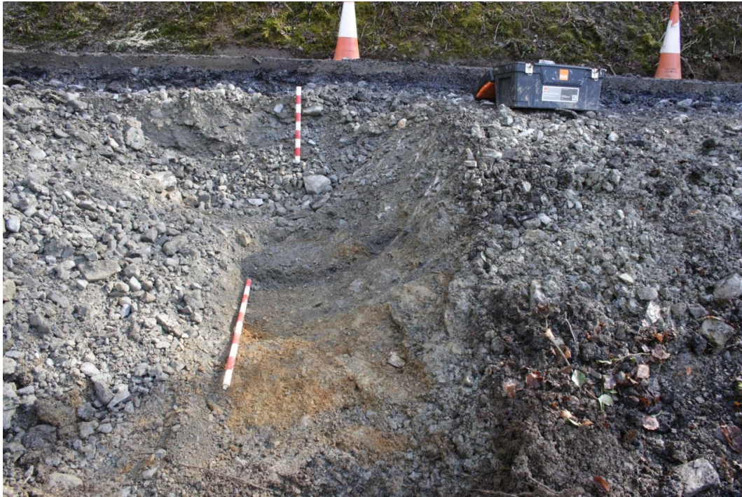
Photo 7: Test slot at northeastern end of scheme showing cut edge of tarmac, road make-up and bedrock beneath viewing southeast (1m and 0.5m scales)
