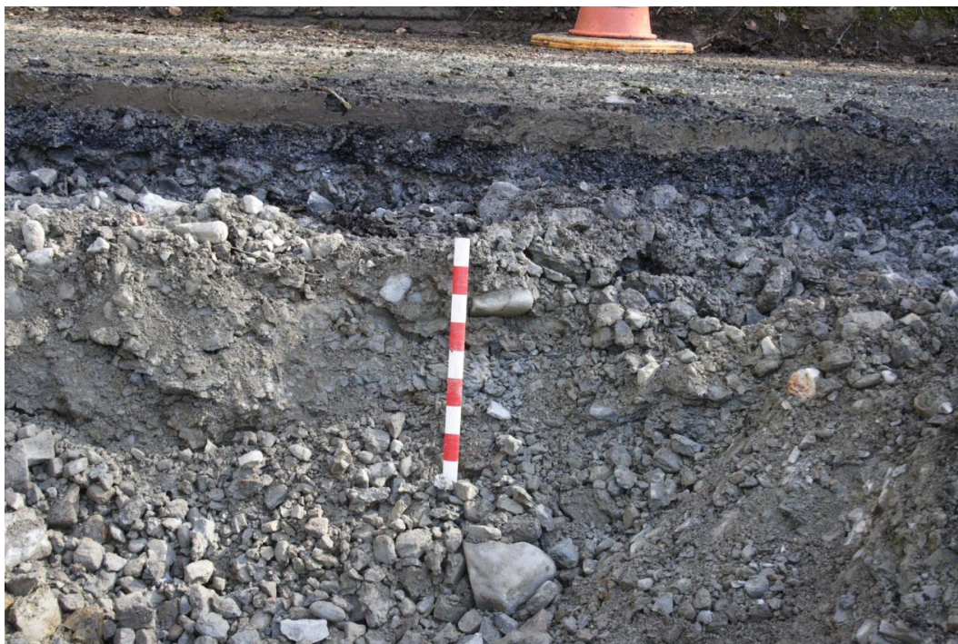
Photo 4: Representative northwest facing section through road make-up deposits within the 15m length of the Brunant Highway Support Scheme area (0.5m scale bar placed in front of bedrock)
