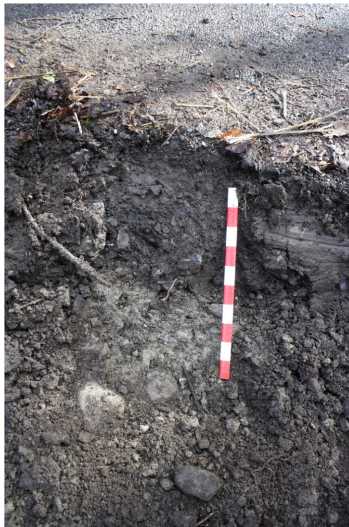
Photo 3: Small section cleaned up against existing road edge showing make-up layers
